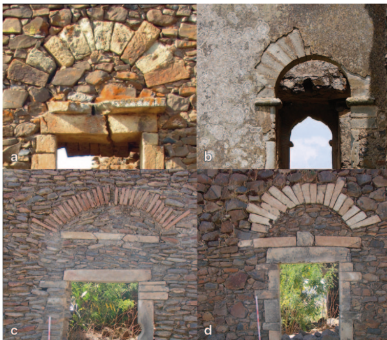
Fig. 7.3 The arches over windows and doors at the Jesuit residences of Gorgora Nova (a), and Däbsan (c–d; c with an arch made of bricks), and at the royal palace of Dänqāz (b). (Photographed by author)
