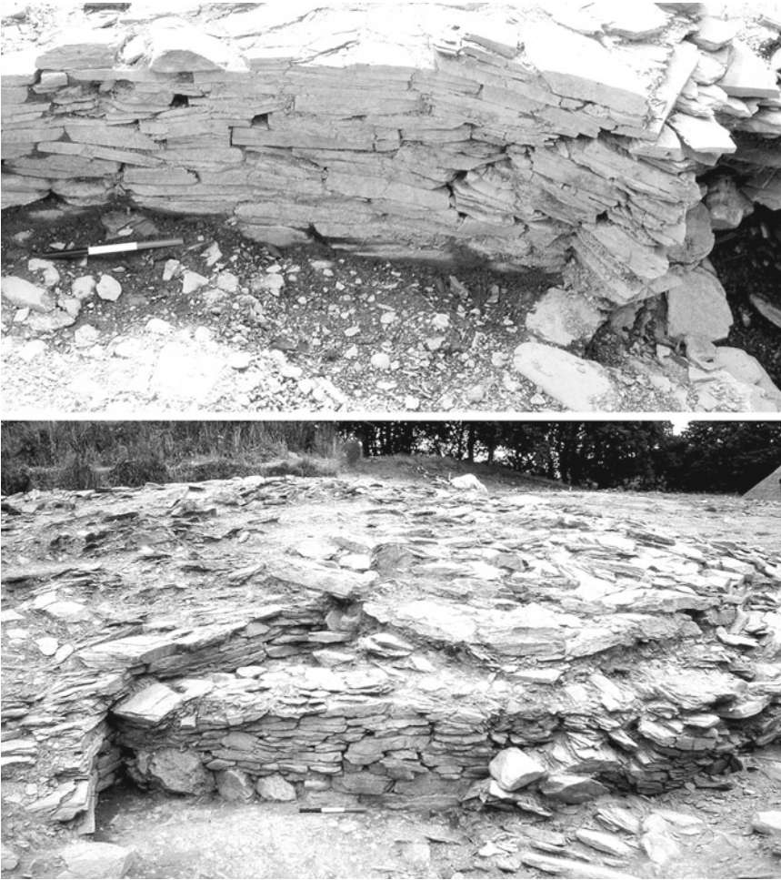
Fig. 12.14 Top: walling 2754 of western Period 3 guard chamber I. Bottom: eastern outer convex walling 3402, butting up against the interior of Period 2 guard chamber II wall 3401. Note the unstable and repaired part of this wall to the right, towards the gate itself, with rough walling 3403
