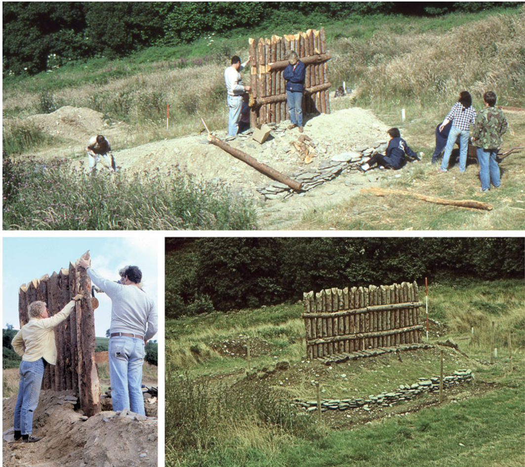
Fig. 10.8 Experimental earthwork. Top : Under construction in 1986 with the rampart built but not fully compacted, rear revetment wall in place, scarp being completed and palisade being put in place. Bottom left : Placing the palisade in its construction trench, more fill was to be added at the front. Bottom right : With animal-proof fence in 1989; note turfs on the front, grass from seeds on the rear; the base of the scarp cut (visible on the left ) has not yet regenerated vegetation naturally
