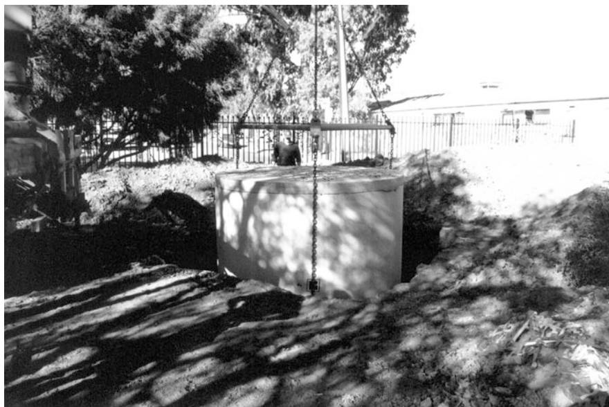
Fig. 12.3 Installation of concrete rainwater tank at St. Mary's Cemetery in Adelaide to accommodate human skeletal remains (photo T. Anson)
