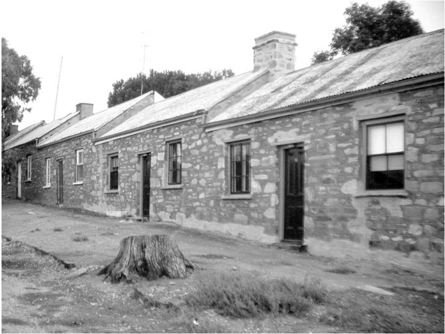
Fig. 9.4 Houses in Burra in South Australia, built in the traditional stone manner and lacking verandahs (photo S. Lawrence)
