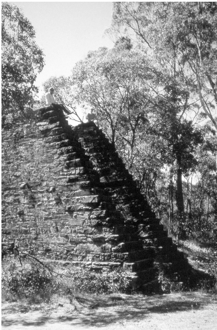
Fig. 7.5 Garfield Water Wheel near Castlemaine in Victoria, used to drive a large stamp battery in the 1880s (photo S. Lawrence)
