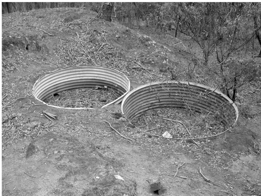
Fig. 7.6 Cyanide vats for separating gold from finely crushed ore at Steiglitz in Victoria (photo P. Davies)
