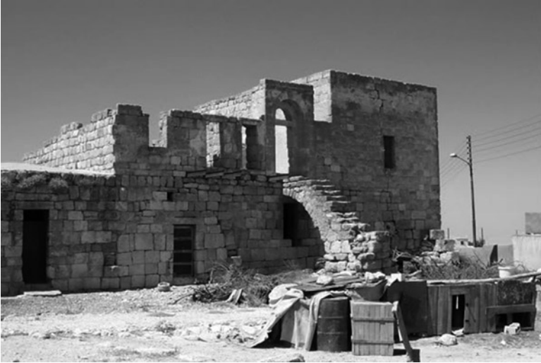
Fig. 5.3 The nineteenth-century farmhouse structure ( Beyt Nabulsi ) at Hisban. Domestic space, including a guesthouse, is located above storage rooms. (Courtesy of the author)
