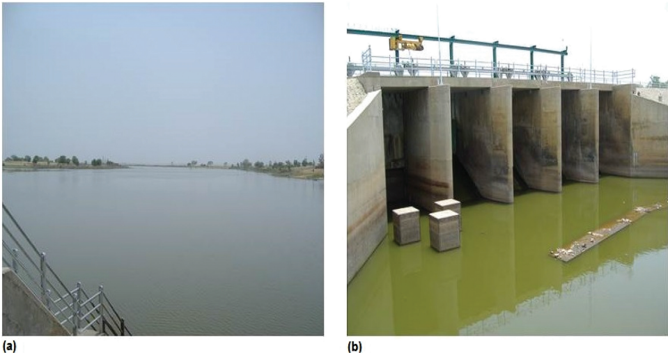
Figure 4.3(a and b) Lake Alau dam reservoir and the dam outlet.
