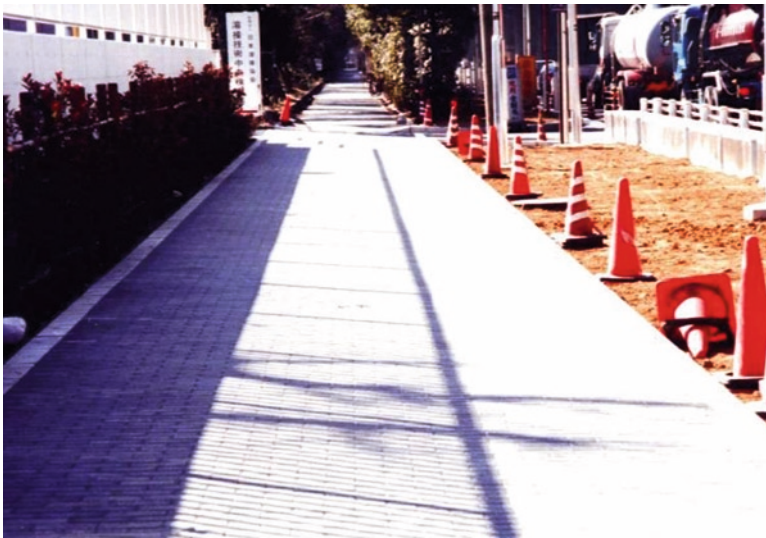
Fig. 5.8 Concrete blocks pavement in Kawasaki City, Japan in 1999
