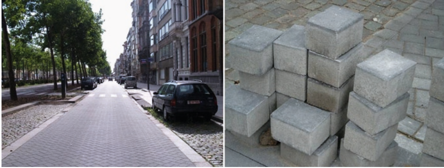
Fig. 5.11 Separate parking lanes at the Leien of Antwerp with photocatalytic pavement blocks
