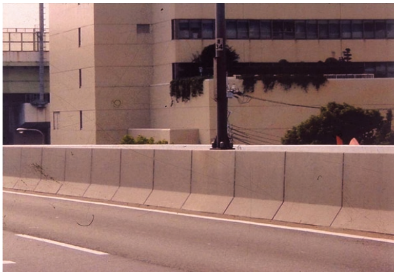
Fig. 5.15 Drainage pavement and railing wall coated with photocatalytic polyacrylic ester-modified pastes in an expressway (Courtesy of Taiheiyo Cement Corporation)
