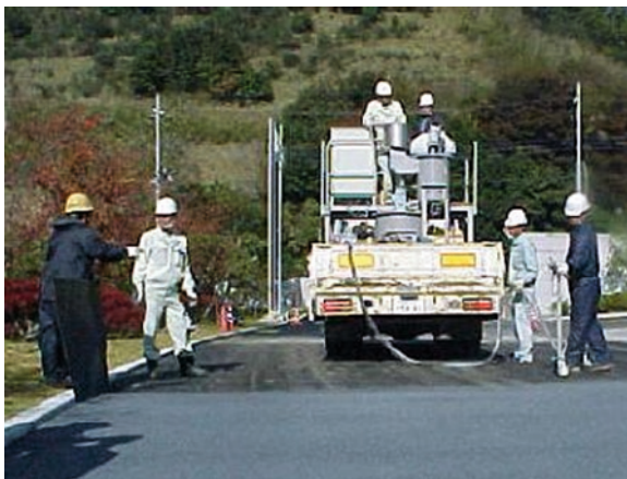
Fig. 5.14 Coating equipment with a mixer and spray applicator for polymer-modified pastes or slurries on a truck (Courtesy of Taiheiyo Cement Corporation)
