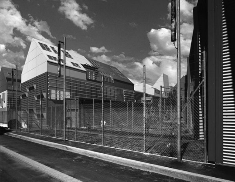
Fig. 7.6 Adam Towle, Open House Alliance, MArch Design Studio project 2009. Using the principles of Open Source Software, the project intends to halt the trend of standard, generic houses that lack individualised architectural input, yet also proposes to place key design decisions in the hands of the user and not the architect. [Copyright: Adam Towle and The University of Sheffield]
