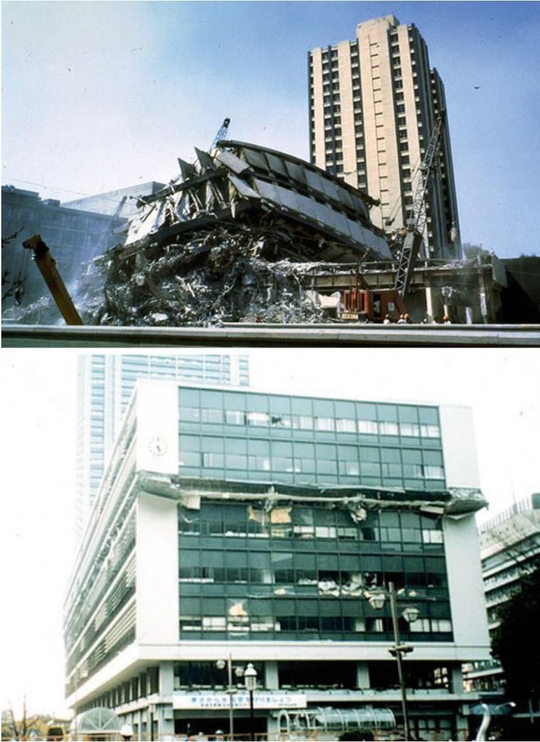
**Fig. 4.16** *Top* Collapse of the 21-storey Pino Suarez building on top of an adjacent 14-storey building after the Mexico earthquake of 1985 (Credit: EERI); *bottom* the mid-storey collapse of the SRC building (it is the old Kobe Town Hall in Chuo-ku) due to brittle weld connections after the Kobe earthquake in 1995. (Source Charles Scawthorn)
