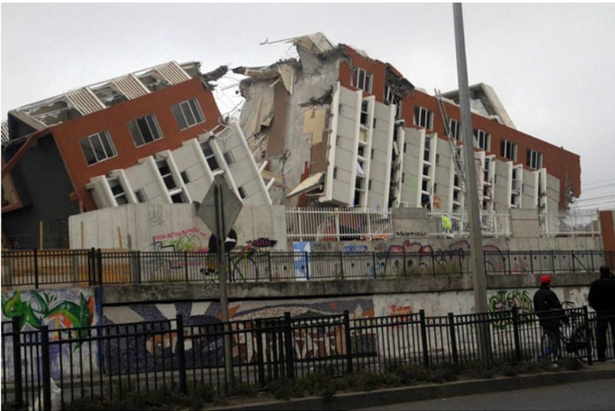
**Fig. 2.18** The collapse of the Alto Rio building in the 2010 Concepción, Chile earthquake (Credit: Wikipedia)
