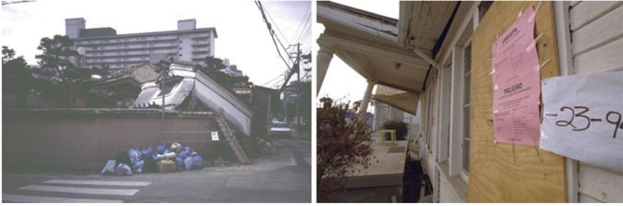
**Fig. 4.1** (L) Typical collapse mechanism of timber houses in the Kobe earthquakes where the entire ground floor is crushed (R) and typical damage observed after the Northridge earthquake in 1994). (Credit: NISEE, University of California, Berkeley, and FEMA, Photographer: Andrea Booher)
