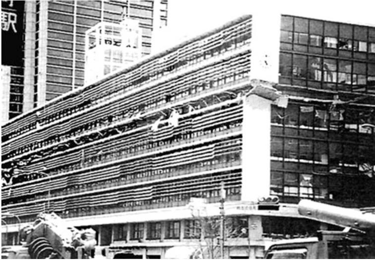
**Fig. 2.14** Photograph shows a single soft storey collapse of a steel frame building (City Hall) after Kobe 1995 (Credit: Courtesy of Earthquake Engineering Field Investigation Team (EEFIT), UK)
