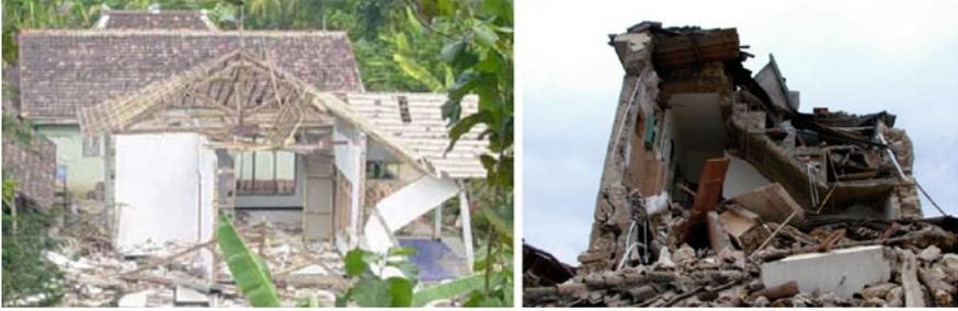
**Fig. 4.4** Collapse of low-rise load bearing brick masonry buildings after the 2006 Yogyakarta, Indonesia (L) and mid-rise collapse in 2009 L'Aquila, Italy earthquakes (Source Author)
