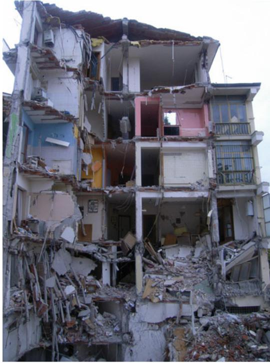
**Fig. 2.12** A multiple RC column failure of a seven storey RC frame building in L'Aquila after the earthquake in 2009 (*Source* Author)
