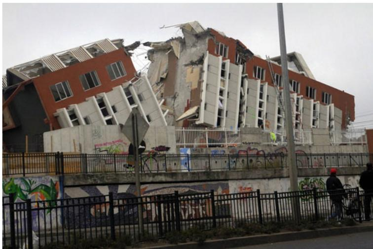
**Fig. 4.12** The overturning collapse of the Alto Rio building in the 2010 Concepción, Chile earthquake. The FR was 9 %. (Credit: Wikipedia)
