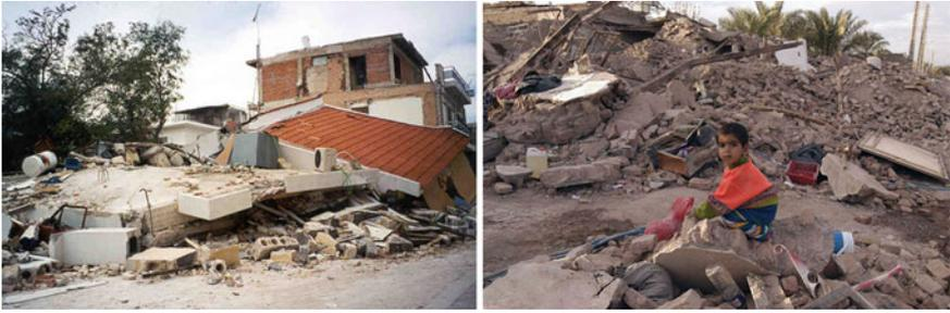
**Fig. 2.16** Complete failure of a non-ductile reinforced concrete frame with brick infill walls structure in Ano Liosia during the Athens earthquake of 1999 (L) and (R) collapse of unreinforced masonry buildings after the Bam 2003 earthquake (Source Pomonis and Flickr)
