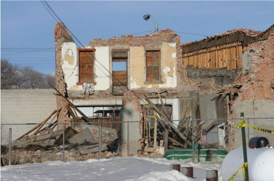
**Fig. 2.9** A house has its roof collapsed after an earthquake in Nevada, 2008 (Credit: EERI, Photographer: Steven Bartlett and Chris Pantelides)
