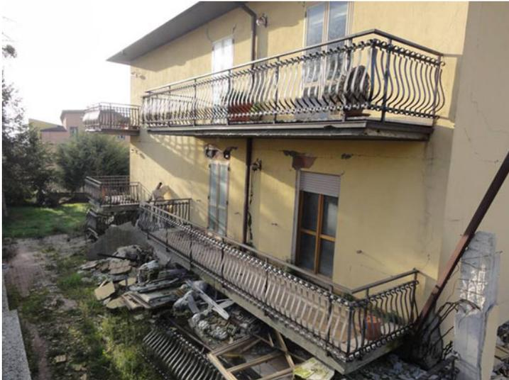
**Fig. 2.13** A soft-storey collapse of a reinforced concrete building after the 2009 L'Aquila earthquake (*Source* Foulser-Piggott 2014)
