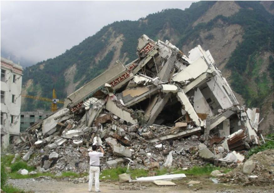
**Fig. 4.5** Total collapse of a dormitory, 2008 Wenchuan (Credit: EERI, Photographer: Dennis Lau)
