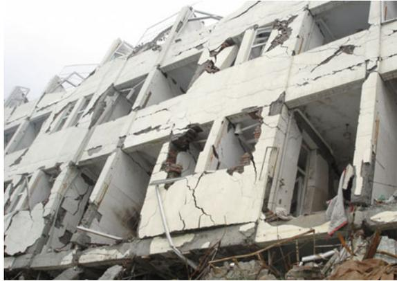
**Fig. 4.10** Complete failure of a seven-story reinforced concrete frame structure with hollow-brick infill in Golcuk after the Kocaeli Earthquake of 1999 (Source NOAA National Geophysical Data Center)
