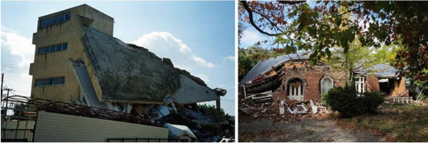
**Fig. 2.11** Multiple wall failures resulting in an overhang collapse observed after the Athens 1999 event (Source Pomonis 2000) and an unreinforced masonry (URM) collapse after the Christchurch earthquake of 2011 (Source Flickr)
