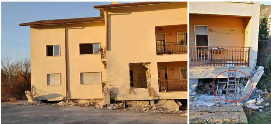
**Fig. 2.15** Soft storey collapse of a reinforced concrete frame building in after 2004 Moroccan earthquake at Al-Hoceima. Zooming into the building as shown on the right, the chances of survival clearly depend on the available space. (Source Flickr)
