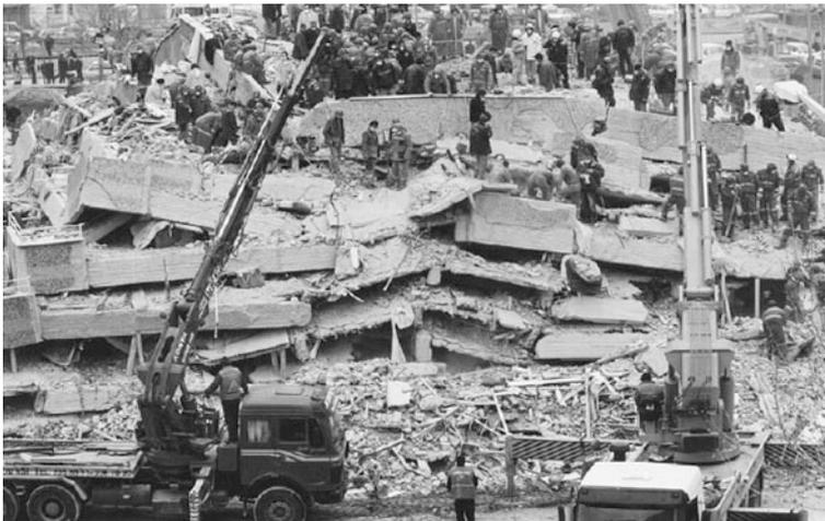
**Fig. 4.15** General view of the totally collapsed Zumrut Apartment Building in Konya City, a non-earthquake collapse (Source Özdemir 2008)
