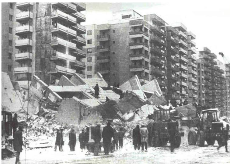
**Fig. 4.13** A RC high-rise collapse (overturn) in Bucharest 1977 (a section of Bloc OD16) with a FR  $\sim 25$  % (Credit: URBAN-INCERC, reproduced with kind permission)
