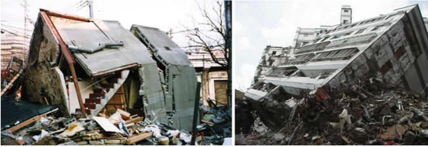
**Fig. 2.17** Overturning collapses observed after the Kobe earthquake of 1995 (L) (Credit: EERI) and overturning collapse witnessed in Taiwan after the Chi Chi earthquake (R) (Source F. Naiem)
