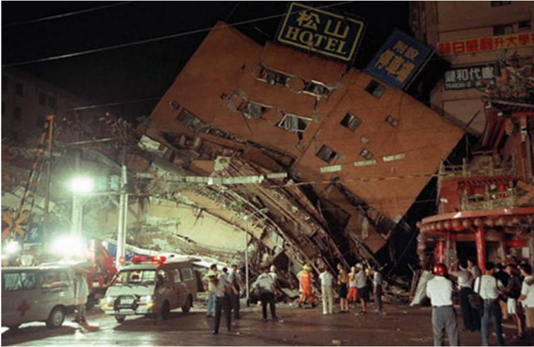
**Fig. 4.14** RC shear wall collapse (overturn) example from the 1999 Chi Chi earthquake in Taiwan (Credit: Wikimedia)
