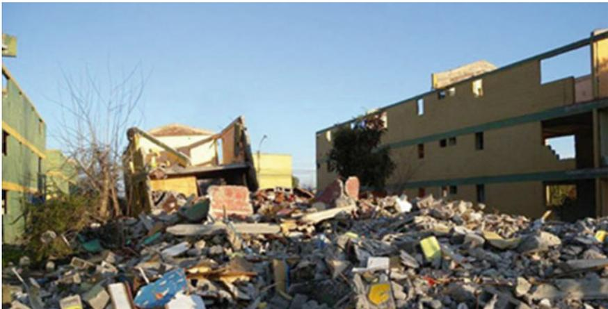
**Fig. 4.6** Collapse of a three-storey confined masonry building in Santa Cruz (2010 Maule, Chile) earthquake (Source Svetlana Brzev)
