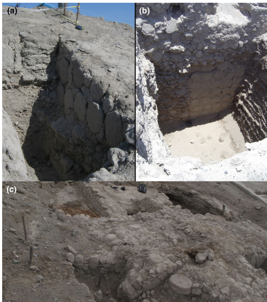
Fig. 20.3 The excavations commonly unearth a variety of building technique, revealing several phases of reuse of structures and spaces. a–b A wall built in conical adobes and the filling of spaces between walls and the closure of a gate or corridor are shown, respectively. c Depicts the superposition of walls belonging to different phases. The difficulty in the processing of geophysical data (in particular GPR data) and the interpretation of results is not only due to the low geophysical contrast between target (e.g., wall, filling, tombs) and medium (subsoil), but also to the complexity of building succession and reuse of materials
