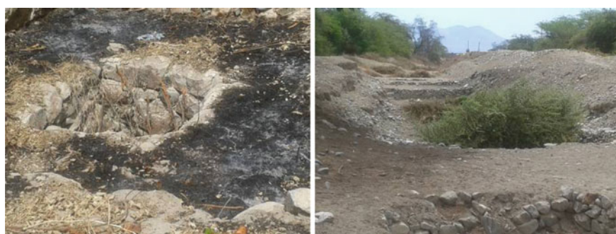
Fig. 13.13 Critical issue of the conservation of filtration galleries: the lack of maintenance. The images show some detail of San Carlos puquio (Photo by Rosa Lasaponara)
