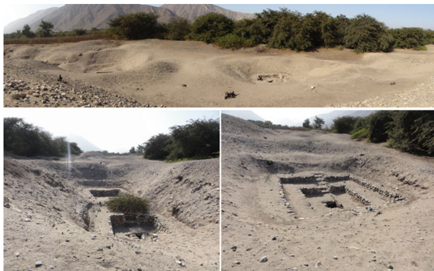
Fig. 22.16 Puquio of Santa Maria. General view of the aqueduct and details of chimneys surrounded by a square, stepped structure built with pebbles
