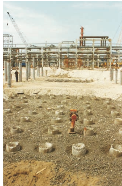
Figure 1.3 Engineering works example – piled foundations.
