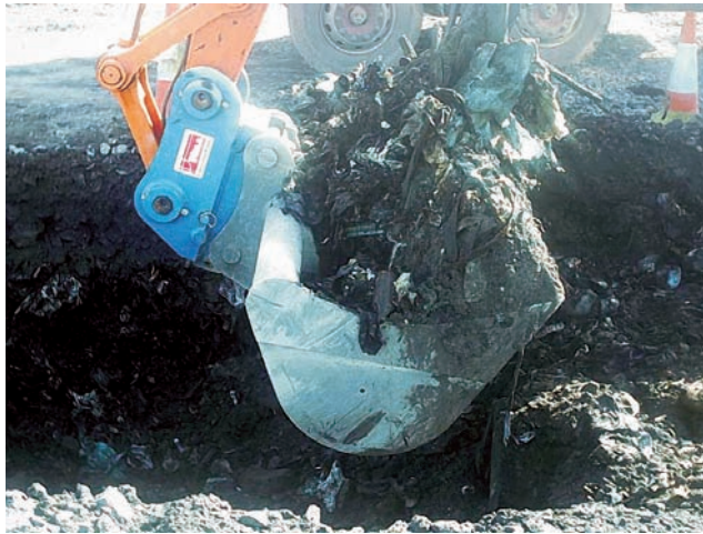
Figure 14.3 Landfill showing heterogeneity and large pieces of materials.
