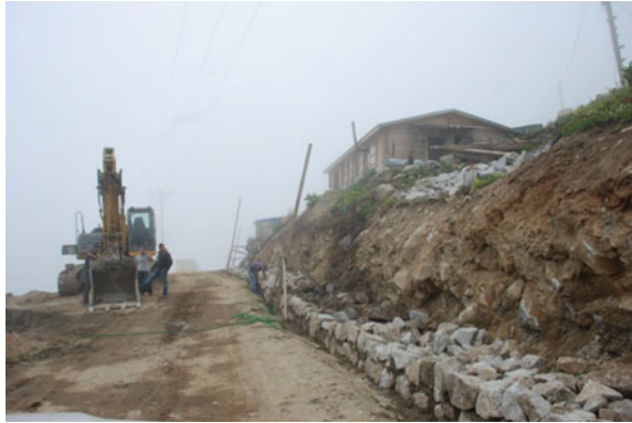
Fig. 5.9 A view from the Green Way Construction in Yukari Kavron Yayla
