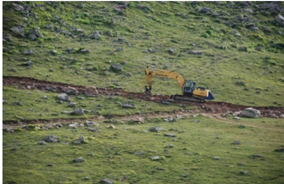
Fig. 5.10 A view from the Green Way Construction in Samistal Yayla
