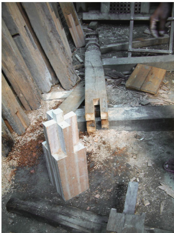
Fig. 2 Bhaktapur, Fifty-Five-Windows Palace. Replacement of weathered bases of timber posts to preserve as much of the old fabric as possible. Photo by Sudarshan Raj Tiwari, 17 August 2004
