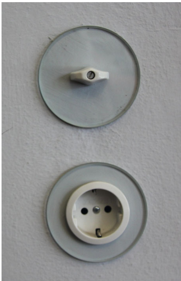
Fig. 8 Dessau, Kandinsky/ Klee House, restored to its original shape in 1998. The electric fittings were replaced by commercially available remakes of the originals. Photo by Niels Gutschow, 23 June 2009
