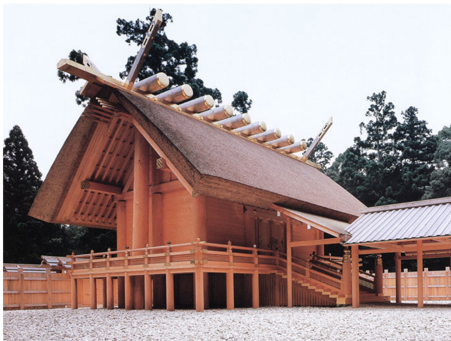
Fig. 29 Ise, the main sanctuary (Jap. shōden ) of the outer shrine, Gekū, after its renewal in 1993. Incised fittings in gilt copper on the grain ends and jewel-like tops on the railing are indicative of a procedure that allows innovations. Source: Brochure “Jingū”, n. d., 14
