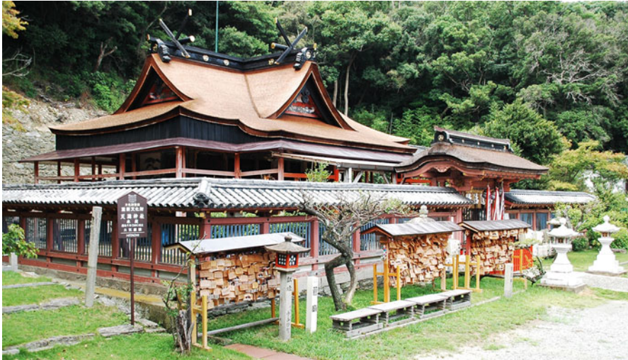
Fig. 6 Tenmanjinja Honden—Elevation. The Main Hall of the Tenman Shrine near Wakayama built in 1604 underwent restoration in 1975. The roofing was replaced, as was the so-called box ridge. Source: Wakayama Center for Cultural Properties
