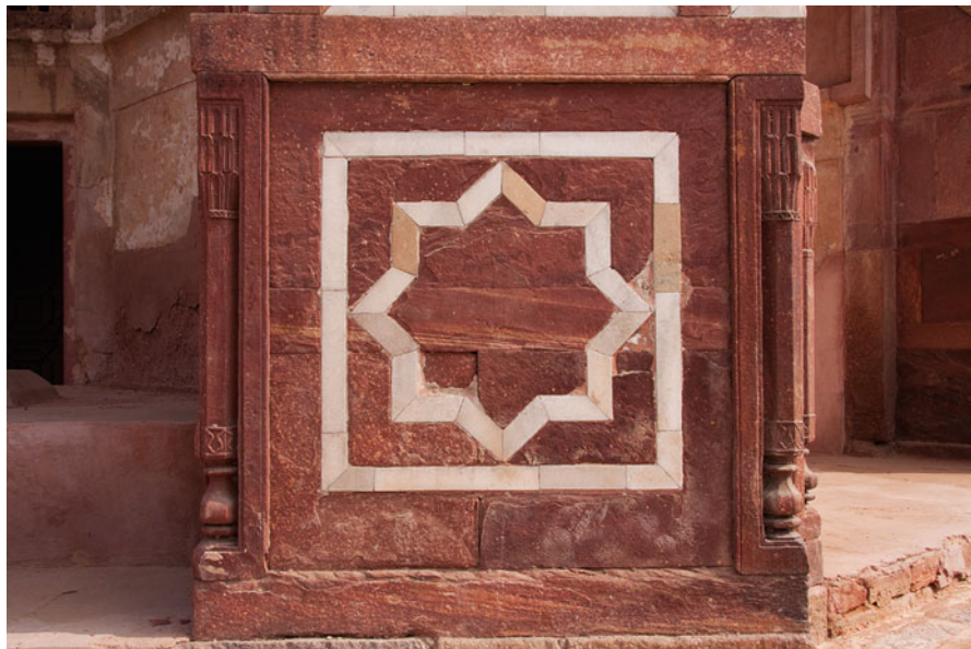
Fig. 7 Humayun's Tomb, terrace level, west side. The repetitive ternary, horizontal pattern of the sandstone work and its marble inlay is a significant feature of the original architectural geometry of the façade pattern and testifies to the design intentions of the builder. Building with red sandstone and white marble was a common characteristic of fourteenth century architecture in the Delhi Sultanate. The combination of these differing stones in Indian architecture was neglected during the fifteenth century, but under the Mughals it was revived and became the standard means of finishing a building. Photo by Niels Gutschow, 14 November 2009
