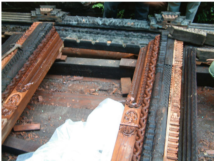
Fig. 3 Bhaktapur, Fifty-Five-Windows Palace. Weathered or lost parts of the decorative timber door frames of multiple parts were carved and fitted according to the old design. Photo by Sudarshan Raj Tiwari, 17 August 2004
