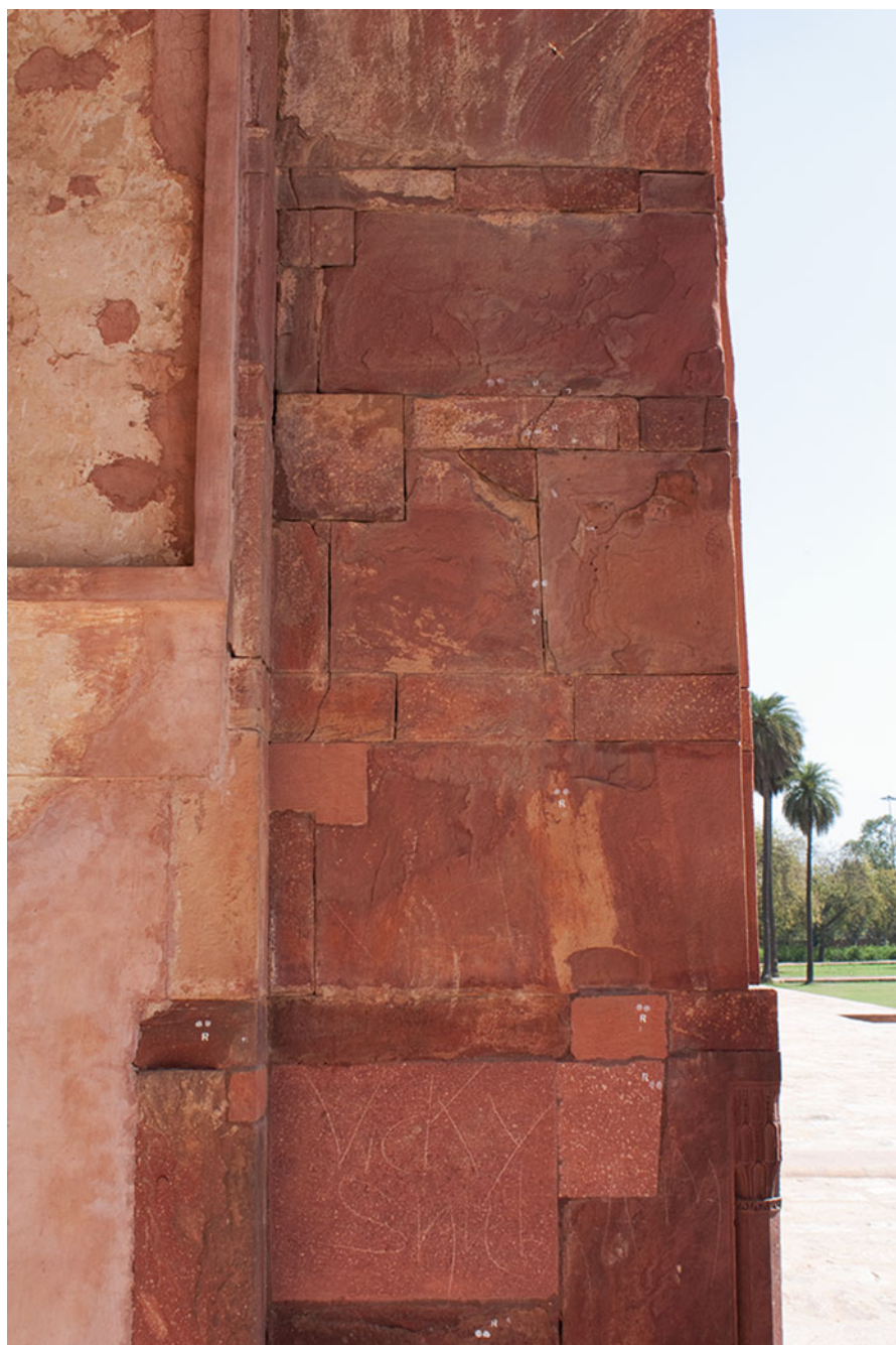
Fig. 8 Humayun's Tomb, terrace level, south side. Repairs undertaken by the Archaeological Survey of India form a patchwork that illustrates the ASI's archeological perspective and conservation approach. The intention is to keep the authentic material and to gradually take any deteriorated element out while neglecting the architectural integrity and the original design intentions of the builder. The issue of the archeological versus the architectural approach was
