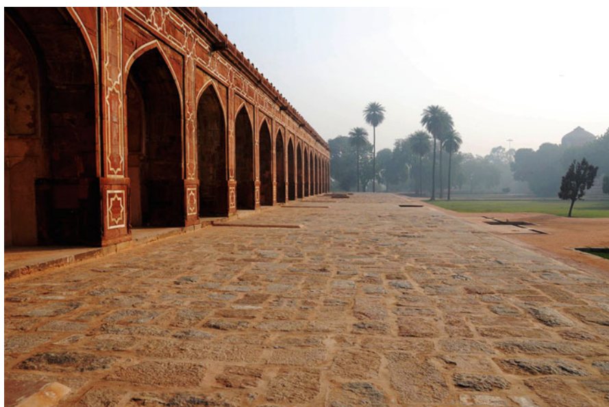
Fig. 10 The unsightly concrete layer on the lower plinth of Humayun's Tomb was removed to restore the original Mughal period quartzite paving in its original patterns. Photo by AKTC © Aga Khan Trust for Culture
