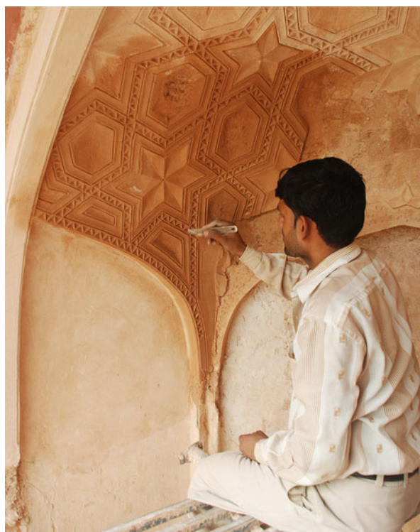
Fig. 11 Master craftsman restoring the ornamental plasterwork of the lower cells of Humayun's Tomb. Half-domed ceilings of the external alcoves of Humayun's Tomb were originally decorated with incised plasterwork with star patterns. Master craftsman restoring the original pattern in lime mortar. Photo by AKTC © Aga Khan Trust for Culture
