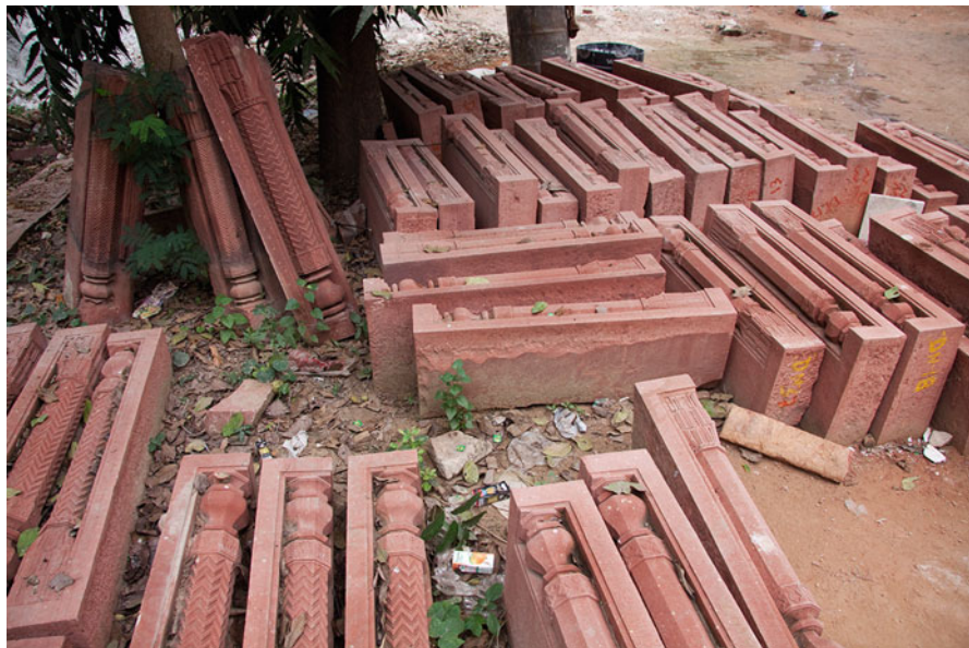
Fig. 4 Humayun's Tomb, stone workshop. The decorative sandstone dwarf corner pillars for the terrace and ground-floor level are dressed by craftsman according to the original form, using the same building traditions that were used in the original construction. Diverse quarries in Rajasthan were surveyed to find out where appropriate stone was available for the replacements. In a few years, the new material will have a patina and resemble the authentic material. In order to document the replacements visibly, small marks were put on each stone. Photo by Niels Gutschow, 14 November 2009
