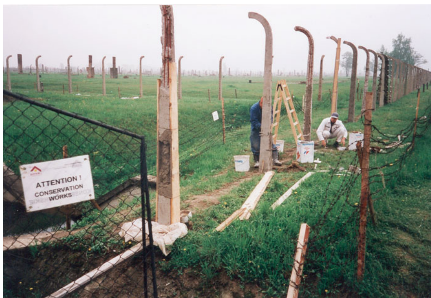
Fig. 6 Oświęcim/Auschwitz. On the compound of the former Nazi concentration camp the severely weathered concrete posts got a new mantle in the course of a recent conservation measure. The rusted barbed wire, spanned between the posts, was replaced. Photo by Niels Gutschow, May 2001
