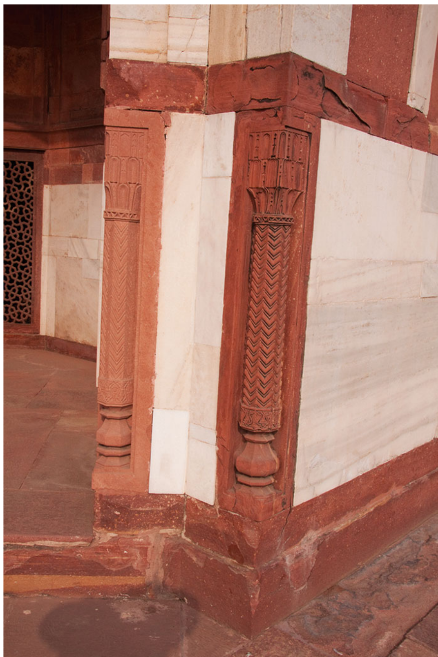
Fig. 5 Humayun's Tomb, south side, ground floor level. Two sandstone dwarf corner pillars, the right-hand one supposedly reputed to be original material fashioned by sixteenth-century craftsmanship, the left-hand one being a recent replacement of mediocre quality rather than a true copy initiated by the ASI. Photo by Niels Gutschow, 14 November 2009
