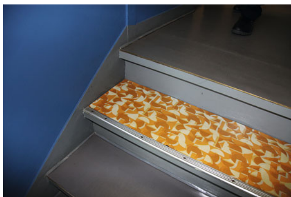
Fig. 7 Dessau, Kandinsky/Klee House, restored to its original shape in 1998. The stairs were returned to their original form, but one stair tread was preserved with its linoleum covering and aluminum profile dating back to a renewal in the early 1970s. Photo by Niels Gutschow, 23 June 2009
