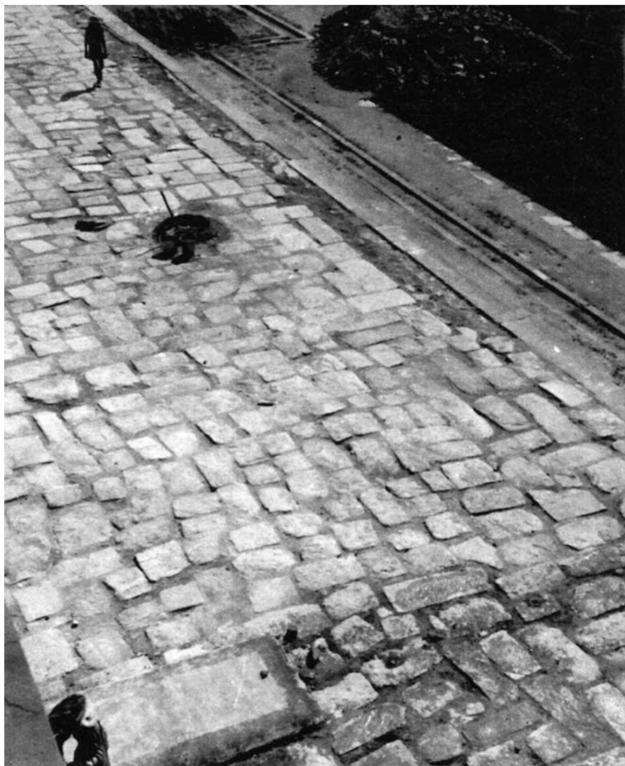
Fig. 9 Humayun's Tomb, plinth. A photo from 1956 documents that the plinth was covered with large quartzite ashlars before the ASI covered it with cement in the late 1950s. Pictured in the Urban Renewal Initiative's Conservation Proposal, March 2008
