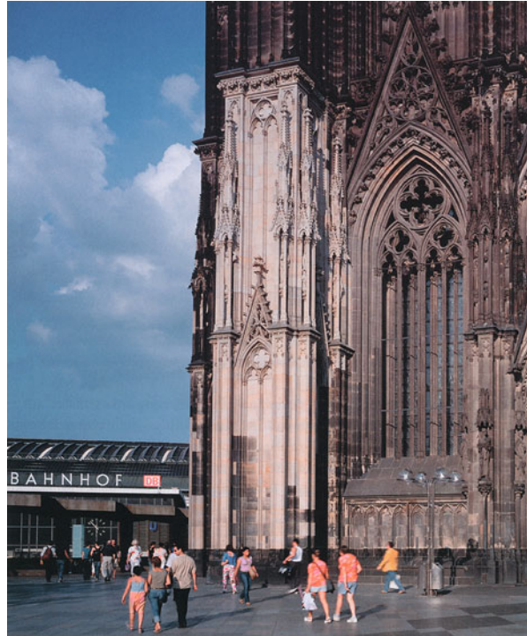
Fig. 42 Cologne Cathedral. Completion of the facing of the “plug” with 103 cubic meters of sandstone from Oberkirchen, August 2005. Source: Schock-Werner 2005, 14
