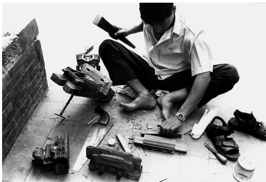
Fig. 31 Patan, Ratneśvara temple at Sulima Square. Indra Kaji Silpakar from Bhaktapur repairs and completes one of the miniature aedicules flanking the doorways of the ground floor. Source: Theophile and Gutschow 2003, 63
