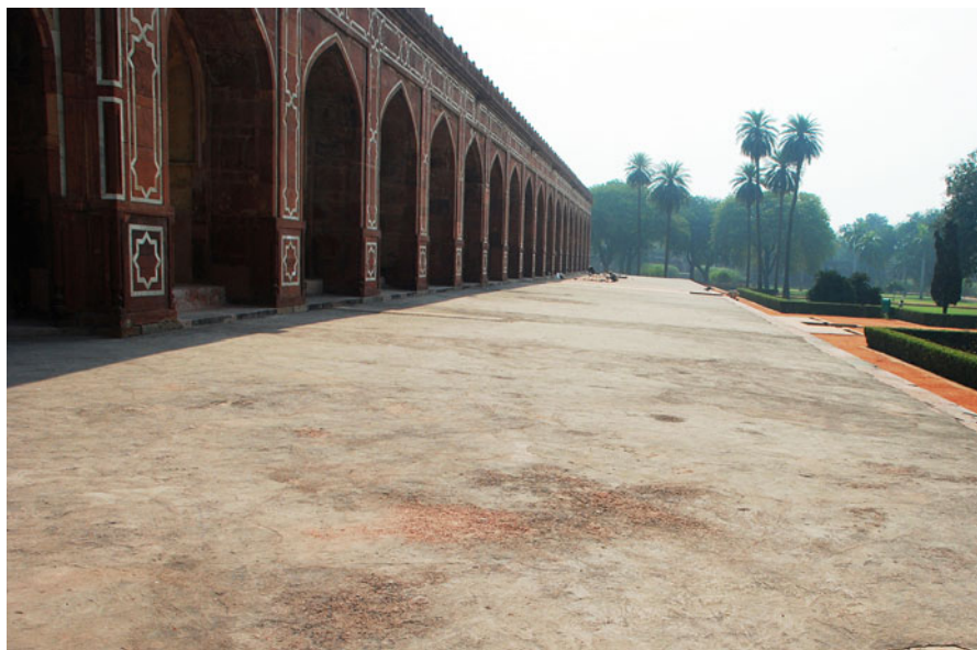
Fig. 9 Lower plinth of Humayun's Tomb with layers of cement concrete, prior to the conservation works. Photo by AKTC © Aga Khan Trust for Culture
