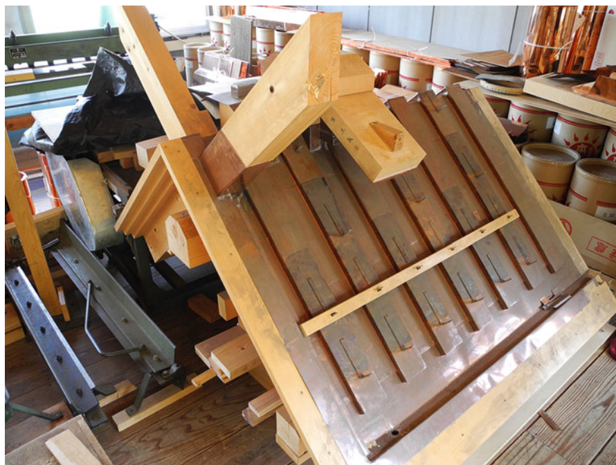
Fig. 15 Yamada Workshop—copper sheet for the roof. The roofs of the major shrines are covered with thatch. This being short-lived and prone to damage, there is a roofing of thick planks underneath. To increase safety even more, these planks are covered with thin copper sheeting as seen on this model in the shrine workshop. Photo by Christoph Henrichsen, May 2011
