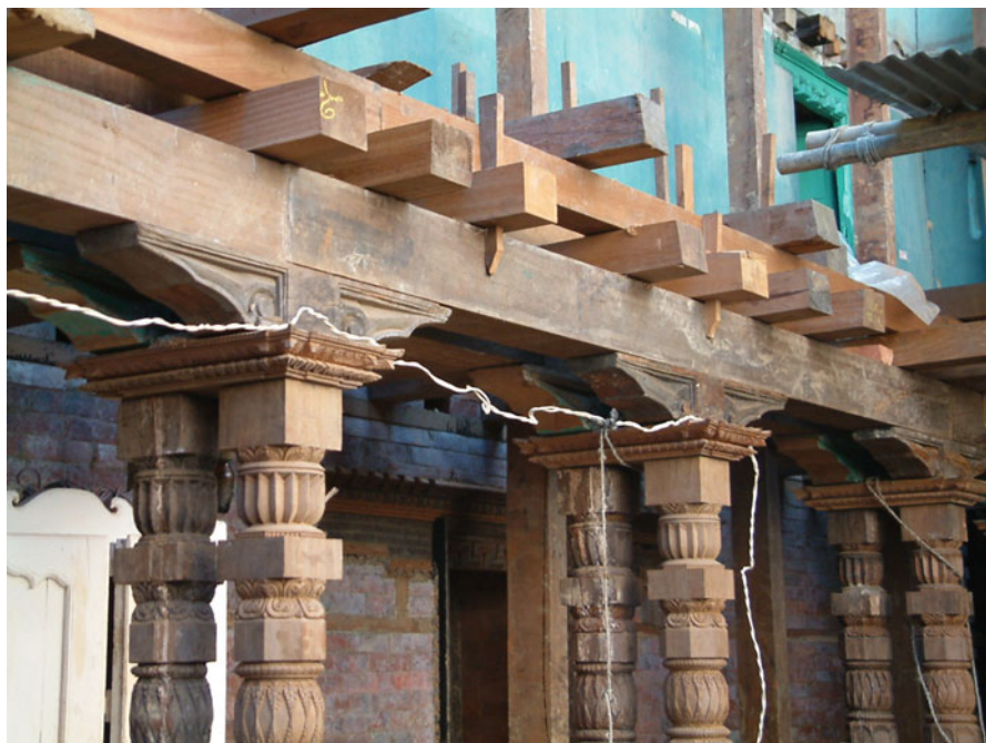
Fig. 1 Bhaktapur, Fifty-Five-Windows Palace. Installation of pairs of old and new posts. Photo by Sudarshan Raj Tiwari, 18 October 2004
