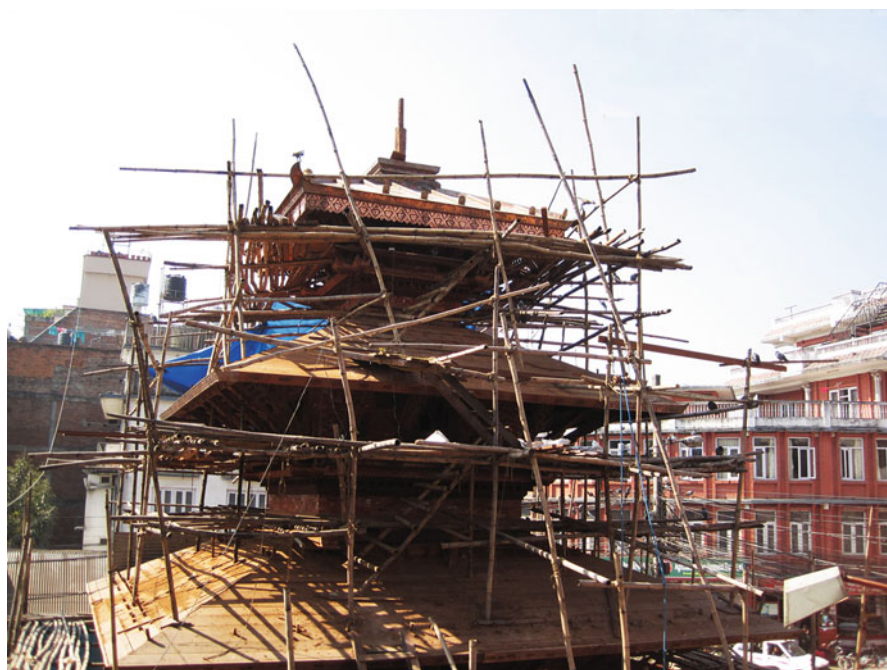
Fig. 4 Naxal Bhagavati, Kathmandu. The temple was completely dismantled since most of its structural parts, such as the existing structural timber beams, the rafters, the core wall around the sanctum, and the roof were feared to be on the verge of collapse. The new base was constructed in the same style and on the same scale as its predecessor in order to retain the original appearance. Photo by Sudarshan Raj Tiwari, 26 February 2011
