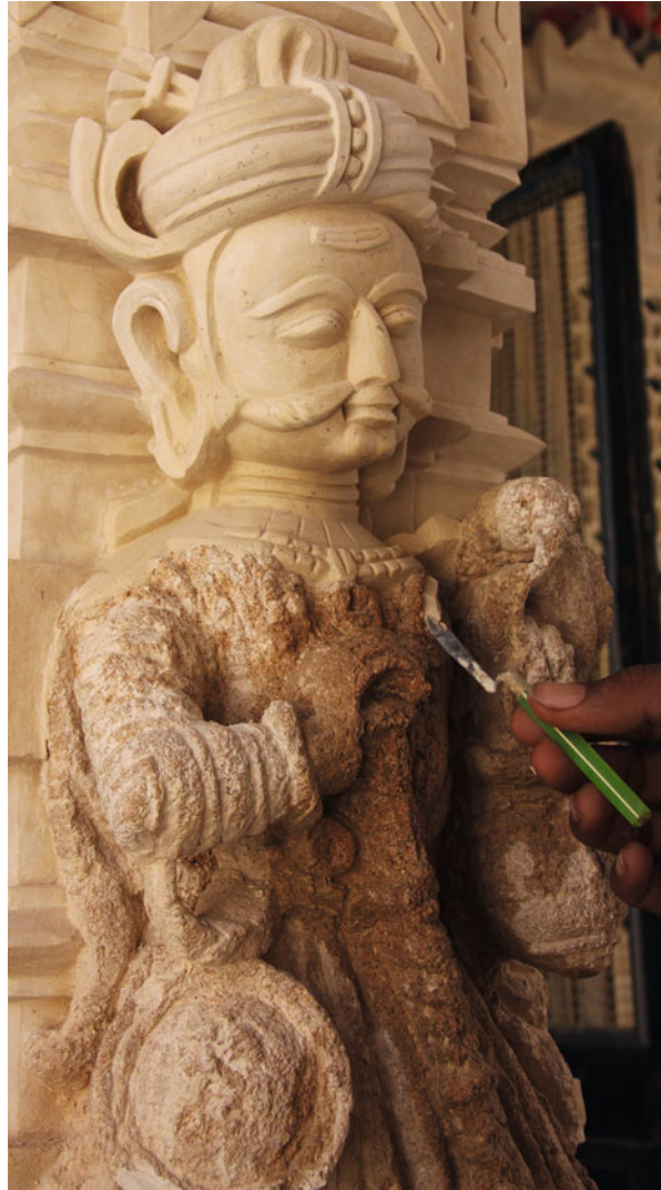
Fig. 22 Detail of a winged celestial musician in the Nandīśvara Dvīpa Temple at Umfai Tuk, established in 1840 by Seth Hemabhai Vakhachand from Ahmedabad. Its regular renewal involves cleaning the limestone and creating a new surface with fine plaster made of lime and stone powder. Photo by Niels Gutschow, 21 November 2009
