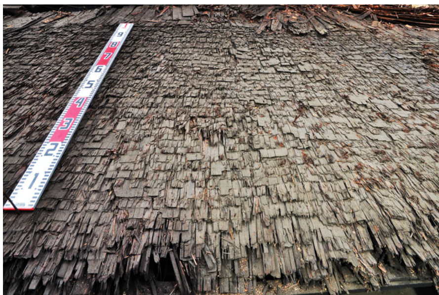
Fig. 8 Kongosanmanin Daidokoro—old roofing. The kitchen building of the temple dates back to the mid seventeenth century. Up to the early twentieth century, a unique roofing technique was used in the mountainous Koyasan region in which layers of cypress bark alternate with thin cedar shingles. This photo shows part of the old roofing. The bark shingles seem to have decayed much faster than the wood shingles. Source: Wakayama Center for Cultural Properties, Kongosanmanin Restoration Office, Tadatsugu Tai
