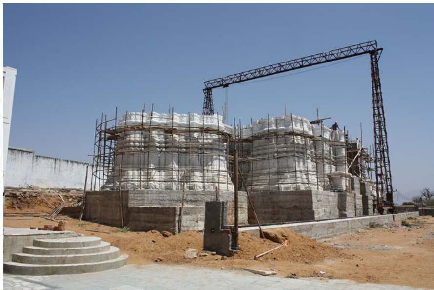
Fig. 22 Varman, sanctuary and eastern mandapa: The marble elements for the Jain temple were designed in Ahmedabad and manufactured in Makrana, then brought to the construction site for the new temple. Photo by Katharina Weiler, March 2010
