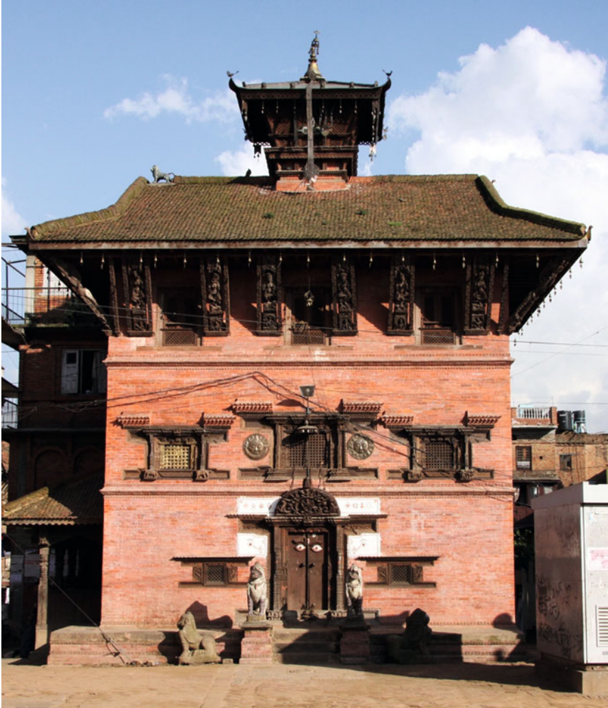
Fig. 13 Bhaktapur (Nepal), replacement of the god-house of the goddess Tripurasundari in 2005–2008. In 2004 it was dismantled and rebuilt using the original struts and a few components of the first floor windows. In response to the wishes of the local community, the building gained 4 feet in height. The crowning spire was redesigned with latticework and copper sheet roofing to reflect eighteenth century prototypes. Photo by Niels Gutschow, 16 October 2009
