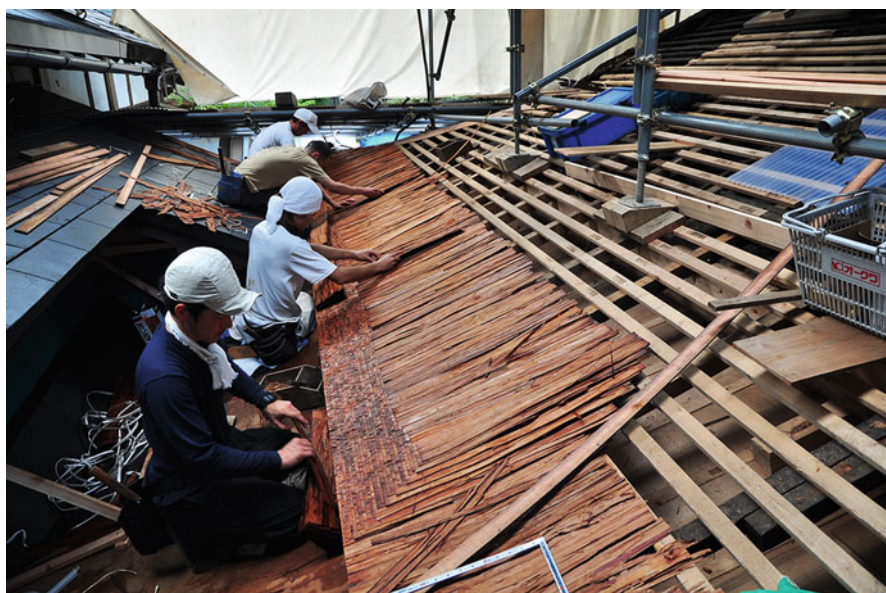
Fig. 9 Kongosanmanin Daidokoro—new roofing. The new roofing carried out in autumn 2010 is entirely made of bark shingles to specifications valid all over Japan. The shingles are fixed to battens with bamboo nails. Source: Wakayama Center for Cultural Properties, Kongosanmanin Restoration Office, Tadatsugu Tai
