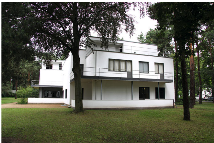
Fig. 6 Dessau, Kandinsky/Klee House, restored to its original shape in 1998. The originally cantilevering slab of the balcony has been replaced by a slab supported by three stainless steel pillars set a little behind the terrace parapet. Photo by Niels Gutschow, 23 June 2009
