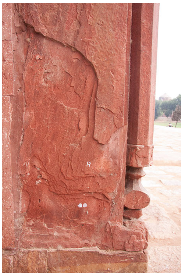
Fig. 6 Humayun's Tomb, west side, ground floor level. Inappropriate conservation work that used cement to fill the joints is one reason for the deterioration of the sandstone. The cement does not allow the water to get out, and the stone starts cracking. Stones marked with an "R" will be replaced. Photo by Niels Gutschow, 14 November 2009
