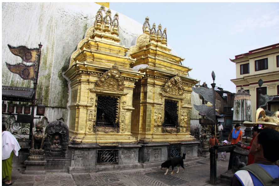
Fig. 32 Svayambhūcaitya, Kathmandu Valley (Nepal). The copper repoussé of all the niches, dating back to a substantial renewal of the caitya in 1918, was re-gilded in 2009, sponsored by the Tibetan Nyingma Meditation Centre in Berkeley. Missing arches with decorative lotus foliage and figural details in high relief were replaced. Photo by Niels Gutschow, 17 September 2009
