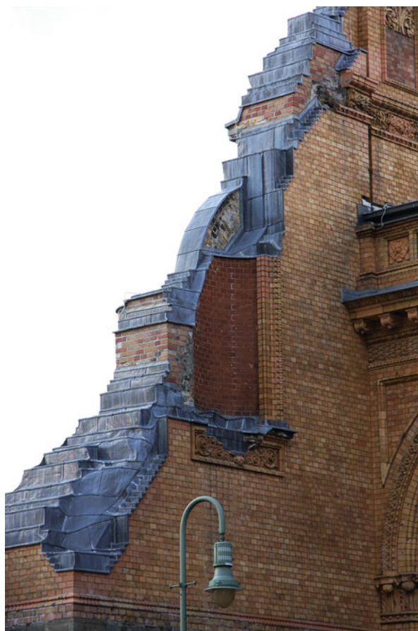
Fig. 3 Anhalter Bahnhof, Berlin. The station was severely damaged during air raids on 3 February 1945. Today, lead sheathing protects the ruined structure from rain. Photo by Katharina Weiler, 13 October 2009
