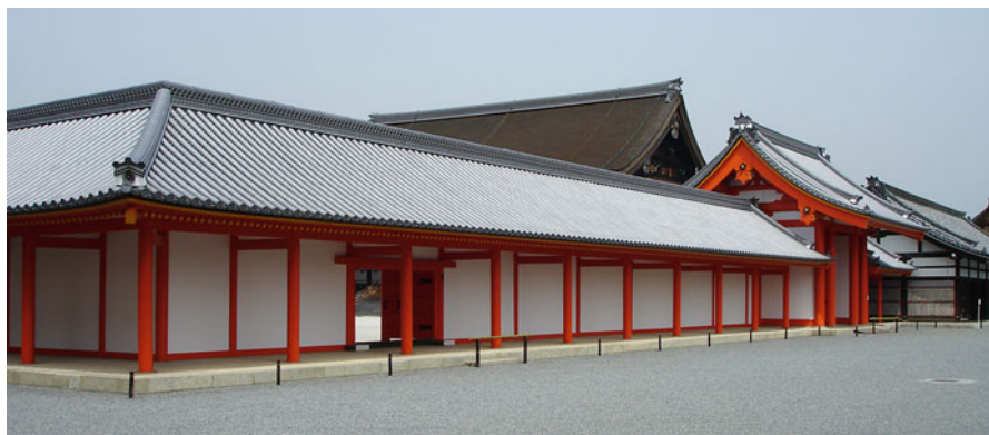
Fig. 10 Imperial Palace. Most Buddhist temples and most historic town houses have tiled roofs. Due to the preparation of the clay—using feet and the varying conditions in the kiln—old tiles come in slightly different colors and surfaces. Maintenance repairs and partial renewal result in very vivid roofing with all shades of grey. Today, the clay for the tiles is prepared by machine and the kiln fired with gas resulting in a very homogeneous color and surface. Maintenance has changed too. In the old days, only severely damaged tiles were replaced, today the roofing is often completely renewed. Photo by Christoph Henrichsen
