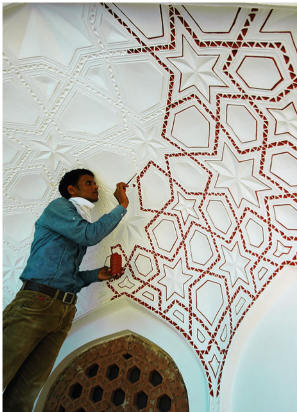
Fig. 12 The final plaster layer comprises a 1:1 lime-marble-dust layer, which is how the Mughals used to mimic marble. Evidence discovered at the tomb suggests that the star patterns are highlighted with red polychromy; they continue the prominent red-white contrast. Photo by AKTC © Aga Khan Trust for Culture
