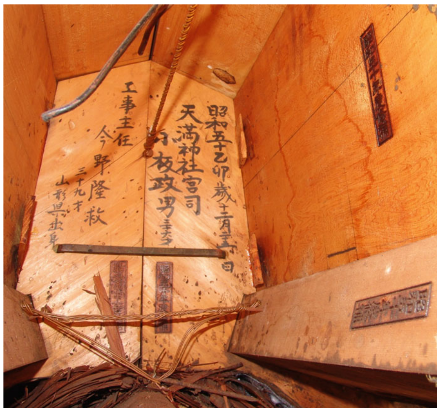
Fig. 7 Tenmanjinja Honden—Ridge. The high ridge on the hipped-and-gabled roof is made of planks. The cypress wood for these extra-wide and long planks was imported from Taiwan. On this photo showing the inside of the ridge, the branding-iron marks can be seen identifying material renewed during restoration and an ink inscription referring to the names of the head priest and the architect in charge. Source: Wakayama Center for Cultural Properties
