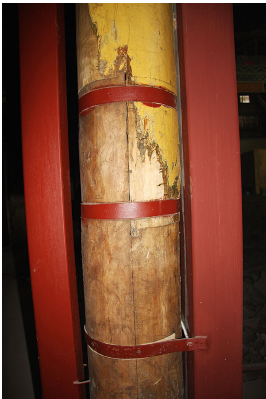
Fig. 4 Yisu Society Theater, Xi'an. Timber columns and their iron supports. The rotten bottom ends of the decrepit columns were cut away and joined with the same kind of wood. Iron bands were added around the joints to reinforce them. Steel reinforcements were added on both sides of the columns. Photo by Shaohua Grasmück-Zhang, 21 September 2010
