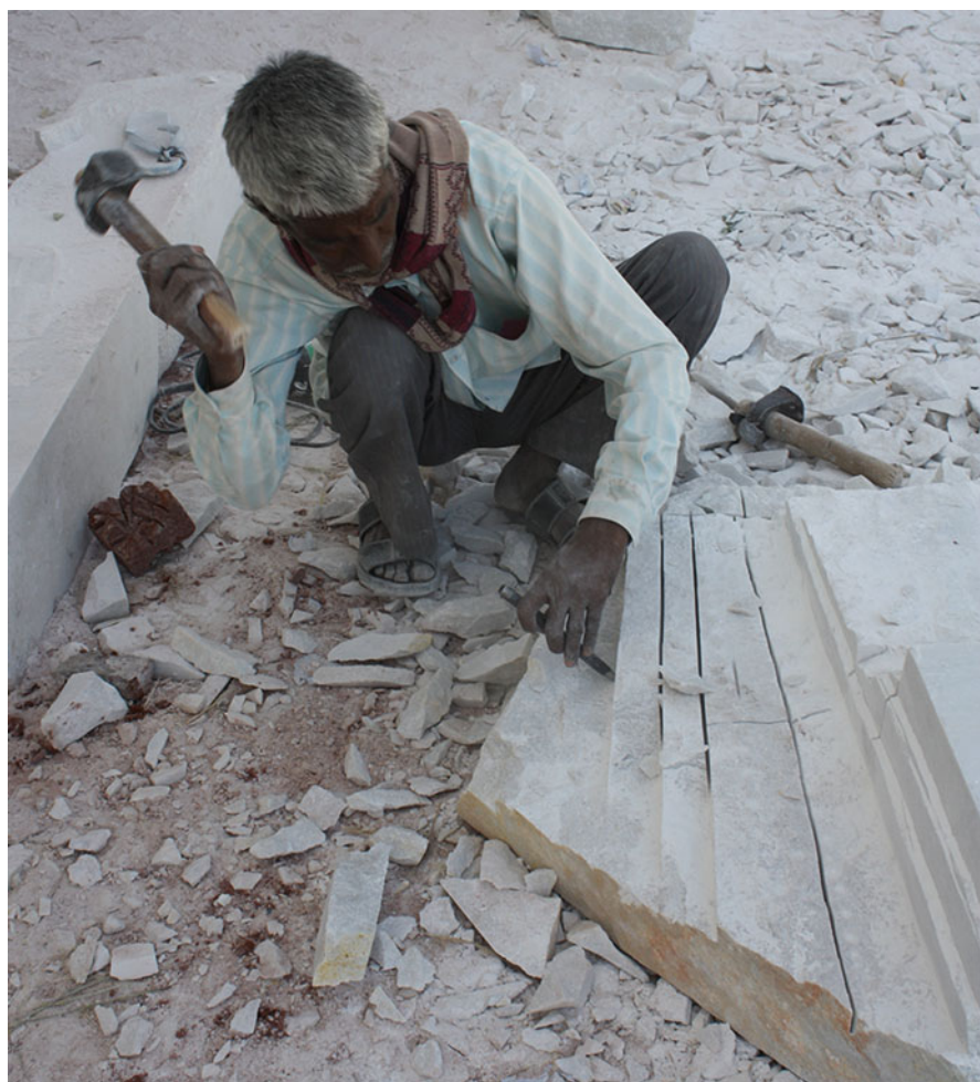
Fig. 17 Makrana: A mason uses a heavy chisel and a hammer to chip off the superfluous parts of an ashlar. Photo by Katharina Weiler, March 2010
