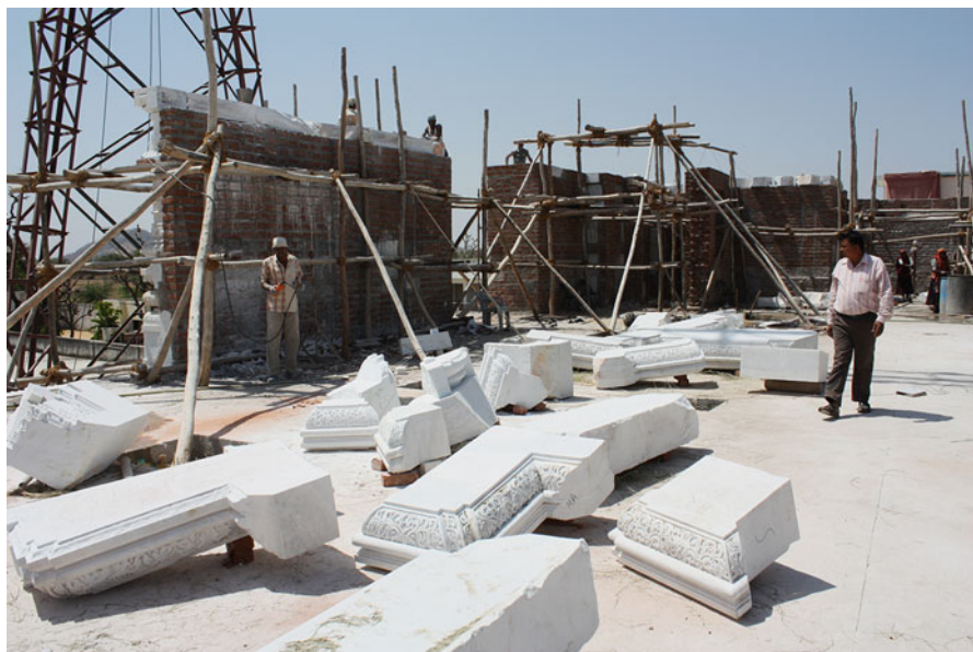
Fig. 23 Varman: Elements of the “H” layer manufactured in Makrana and ready to be placed on top of layer G in the construction process. Photo by Katharina Weiler, March 2010
