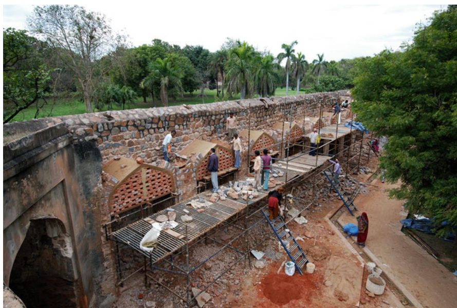
Fig. 13 Conservation of the enclosure wall of Humayun's Tomb. Master craftsmen have used traditional materials and building techniques employed by the original builders to complete the portions of the wall that had collapsed in the twentieth century. Photo by AKTC © Aga Khan Trust for Culture
