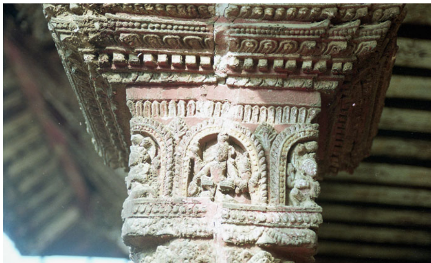
Fig. 24 Bhaktapur (Nepal), Nyatāpvala Temple. The beautification program initiated by King Mahendra in 1962 had the entire temple covered with a coat of paint (hitherto unknown in Newar architecture) for which a smooth surface was produced by filling in cracks with cement mortar. Photo by Niels Gutschow, 4 November 2007
