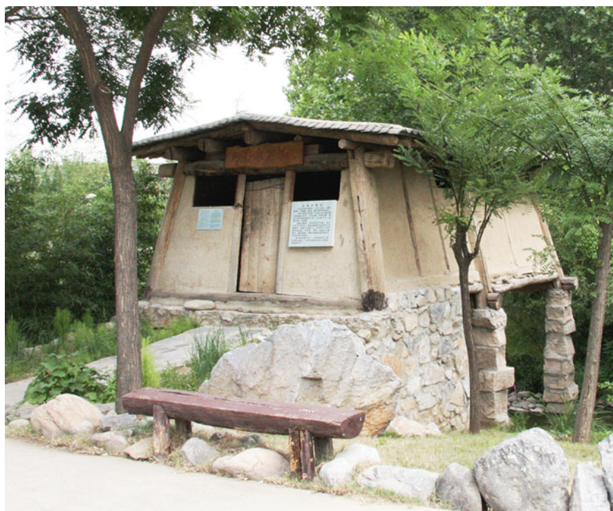
Fig. 4 China Nationalities Museum, Beijing. A water-powered grain mill from Longge village in the Huzhu Tu Autonomous County of Qinghai Province, probably dating back to the second half of the nineteenth century, has been moved to the Tu Museum. It is situated on the banks of an artificial creek. The water mill is built of stone and wood and its outer walls are plastered with mud. Wire netting, a “modern” material, has however been used to make the mud walls more durable. Part of the building hovers 2.6 m above the creek, supported by stilts masoned with ashlar. The grinding mechanism is regarded as “an intangible heritage,” while the mill as a whole is accorded the status of a “first-grade cultural relic of the museum” (Chin. 一級文物 Yiji wenwu ). Photo by Katharina Weiler, 8 September 2010
