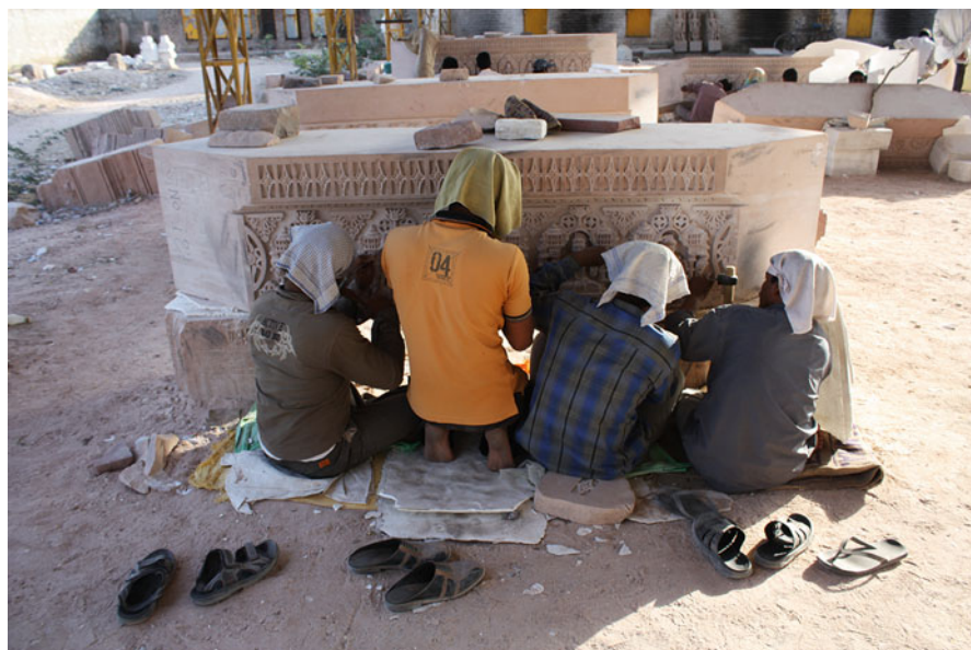
Fig. 12 Four craftsmen from Orissa kneel in front of a rectangular stone block to do the fine carving on five Swamy images for the Swaminarayan Temple in Nagpur. The sandstone was mined in Bansipaharpur near Bharatpur in Rajasthan. Photo by Katharina Weiler, March 2010
