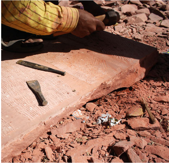
Fig. 5 Stone workshop at Humayun's Tomb, Delhi: Training of the youngsters and newcomers in basic techniques, for example the working of the raw stone slabs from the quarries in a three-step system. In order to obtain the required depth, extra layers were initially removed from the sandstone with a pointed chisel ( gadai ). This gave the stone a temporary texture. After that, the surfaces of the stone were subdivided into regular partitions with a wide chisel ( dalpai ). This method made it easier to achieve a regular overall surface since these fields were removed progressively with a wide chisel. Work with a pointed chisel resulted in a pointed surface, whereas the wide chisel was used for smooth textures. The craftsmen at Humayun's Tomb worked with approximately 50 different kinds of chisel, gadai , and dalpai . In the end, the worked stone slabs could be used for the further stages of the work, e.g., for grill windows ( jali ) or pillars. They were the basis for the carving of those elements designed to replace original material that had deteriorated beyond repair. Photo by Katharina Weiler, March 2010
