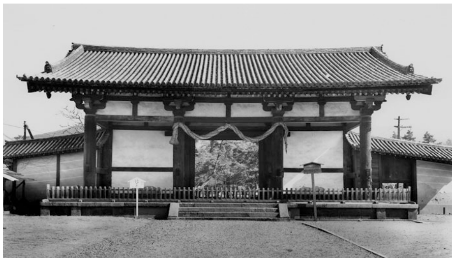
Fig. 5 Tōdai-ji Tegai-mon. The Tegai-mon is the only gateway of the famous Nara temple dating back the founding period in the mid eighth century. The gate was altered and raised around the year 1200. During restoration work carried out in 1931, the gate was not restored to its original state. Source : Nara Board of Education, Department of Cultural Properties
