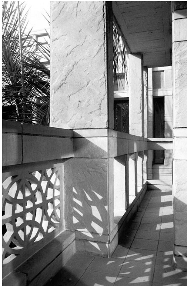
Fig. 6 World Bank Building, New Delhi. The detail of a balcony presents handicraft sandstone cladding, a characteristic building material for the Delhi, Gujarat, and Rajasthan region. Architect Raj Rewal has integrated elements manufactured through craftsmanship into modern building design in order to preserve a certain authenticity linked to the Indian crafts tradition and to emphasize the play of light and shadow on the stone's surface. Source: Jahanbegloo and Rewal 2010, 69. Photo by Ferrante
