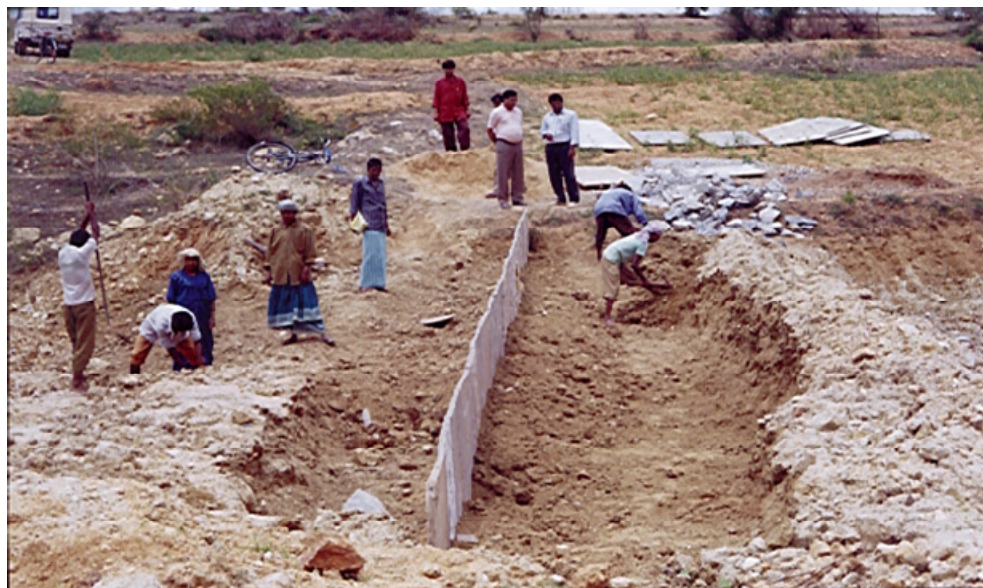
Fig. 17. Providing sub-surface drainage to manage soil salinity/alkalinity
