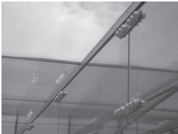
Figure 17.2 Structural glass: Glasgow Medical School – roof support beam, detail.
