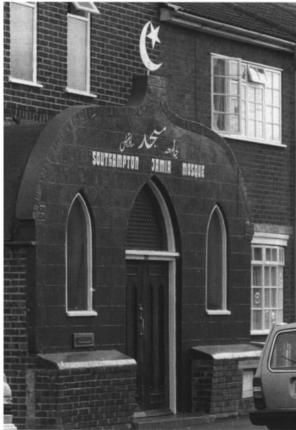
FIGURE 5.3 A terrace house is turned into a mosque
