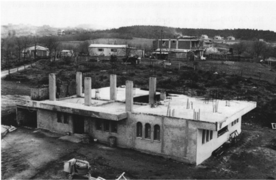
FIGURE 2.4 Illegal housing in Istanbul
