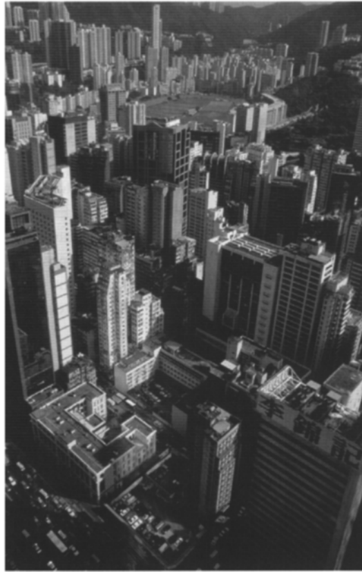
FIGURE 6.13 The densely packed high-rise buildings of Hong Kong
