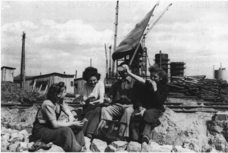
FIGURE 7.5 Youth workers take a break from building the future in the German Democratic Republic 2.2
