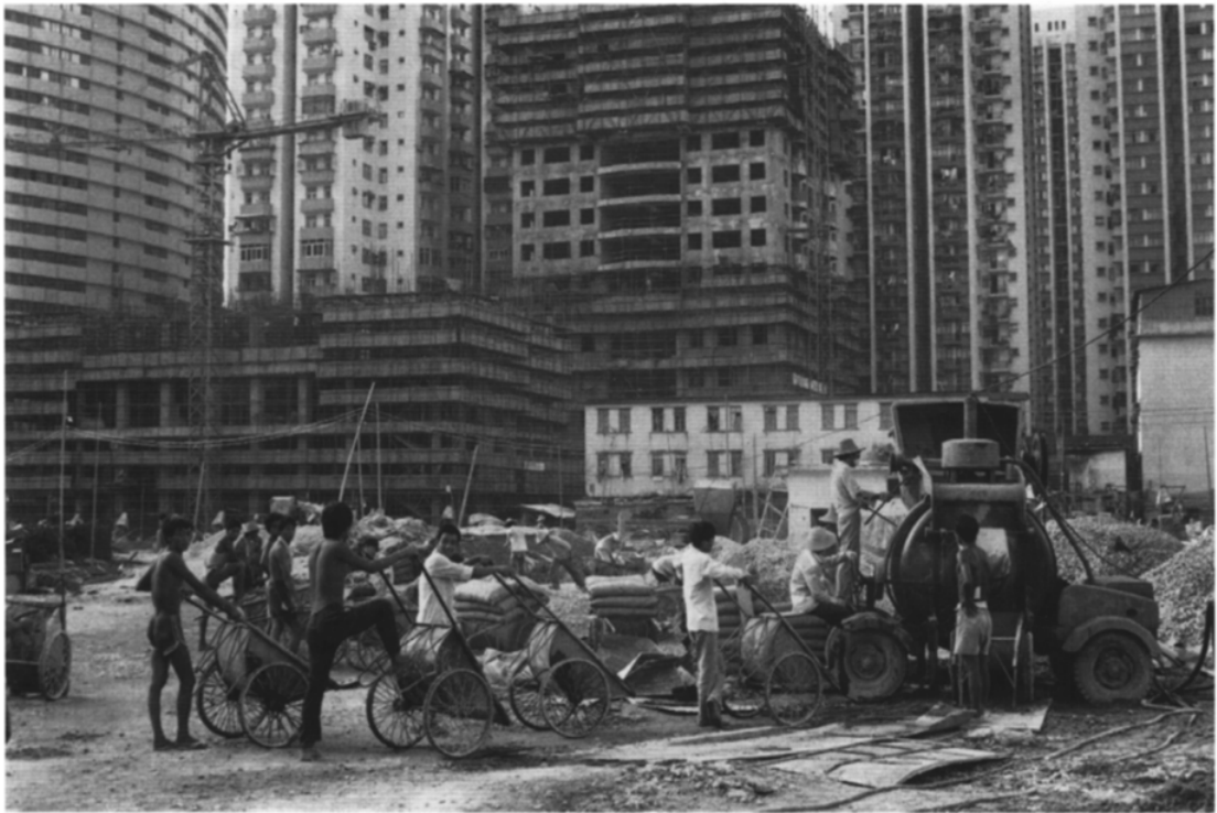
FIGURE 6.14 Construction sites in China's cities attract many migrant workers
