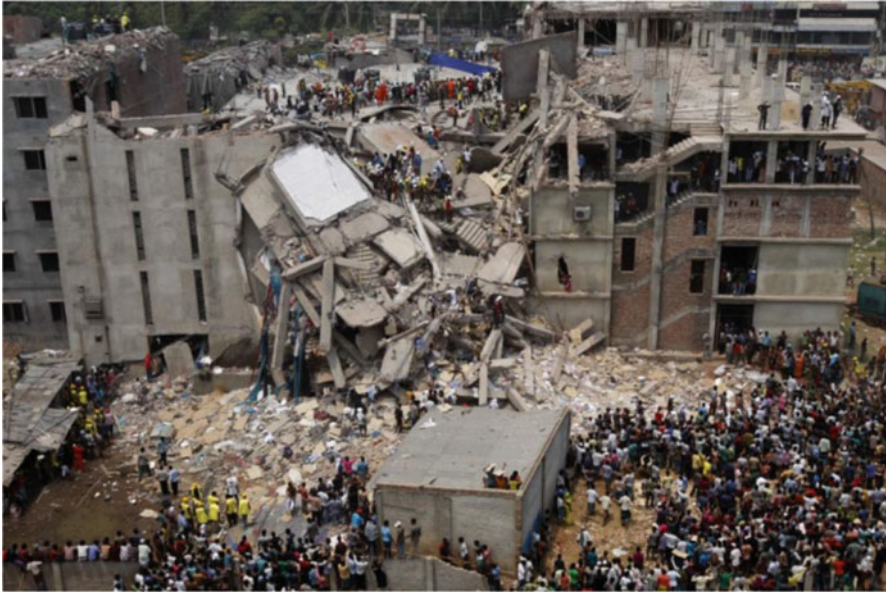
Fig. 3.7 Rana Plaza factory building after collapse (Wikipedia Commons 2013 )
