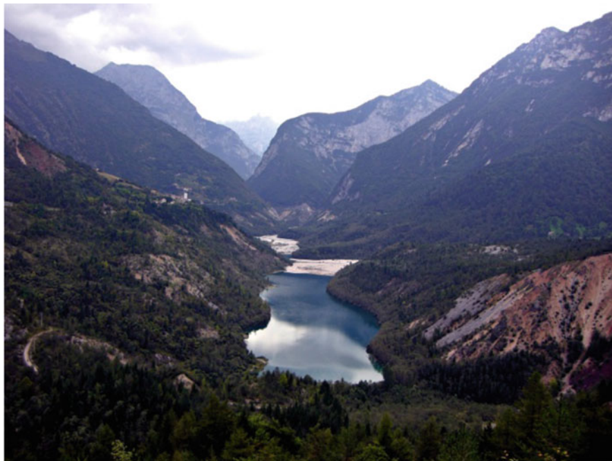
Fig. 3.5 Behind the Vaiont Dam – reservoir filled in by landslide (Wikipedia Commons 2013 )
