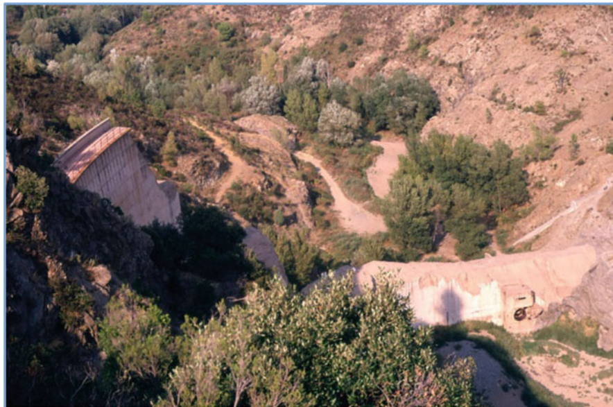
Fig. 3.3 The failed Malpasset Dam (Wikipedia Commons 2013 )
