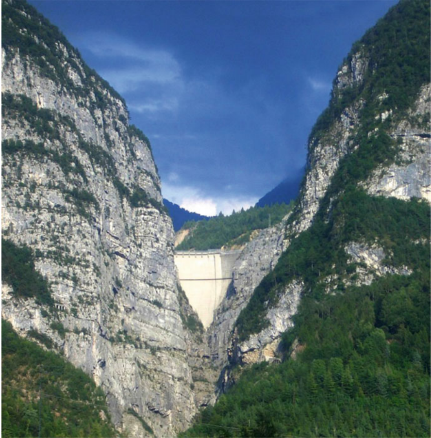
Fig. 3.4 The Vaiont Dam, as seen below from the town of Langarone (Wikipedia Commons 2013 )
