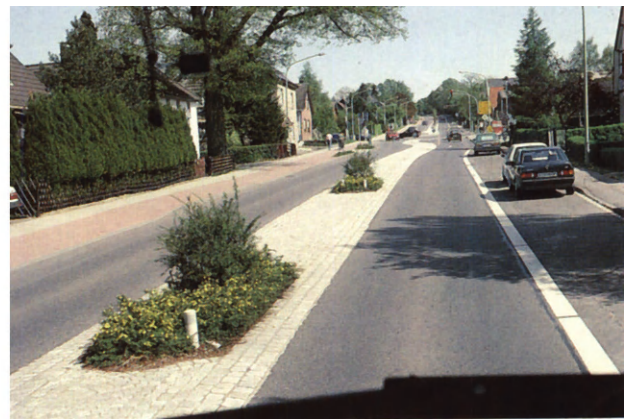
Plate 11. Design of median strip prevents overtaking whilst enabling manoeuvring, Aachen, Germany (see p. 128).
