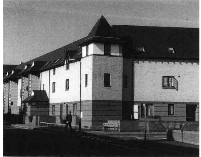
Figure 17. New development (1992); Moseley and District Churches Housing Association, Balsall Heath, Birmingham. Architects: Databuild Ltd.
