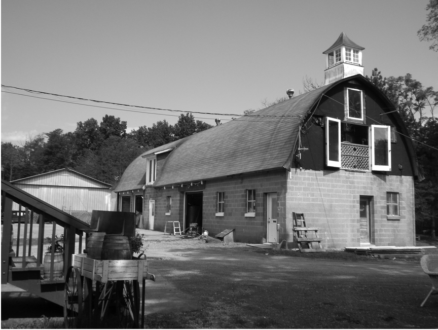
FIGURE 4. The converted granary building with Tuthilltown's main operation. Photo by the author.
