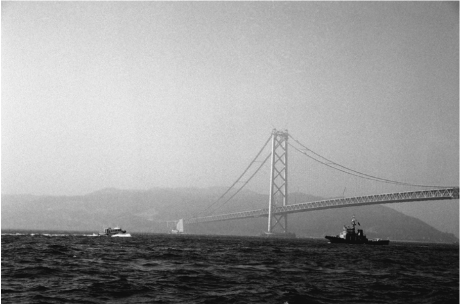
Figure 12.1 Akashi-Kaikyo Bridge, Japan.
