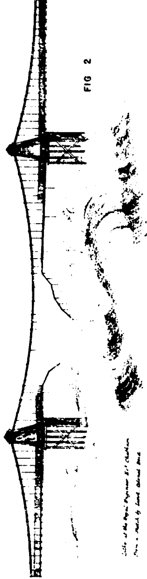
Figure 1.10 Failure of the Brighton Chain Pier, 1836.
