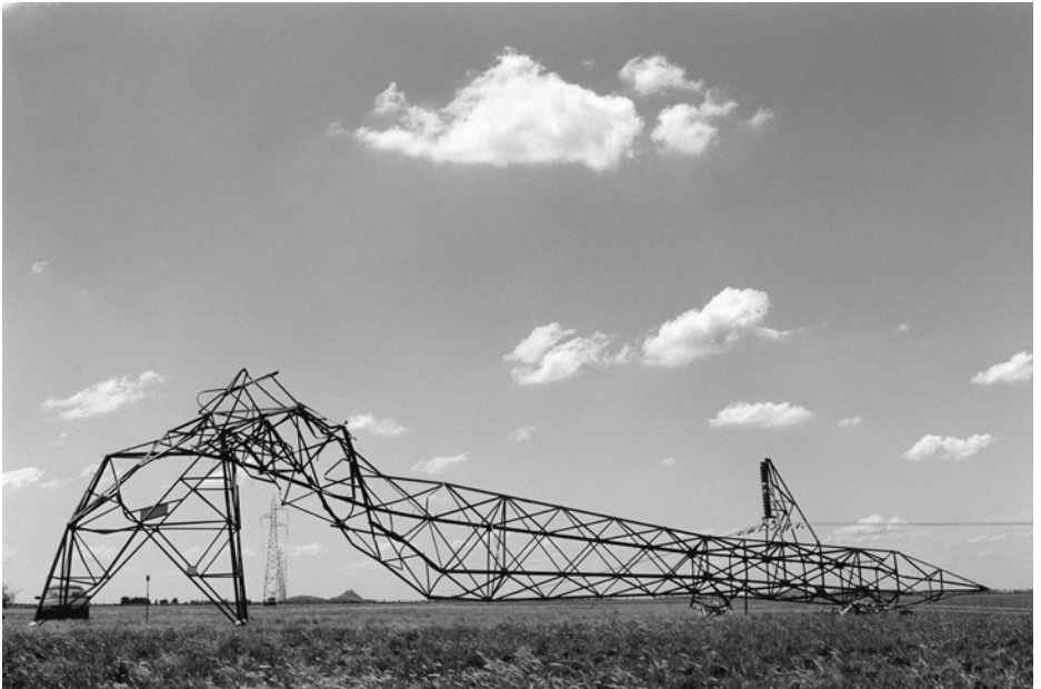
Figure 13.4 Failure of a high-voltage transmission tower following a local downburst event.
