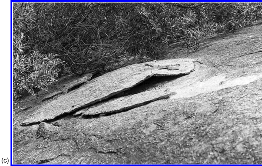
Figure 11.8. (c) Thin A-tent in granite gneiss on western midslope of Carapsee Hill, northeastern Eyre Peninsula, South Australia.
