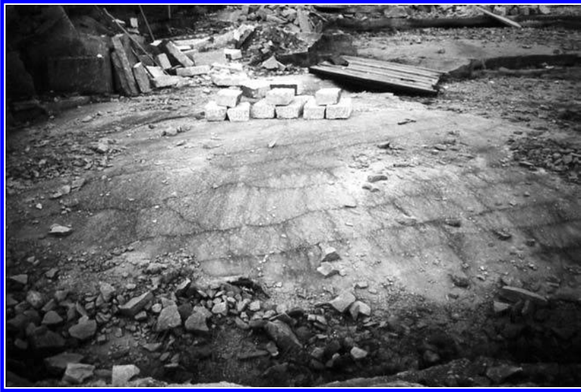
Figure 11.27. Polygonal cracking over the outer shell of a dome in Mariz Quarry, Galicia.
