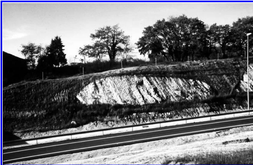
Figure 6.11. (a) Schematic development of void masses of fresh rock set in foliated matrix as a result of shearing along low-planes of dislocation. (b) Highway cutting near Lugo, Galicia, northwestern Spain, showing two large corestones set in shattered and weathered matrix corresponding to a major plane of subhorizontal shearing.
