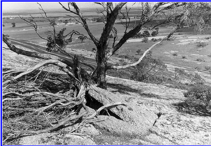
Figure 3.4. Disruption of granite slabs by tree roots, Wudinna Hill, northwestern Eyre Peninsula, South Australia.
