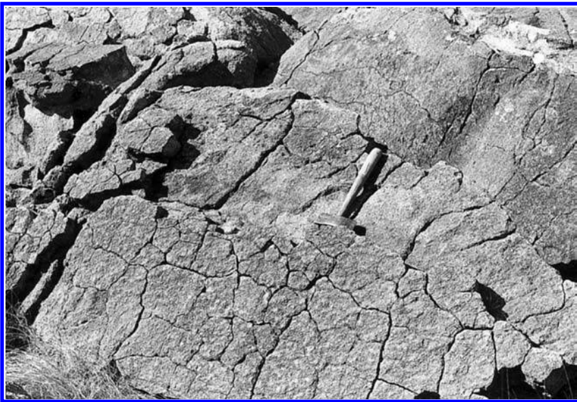
Figure 11.28. Polygonal cracking on several layers at The Granites, Mt Magnet, Western Australia.
