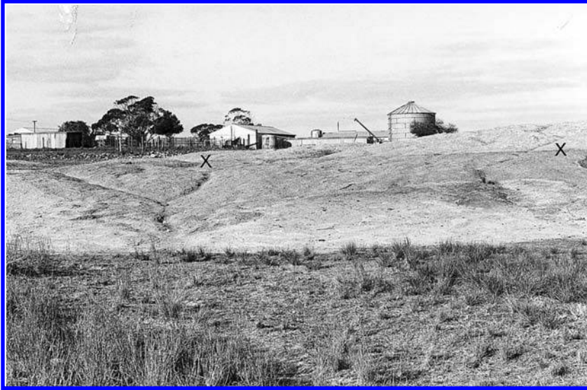
Figure 9.17. Reservoir at Dumonte Rock, near Wudinna, Eyre Peninsula, South Australia, showing gutters draining naturally exposed surface and continuing along exposed weathering front (below X–X). Some even converge in the natural subsurface.
