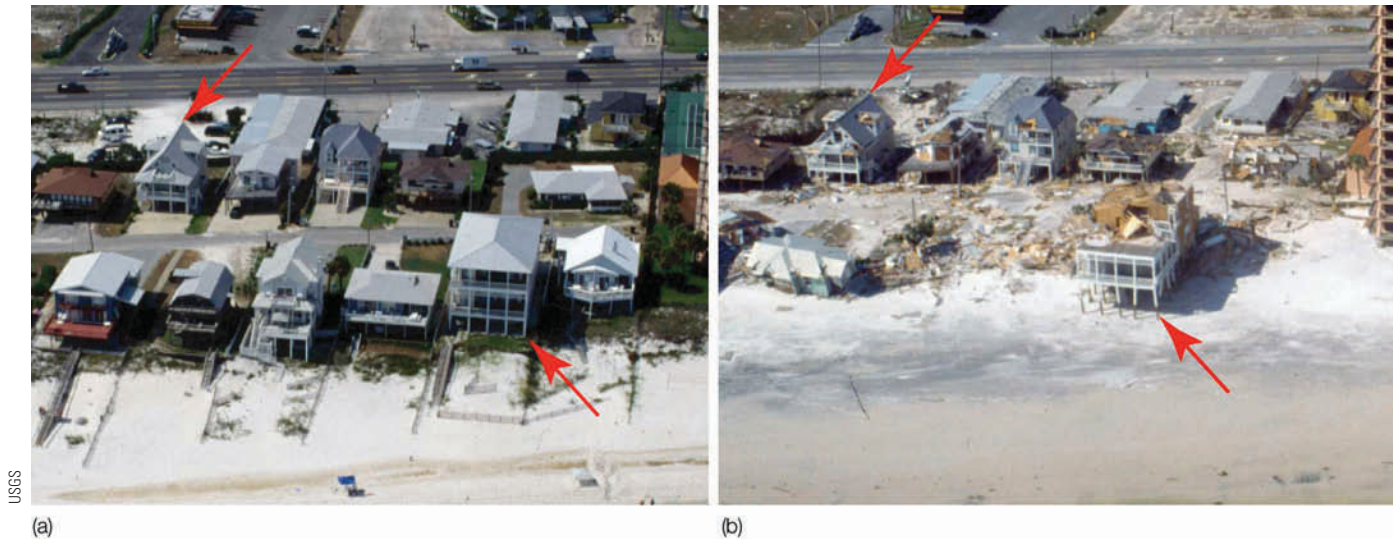
FIGURE 11.21 Beach homes along the Gulf Coast at Orange Beach, Alabama (a) before, and (b) after Hurricane Ivan made landfall during September, 2004. (Red arrows are for reference.)
