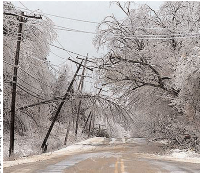
■ FIGURE 1.16 Ice storm near Oswego, New York, caused utility poles and power lines to be weighed down, forcing road closure.
