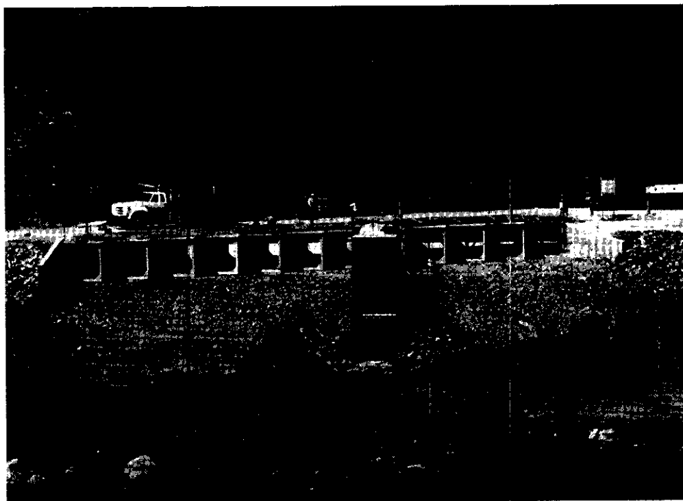
Figure 17.2.20 Culvert spillway under construction in northern New Mexico (Photograph by L. W. Mays).
