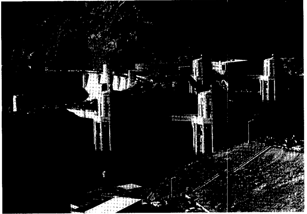
Figure 17.2.13 Hoover Dam on the Colorado River. (b) Intake towers to 30 ft diameter steel penstocks (Photographs by L. W. Mays).
