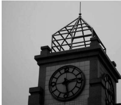
Figure 4-1. The Stopped Clock at Hanwan Town
