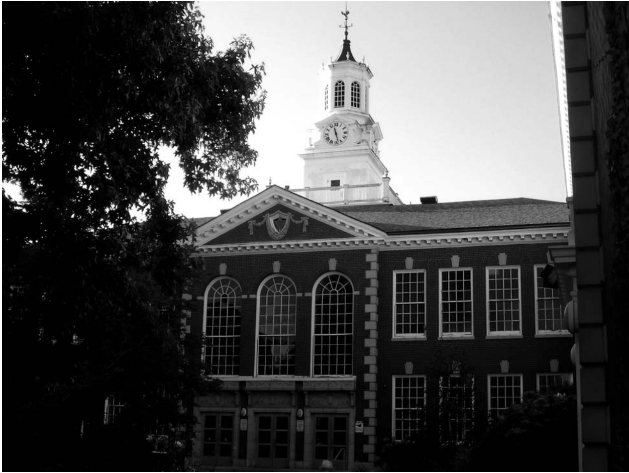
Figure 3-3. Portland, Oregon's Franklin High School is one of three URM high schools that will be rebuilt thanks to a school bond approved by Portland voters in November 2012
