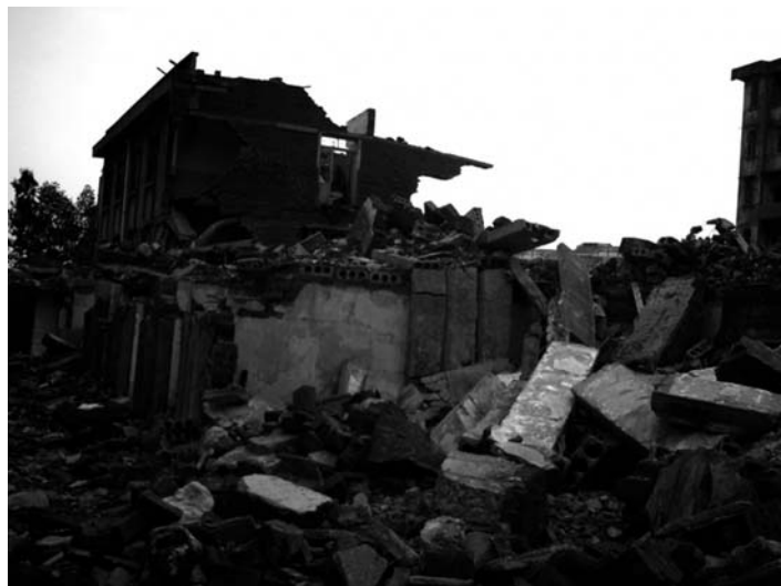
Figure 4-4. Collapsed URM Hospital building structures
