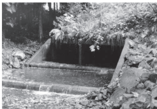
Fig. 1-22. Photos show barrier to fish passage through bridge culvert before (top) and after (bottom) construction of log step weirs and gravel-bottom pool and step approach aprons on Little Salmon Creek, Toledo, Washington. View is upstream. Photographs by J. Johnson.
