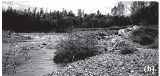
Fig. 23-3. (a) Saeltzer Dam on the Clear Creek, California, removed in 2000, courtesy of Geoff Fricker; and (b) former impoundment area of the Saeltzer Dam, photo taken in 2003, courtesy of Peter Miller. No head cut was observed in the reservoir deposit following the removal of the Saeltzer Dam (Matt Brown and Jess Newton, personal communication, 2003).
