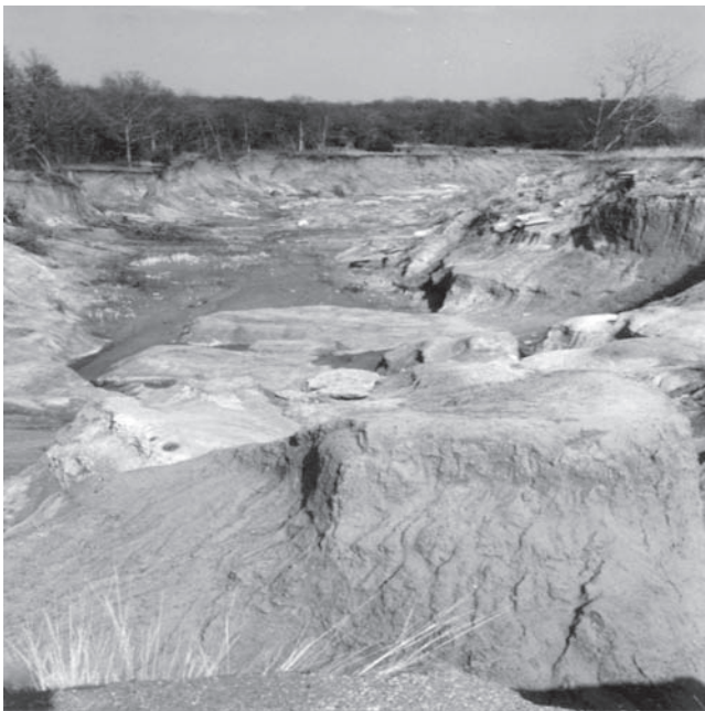
Fig. 1-8. Severe erosion and headcutting in former natural channel below Grapevine Dam Spillway, Texas, resulting mainly from greatly increased maximum outflows from collected urban flood runoff. Photograph by C. R. Neill.
