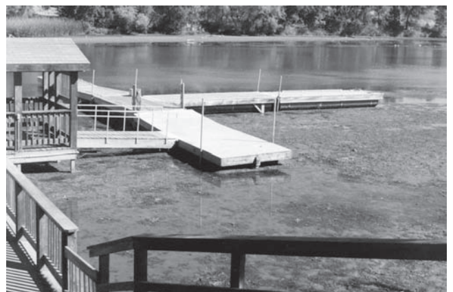
Fig. 1-18. Lake Solano, California: example of significant reservoir siltation. Photograph by R. C. MacArthur.
