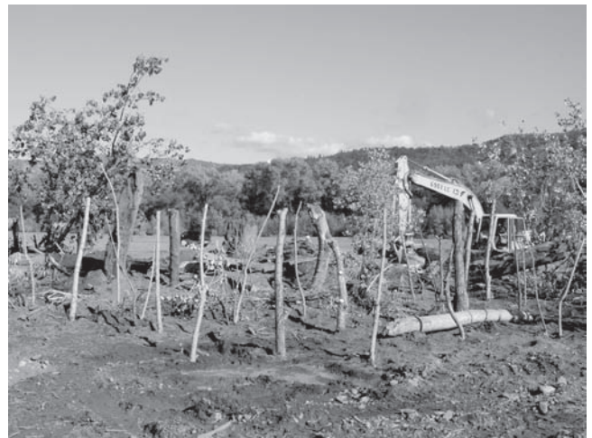
Fig. 1-20. Planting vegetation to reduce flow velocities, capture debris, and encourage sediment deposition to provide protection along an eroding bank of the Russian River, California. Photograph by D. Ripple.
