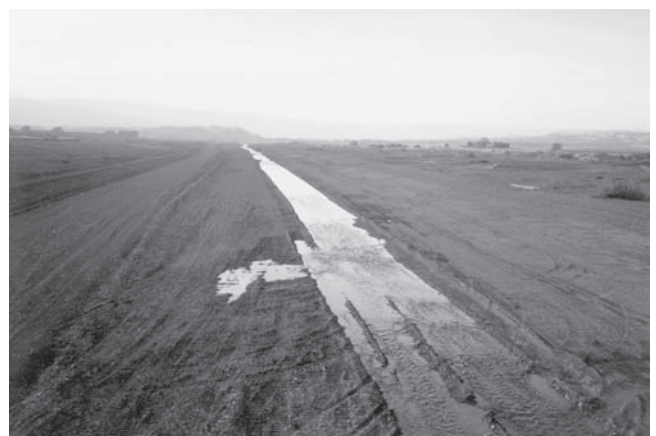
Fig. 1-7. Natural (top photo) and mined (bottom photo) reaches of Cache Creek, California, in 1986. Historically, excessive aggregate mining significantly altered the channel's morphology, causing channel degradation and thalweg lowering (incision). Implementation of comprehensive mining regulations in 1996 has improved conditions. Photographs by R. C. MacArthur.
