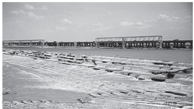
Fig. 11-5. An undermined and failed concrete check dam designed to control degradation on a Taiwanese river (looking upstream).
