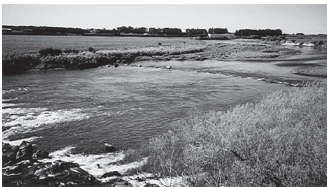
Fig. 11-4. The rock weir and rock mattresses protecting the Oreti River road bridge (looking downstream).
