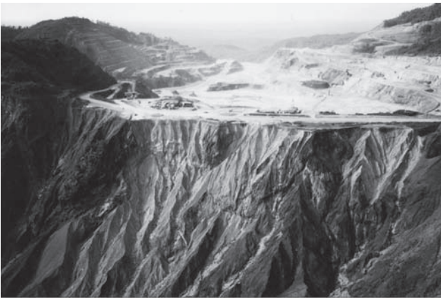
Fig. 1-15. Copper and gold mine on Mount Fubilan in Papua New Guinea. Since the mid-1980s, the mine has discharged 70 million tons per year of contaminated rock and tailings into the Ok Tedi and Fly rivers. Photograph by B. Hall.
