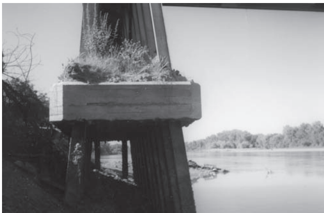
Fig. 1-9. 1995 photo of bed scour and bank erosion under Highway 162 Bridge on Sacramento River, California. Long lengths of formerly buried piles are exposed by bank recession associated with toe scour. Photograph by R. C. MacArthur.
