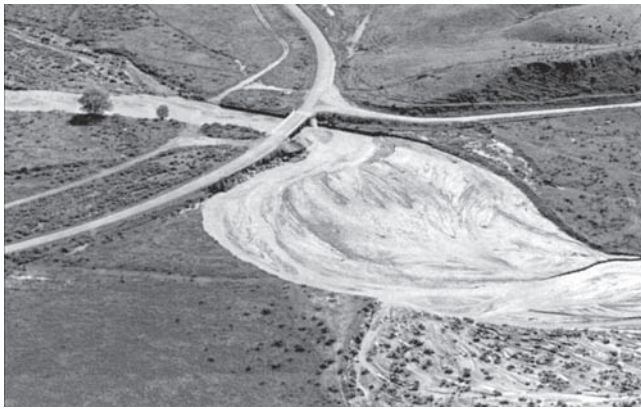
Fig. 1-5. Jacalitos Creek, California: the creek is attempting to outflank a highway bridge because the narrow bridge constriction and approach embankment prevent natural down-valley migration of meanders. Flow is from right to left. Photograph by V. J. Galay.
