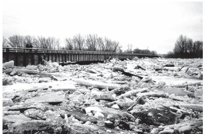
Fig. 13-13. Ice jam at a bridge across the Iowa River, Iowa.
