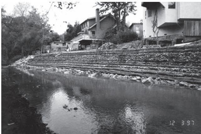
Fig. 1-19. Bank protection works in urban setting consisting of riprap toe armor and bank revetment materials with horizontal rows of willow pole plantings, as installed on Soquel Creek, California. Photograph by S. Seville.
