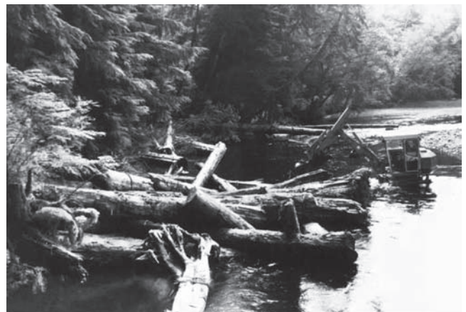
Fig. 1-21. Bioengineered logjams being installed to protect eroding river banks, to increase habitat complexity, and to provide deep pools for fish on the Mahatta River, British Columbia, Canada. Photograph by B. Walsh.
