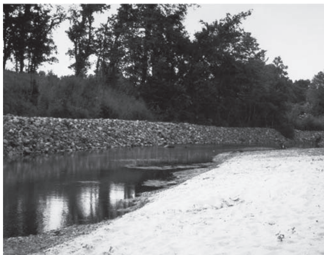
Fig. B-1. Riprap protection on lower bank only. Photo by author.
