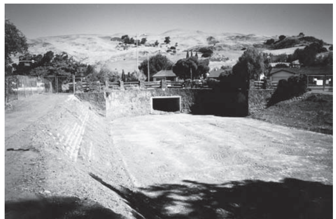
Fig. 1-13. Box culvert and sediment detention basin on urbanized reach of Upper Berryessa Creek in Milpitas, California. Basin filled with gravel is shown in top photo and after cleaning in bottom photo. View is upstream. Photographs by R. C. MacArthur.
