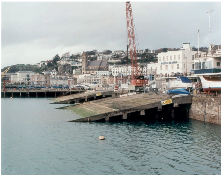
Fig. 36 The slipways at Torquay (Torbay). Photo: English Heritage (AA012294)
