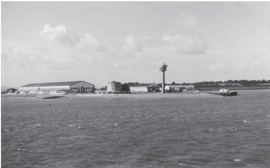
Fig. 6 Calshot Castle ( centre ) and the flying boat hangars (to its left and right ), now managed through scheduling and listing respectively. Photo: author
