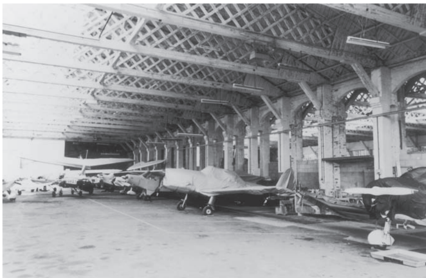
Fig. 30 First World War hangars at Old Sarum (Wiltshire), still used for their original purpose. Photo: author
