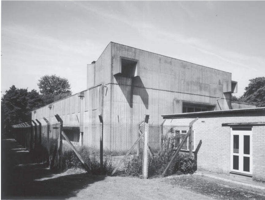
Fig. 3 Exterior of the Regional Government Headquarters, Brooklands Avenue, Cambridge (UK). Photo: Crown Copyright NMR (AA99/01972)
