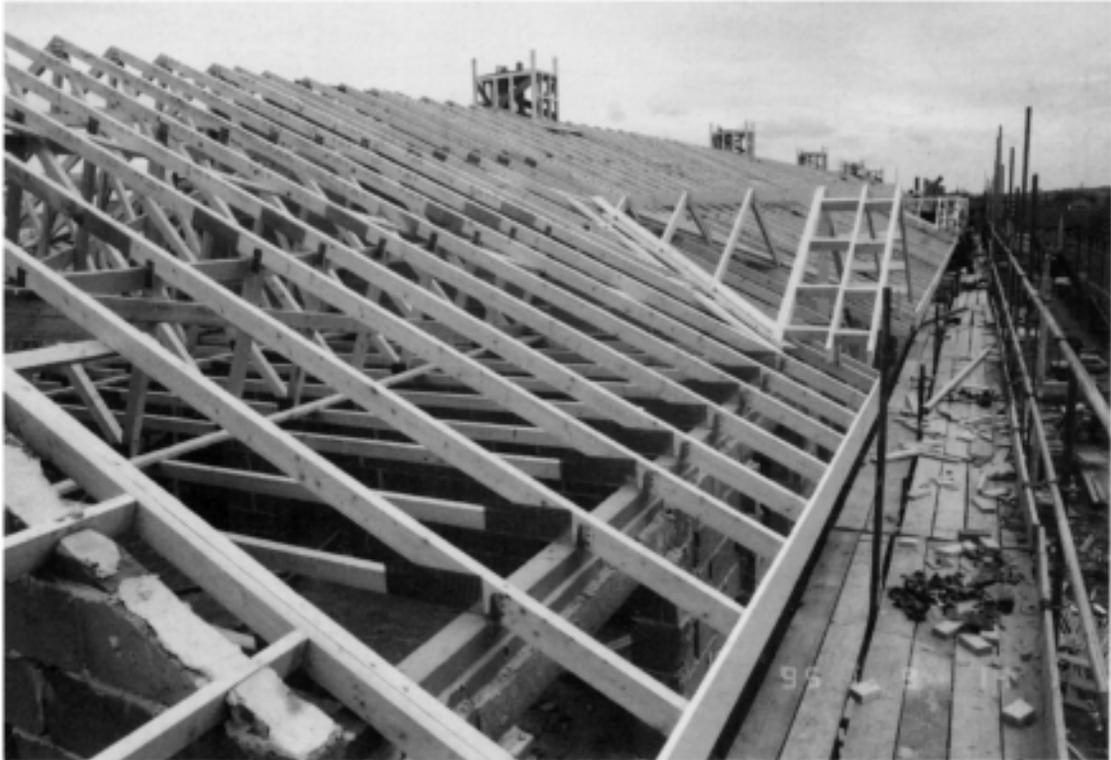
**Plate 6.4 King's Bridge Court, pitched roof during construction**
