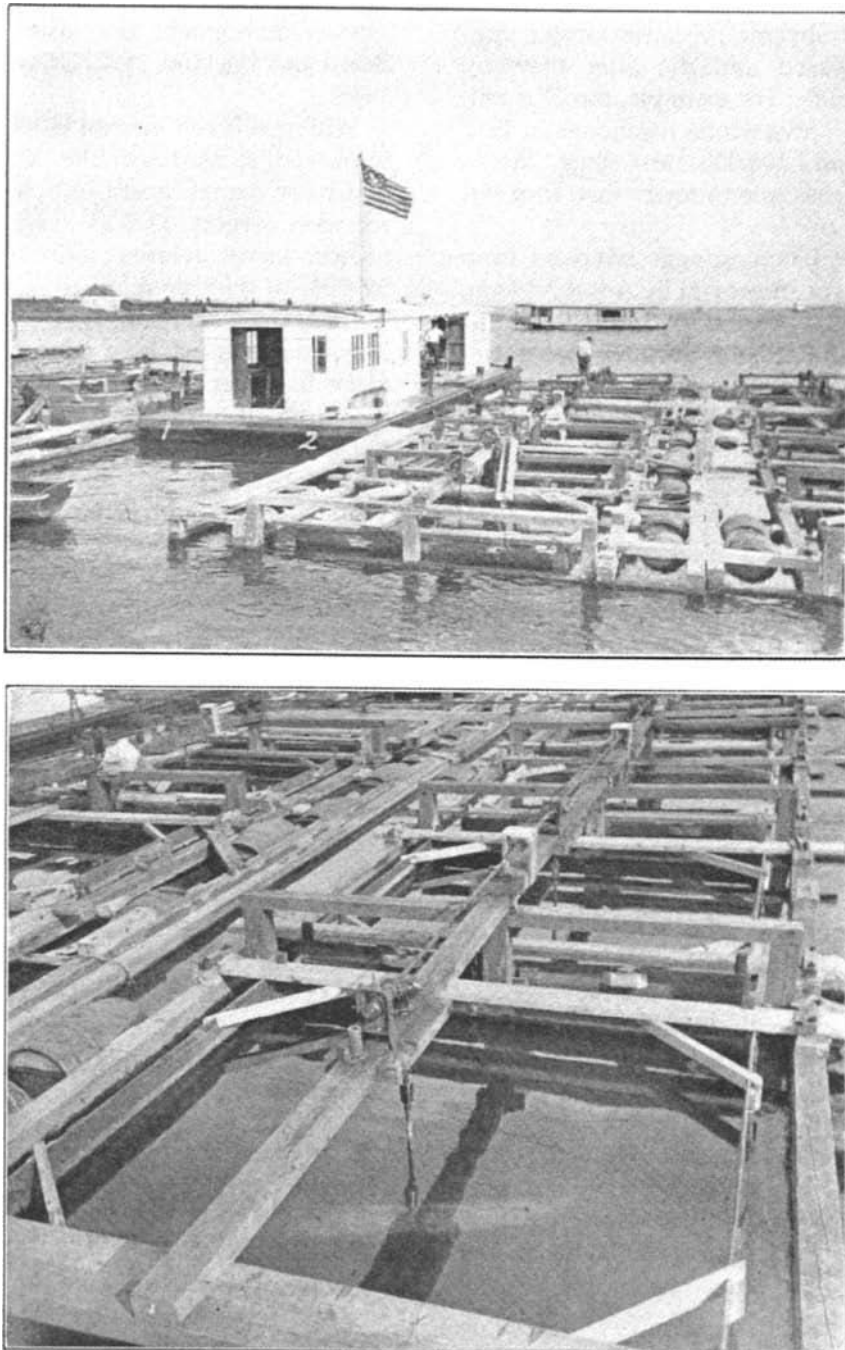
FIGURE 1 The floating laboratory of the Rhode Island Commission of Inland Fisheries at Wickford, Rhode Island. General view of a house boat with floats attached (top). The arrangement of the rearing cars, alleyways, and flotation barrels is visible on the right. Rearing cars are shown, with drive shaft and gears (bottom). The propeller is visible, submerged in the first car. (From Mead, 1908.)
