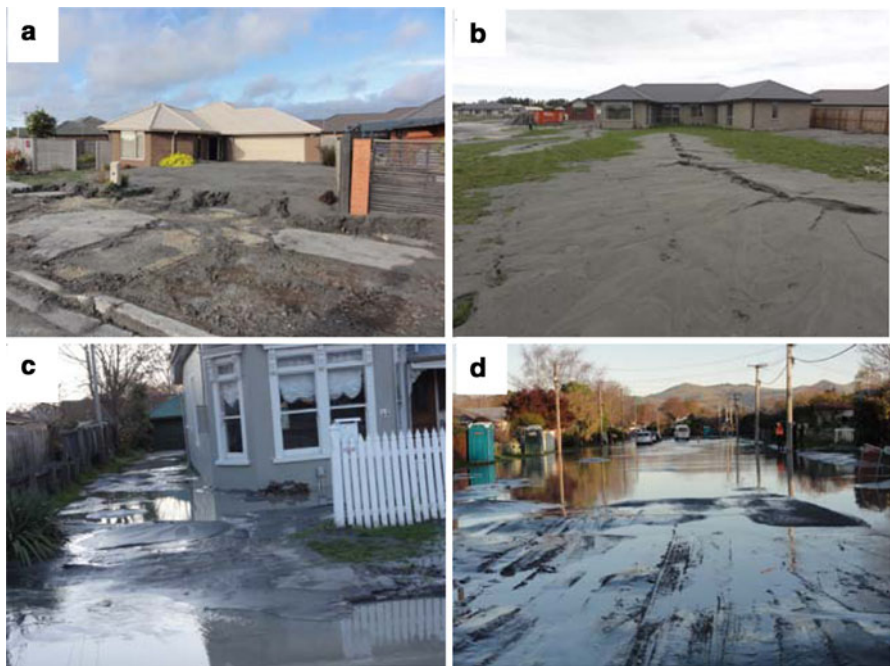
Fig. 1.10 Severe liquefaction in residential areas (suburbs along Avon River in the abandoned “red zone”)
