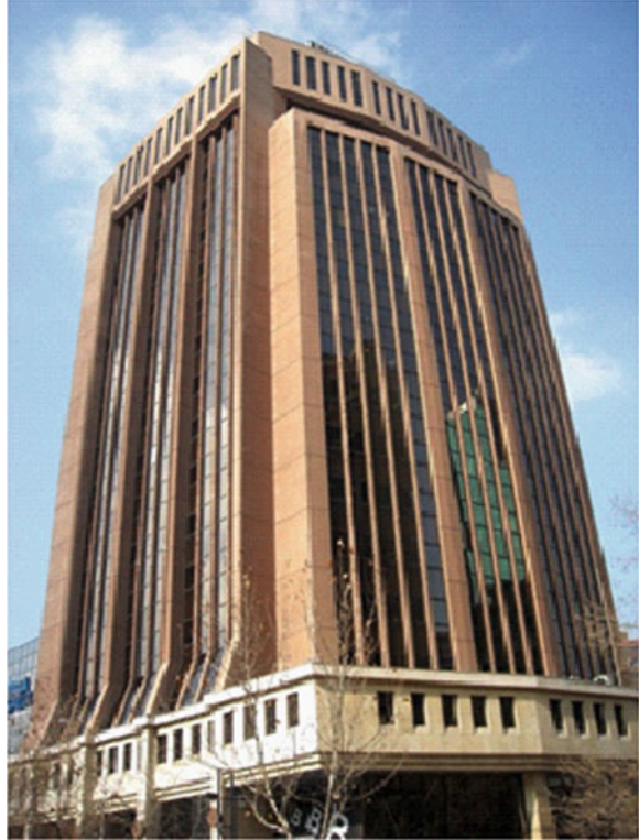
Fig. 8.14 General view of the Chilean Construction Chamber Building
