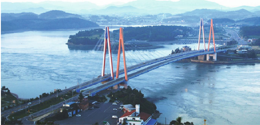
Fig. 2.38 Densely instrumented cable-stayed 2nd Jindo Bridge in South Korea uses wireless sensors (Photo courtesy of B. Spence, 2011)
