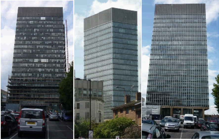
Fig. 6.1 Arts tower during ( left ) and after ( right ) retrofit
