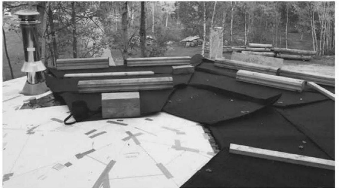
Fig. 8.6 (below): Trapezoidal sheets of Enkadrain® 3615R composite drainage are placed over the plastic, with the filtration mat uppermost. No, we haven't forgotten the plastic sheet. You can see it poking out here and there. A large centerpiece of plastic will be tucked under the Enkadrain® before it is covered with earth. Heavy wooden blocks keep everything in place until the earth goes on.
