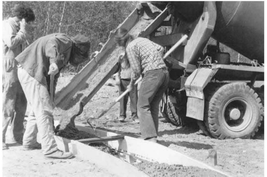
Fig. 3.22: Pouring the footings at Earthwood.
