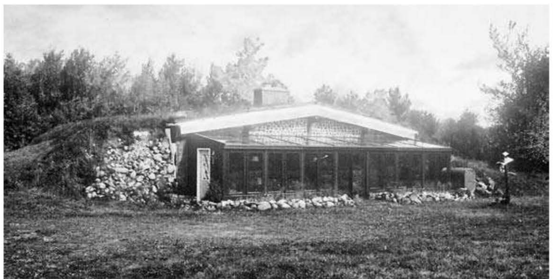
Fig. 2.2: Richard Guay's 40 × 40' Log End Cave, during construction. Fig. 2.3: Richard and Lisa Guay's completed earth-sheltered home in Champlain, New York. The solar room addition was paid for with some of Lisa's winnings as a five-time Jeopardy champion.
