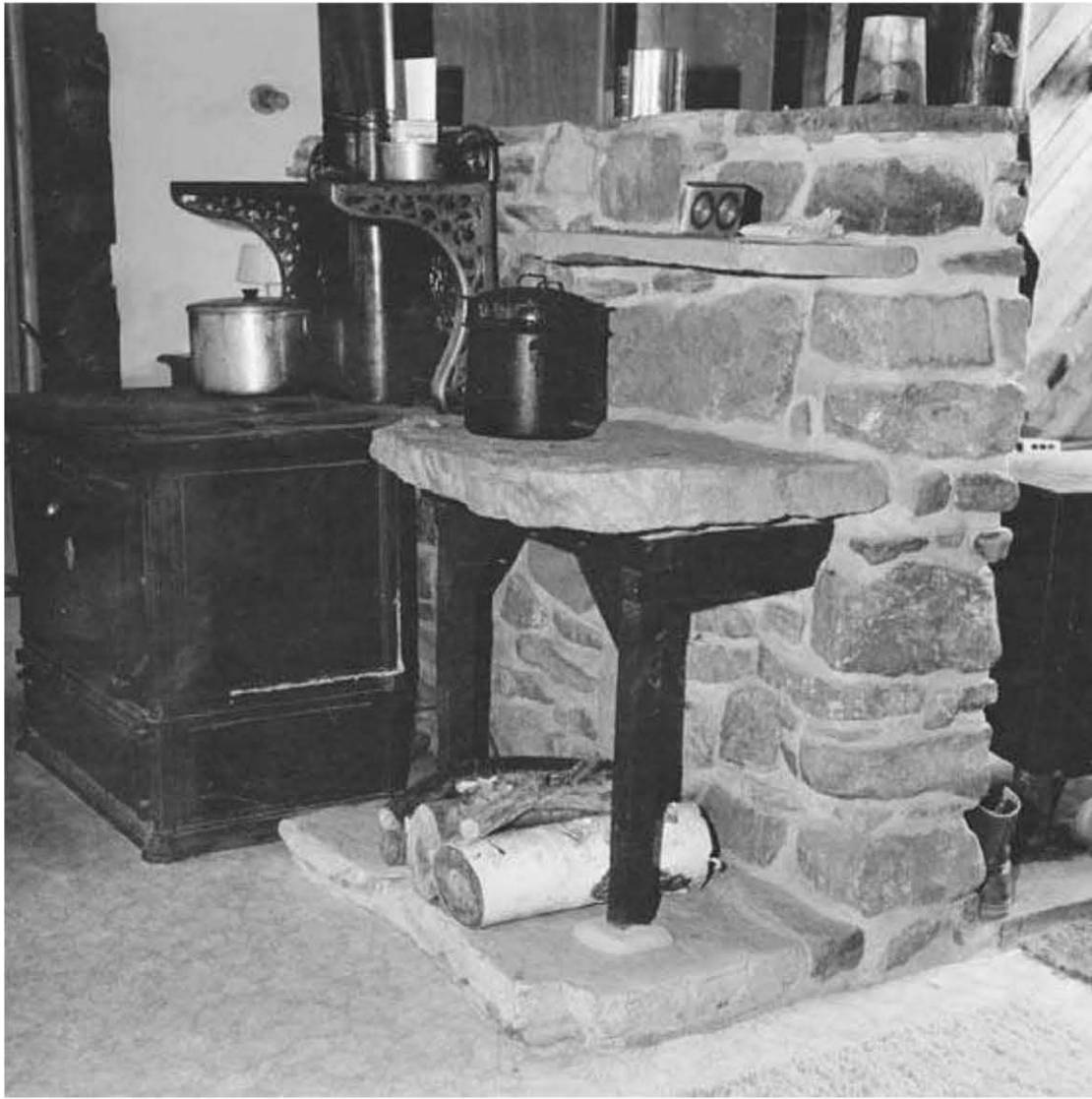
Fig. 10.2: The three-ton room divider at Log End Cave helped the home maintain a steady temperature.
