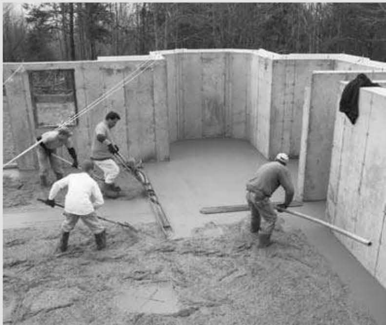
Fig. 4.15: One man operates the power screed while another bullfloats right behind him.
