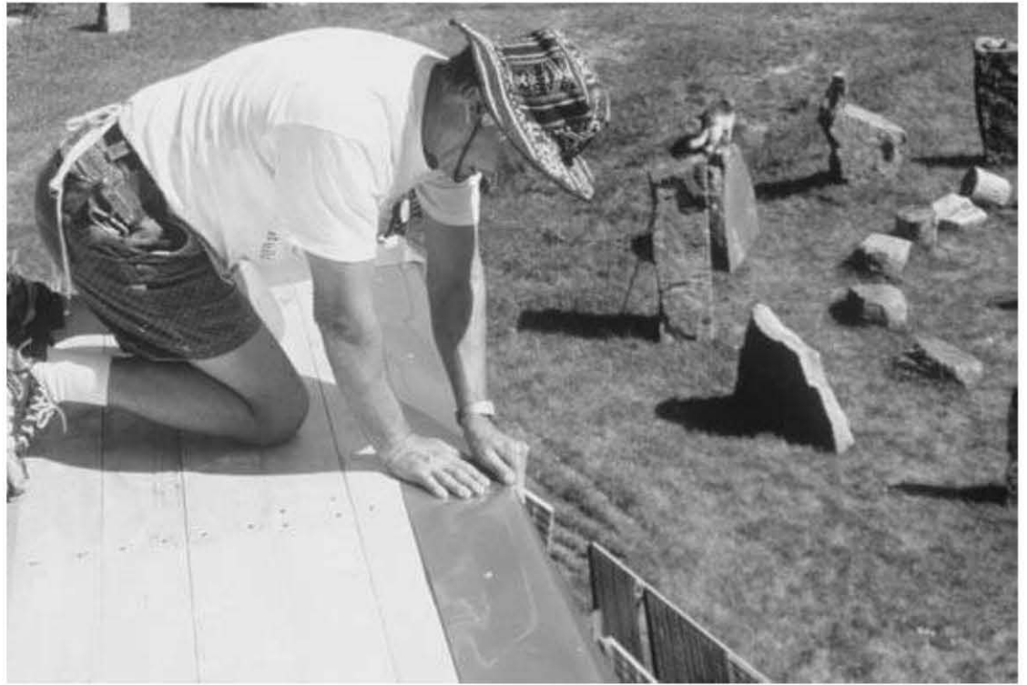
Fig. 7.4: The author bends two inches of the 7" wide flashing over the edge of the 2 × 6" deck.
