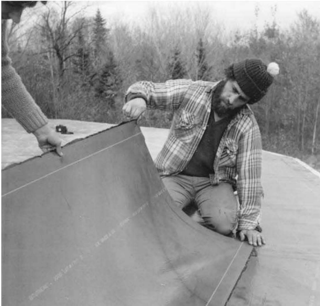
Fig. 7.8: Later, when the adjacent sheets of the same course are installed, they too should extend onto the next facet by three inches, giving a six-inch lap where two facets meet. Normally, a 3-inch lap is sufficient with Bituthene® 3000 and 4000 membranes, but you want extra protection where facets come together, pressing hard onto three inches of solid wood on each side of the crack. Apply the lower edge of the Bituthene® first, using the white line on the previous sheet as a guide.
