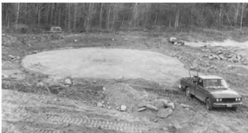
Fig. 3.6: A view of the finished sand pad at Earthwood. The pad extension near the truck is for the greenhouse.
