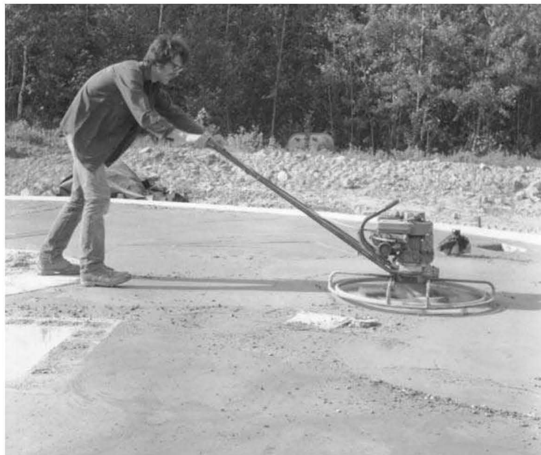
Fig. 4.17: Jonathan Cross power-trowels the slab at Earthwood.
