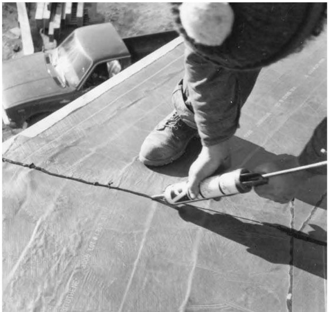
Fig. 7.9: Exposed cut edges must be sealed with a compatible caulking. After applying a bead of caulk, use a butter knife to create an edge that looks something like the factory edge. Tip: bend the last inch of a non-serrated butter knife just a little bit to make an excellent tool for this purpose.
