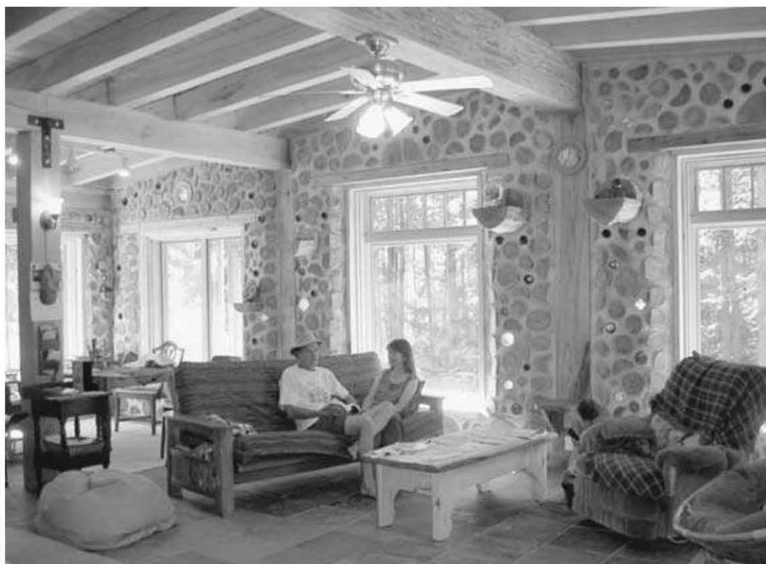
Fig. 12.3: Mark and Mary in their new home. The engineered paralam beam overhead spans 18 feet.
