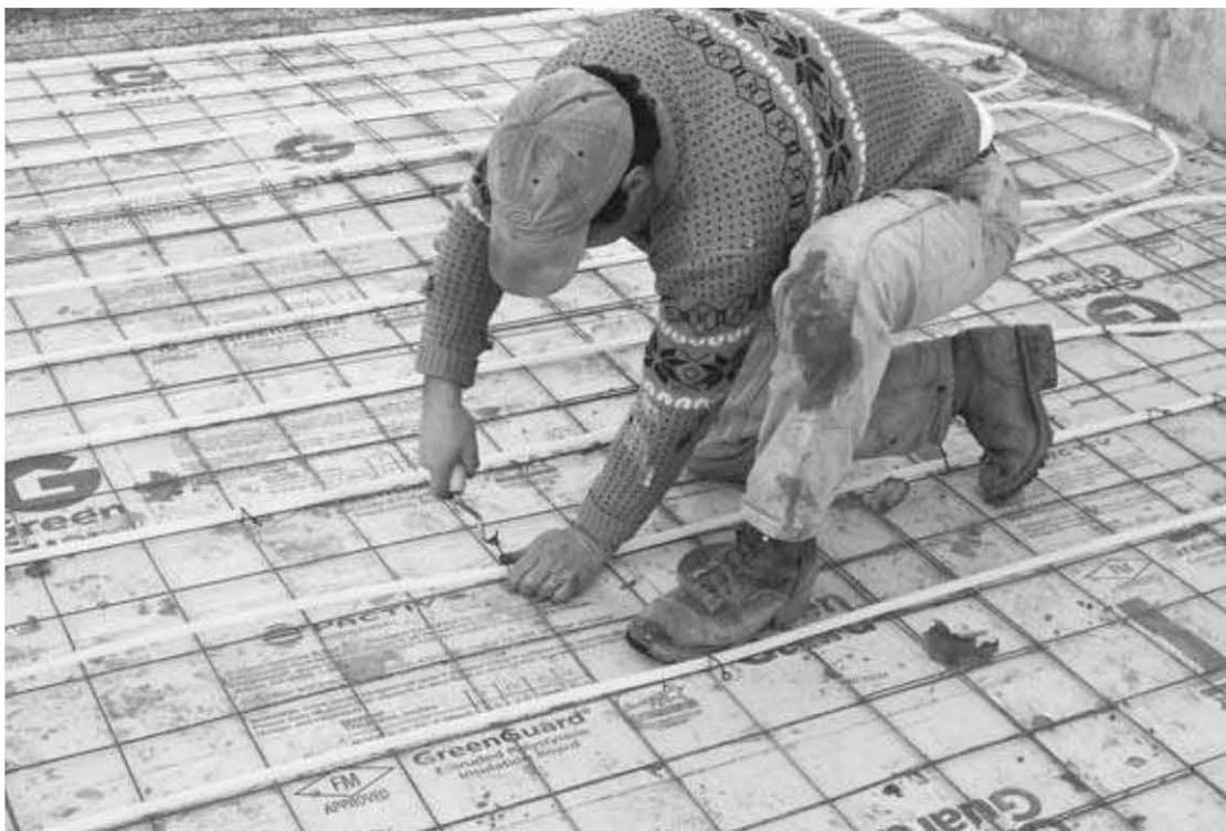
Fig. 4.6: Steve Bedard fastens his polyethylene tubing to the wire mesh with a special rotating hook made for twisting tie bands.
