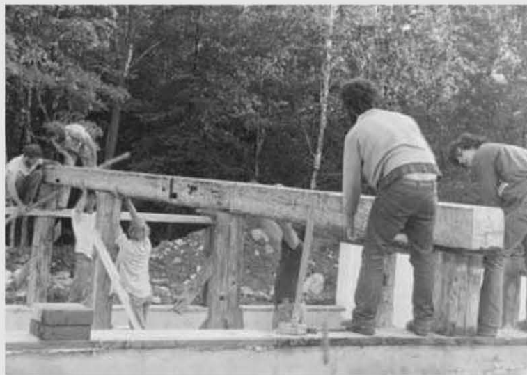
Fig. 6.5: We place the center girder on its posts, Log End Cave.
