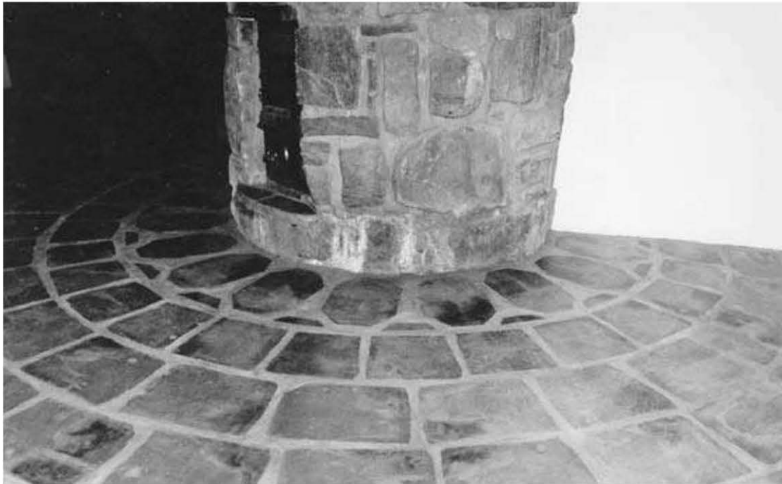
Fig. 10.5: The slate floor draws one's eye to the masonry stove at Earthwood's center.
