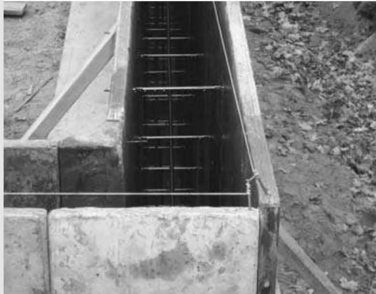
Fig. 5.2: Strong forming is critical to pouring concrete walls. Note frequent cross ties that keep the forms from spreading.
