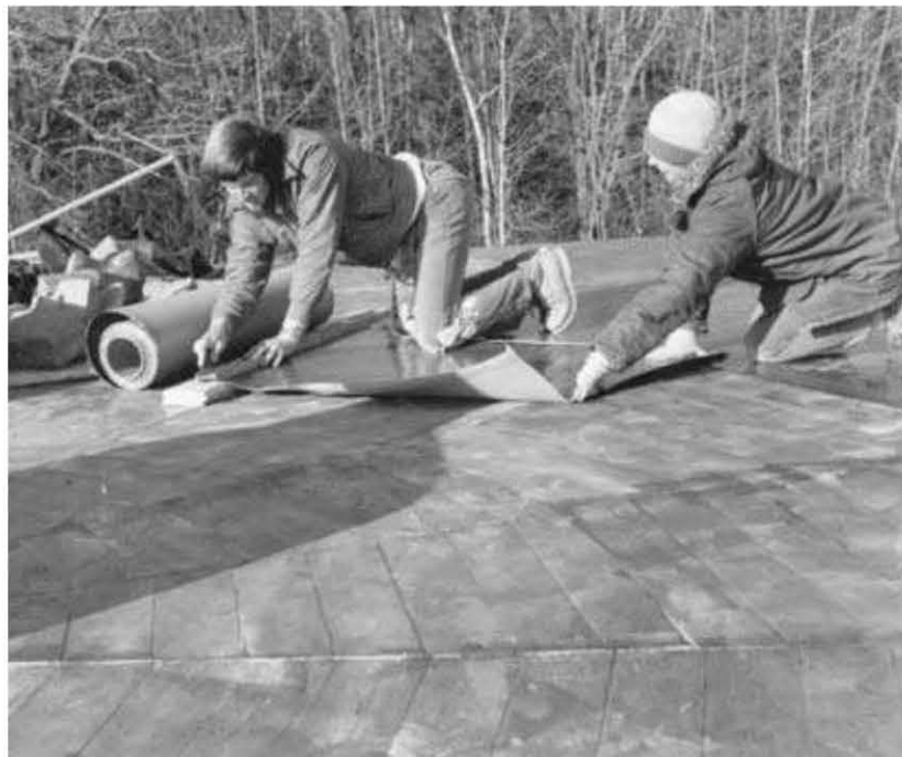
Fig. 7.7: Cut Bituthene ® with a razor knife, over a scrap board.
