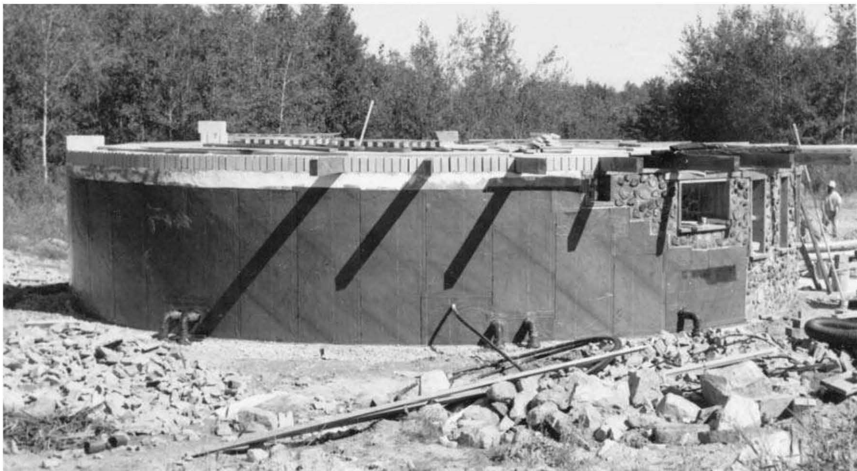
Fig. 7.3: The Bituthene ® has been applied to the lower story at Earthwood.
