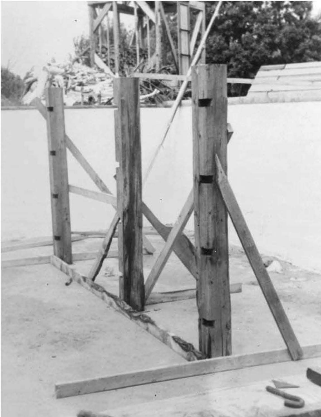
Fig. 6.4: We temporarily braced the support posts for the main girders.
