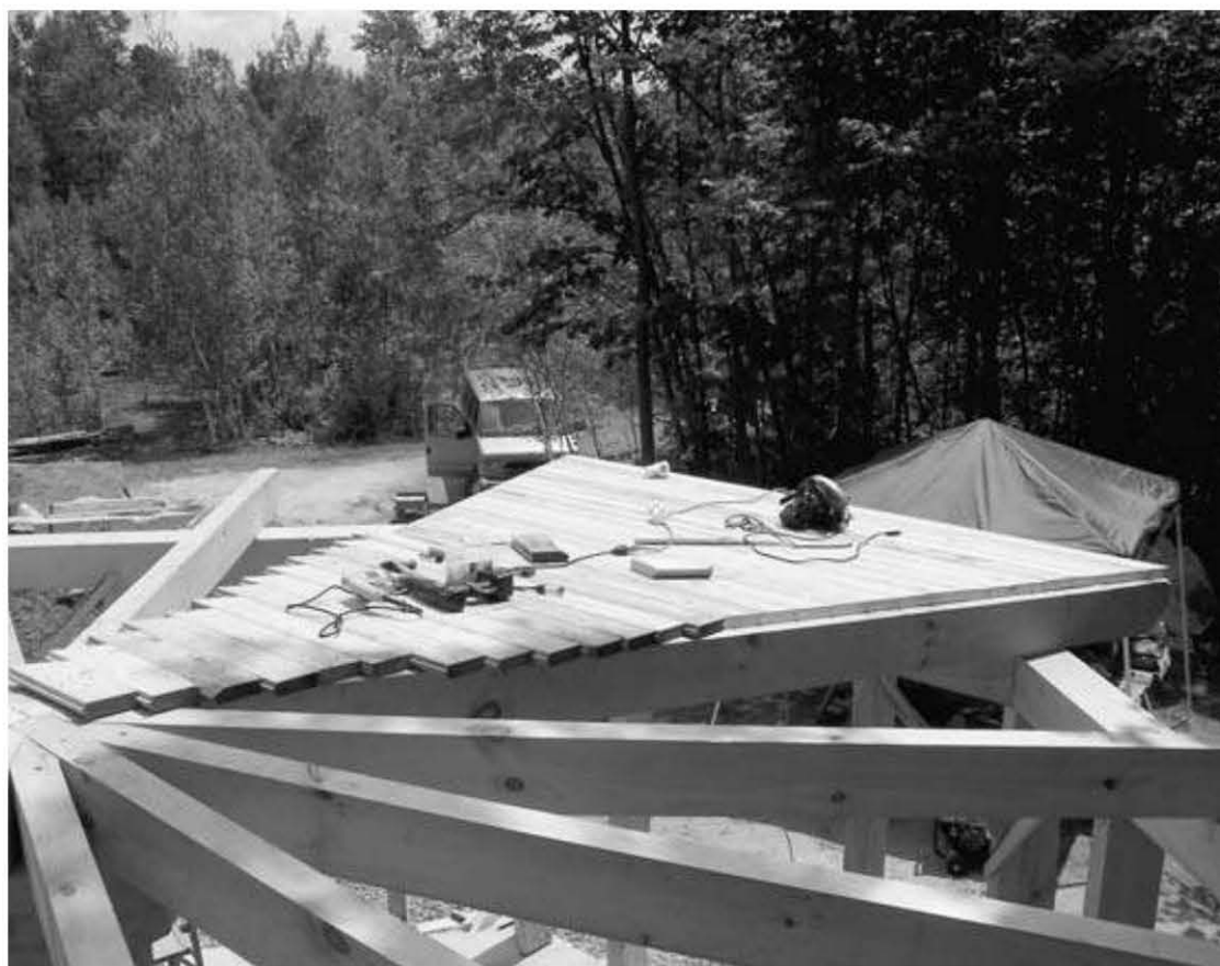
Fig. 6.19: The "waste" from the first cut is used further up the facet, so it isn't waste at all. Next, we would snap chalklines again and trim the two saw-toothed edges.
