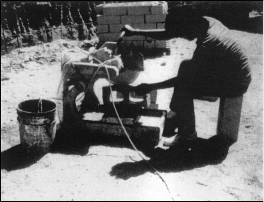
FIGURE 2.23 A mechanical cutter in use at a jobsite. (Courtesy: Author.)
