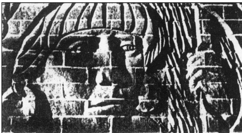
FIGURE 2.16 Sculptured brick panels at Loew's Anatole Hotel, Dallas, Texas. Beran and Shelmire, architects. Mara Smith, sculptor. (Courtesy: BIA).
