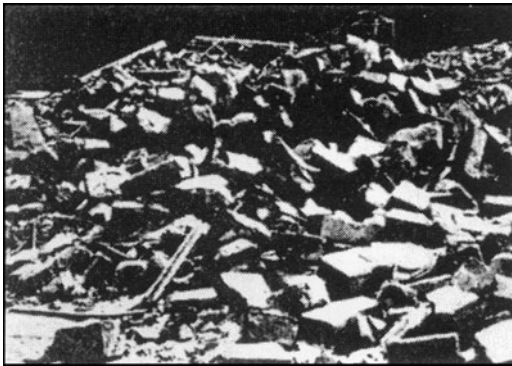
FIGURE 2.15 Brick salvaged from demolition of existing walls. (Courtesy: BIA.)
