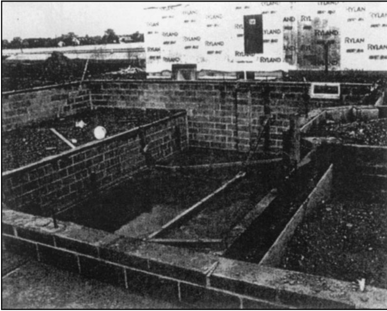
FIGURE 8.5 A subterranean wall. (Courtesy: NCMA.)
