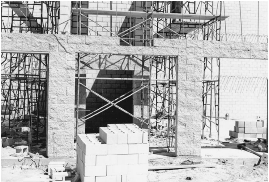
FIGURE 4.18 Concrete masonry lintels under construction. (Courtesy: Author.)
