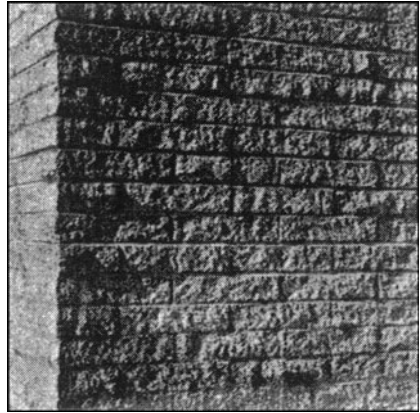
FIGURE 2.33 A wall with split-face concrete blocks. (Courtesy: PCA.)
