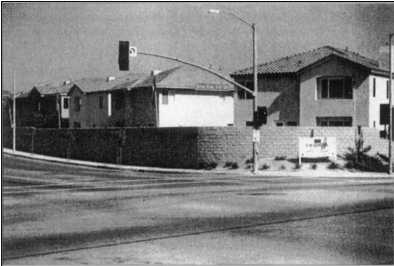
FIGURE 6.44 A typical fence wall in a residential area. (Courtesy: Author.)
