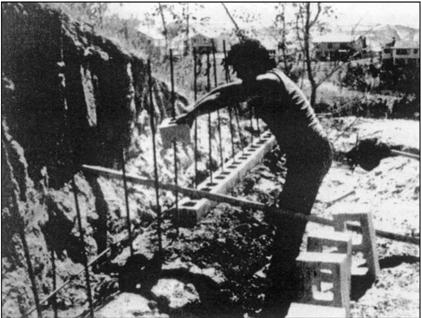
FIGURE 2.21 Threading a reinforcing bar through a hollow concrete block. (Courtesy: Author.)
