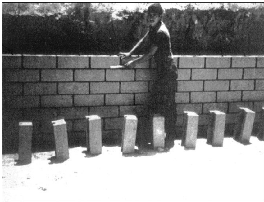
FIGURE 2.42 Tooling of masonry joints. (Courtesy: Author.)
