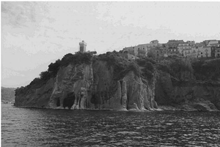
Figure 3.28 Coastal stretch near Agropoli, Italy, affected by recurrent rock-falls (from Budetta et al. (2008).
