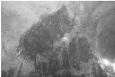
Figure A6 Moderate rockburst, drainage gallery. Figure A7 Slight rockburst, downstream spandrel.
