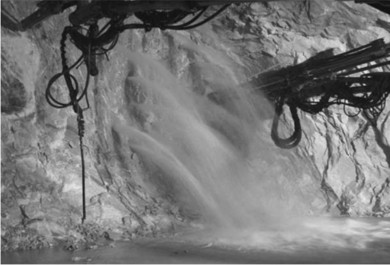
Figure 6.74 A water inrush case explored by drilling and probing (HydroChina Huadong Engineering Corporation, 2005).
