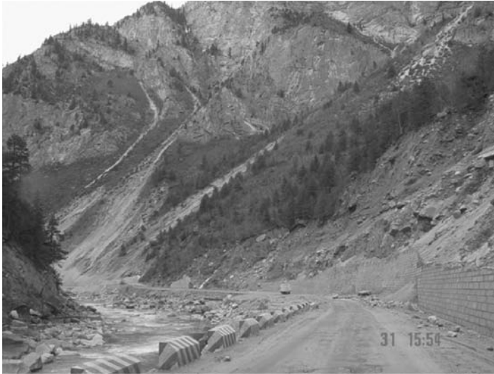
Figure 3.27 Adverse highway landslide conditions along the Sichuan–Tibet Highway (northern Yarlu-Tsangpu Grand Canyon of Tibet), from Shang et al. (2005).
