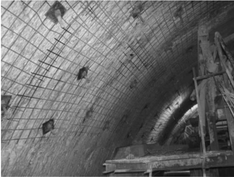
Figure 6.86 Example of support in headrace tunnel #3.
