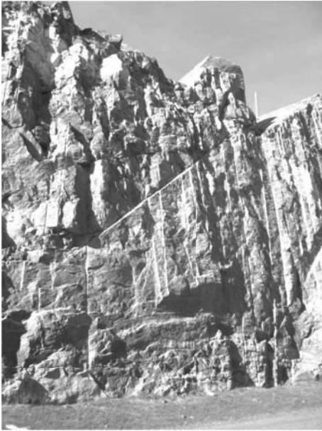
Exposure 11. Pre-split, granitic basement rockface, Finland
