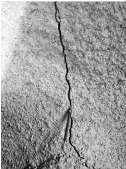
Figure 7.218 Sprayed concrete cracks at 3# bus tunnel.
