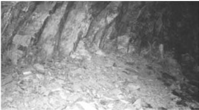
b Surrounding rock collapse
