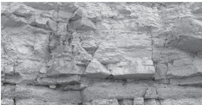
c Chalk strata with horizontal, vertical and inclined, conjugate fractures.
