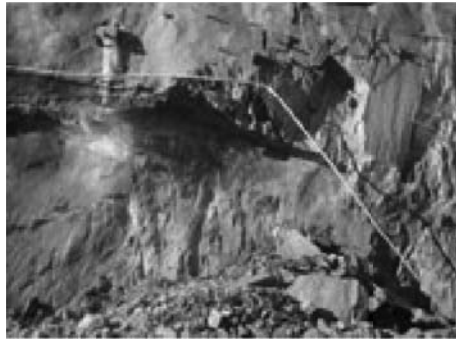
Figure A21 Collapse at a fault.
