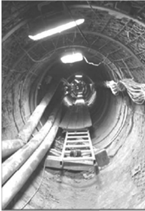
Figure 5.13 The research tunnel at the Mont Terri Underground Research Laboratory, Switzerland.
