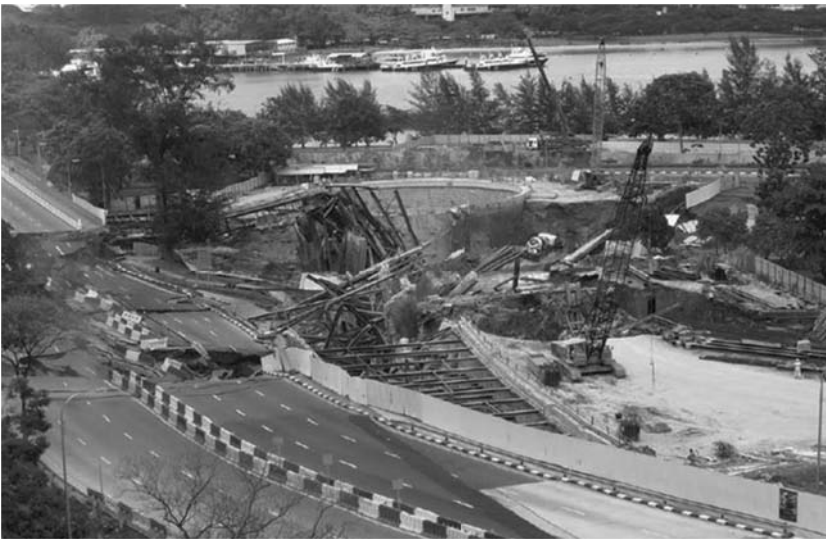
Figure 2.4 Collapse during construction of the Singapore MRT, 2004 (Government of Singapore).
