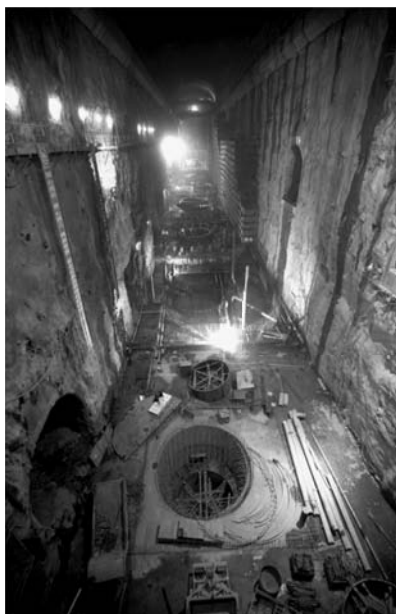
Figure 2.8 Construction of large caverns for hydropower projects.
