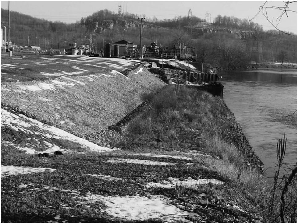
Figure 5-52. View downstream toward the intake. The river bank upstream of the intake was realigned to guide flow directly past the intake. Source: Michell et al. (2006), ASCE.
