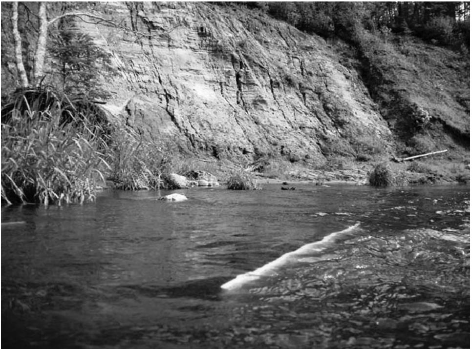
Figure 5-14. Downstream view of North Fish Creek at low flow. Submerged vanes protect the toe of the bluff. Source: Fitzpatrick et al. (2005), courtesy of U.S. Geological Survey.
