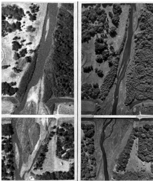
Figure 5-24. Aerial photos of the West Fork Cedar River bridge crossing (left) prior to vane installation in 1984, and (right) in 1989, five years after vane installation. Source: Odgaard and Wang (1991), ASCE.
