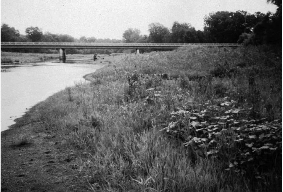
Figure 5-25. View downstream toward the Butler County (Iowa) bridge, August, 1989. Bank eroding prior to vane installation is by tree line to right in photo. Source: Odgaard and Wang (1991), ASCE.
