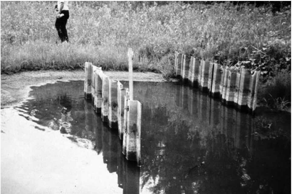
Figure 5-26. Most-upstream vane array of the West Fork Cedar River installation.
