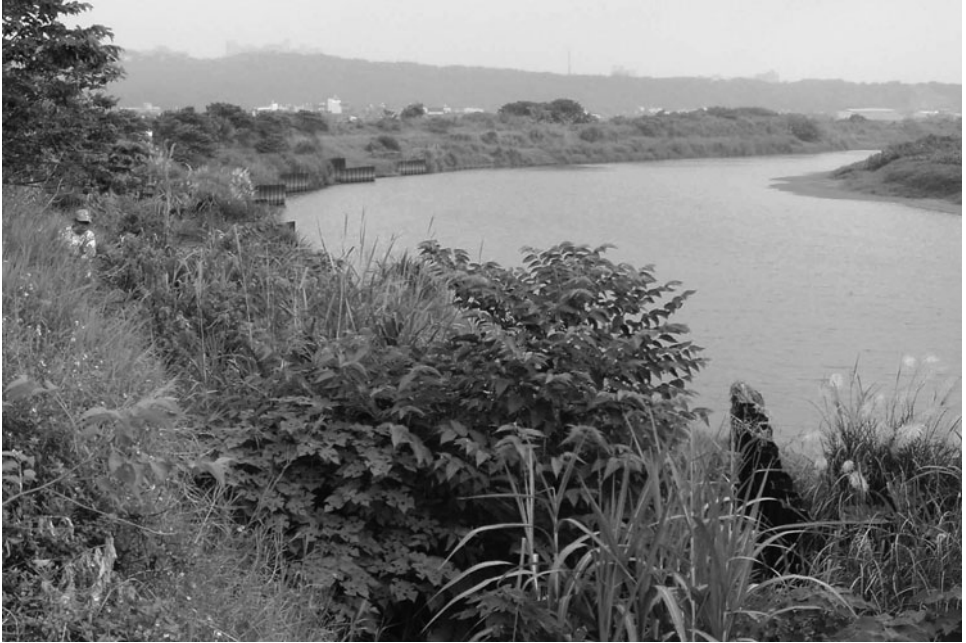
Figure 5-19. Upstream view of vane installation in the Maoerding bend, one year after installation, at extreme low flow.
