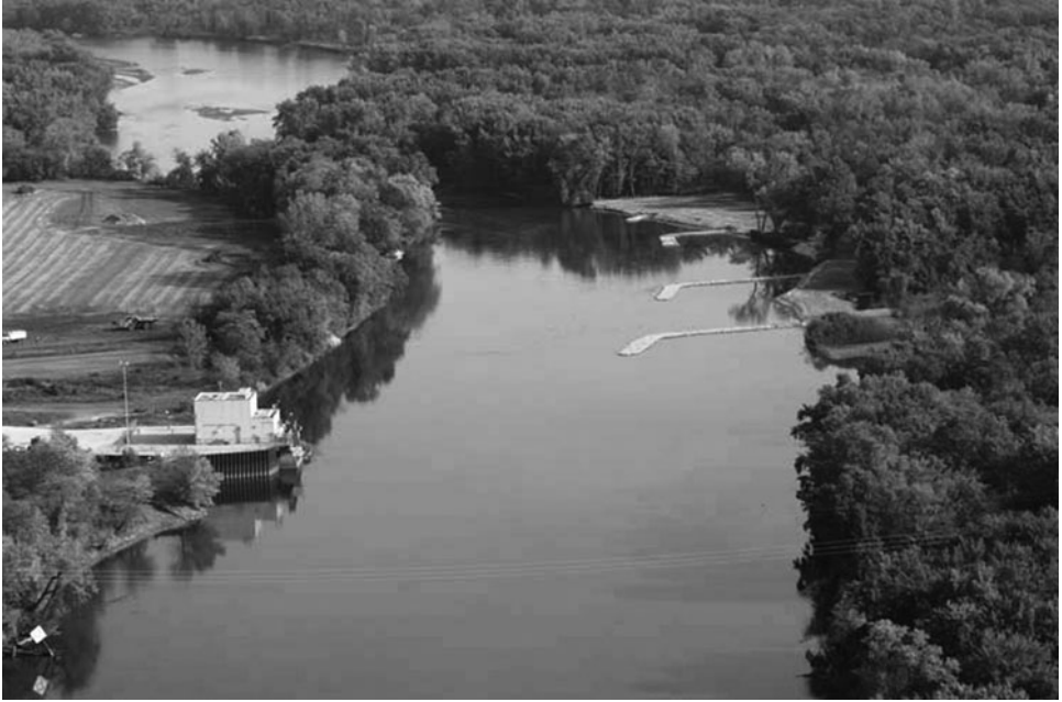
Figure 5-34. Upstream view of Cedar River at the DAEC intake structure. In 2006, four spur dikes were installed on left bank upstream from the intake. The wings of the spur dikes delineate the 1980 left bank of the river. Courtesy of Paul Collingsworth, FPL Energy Duane Arnold.
