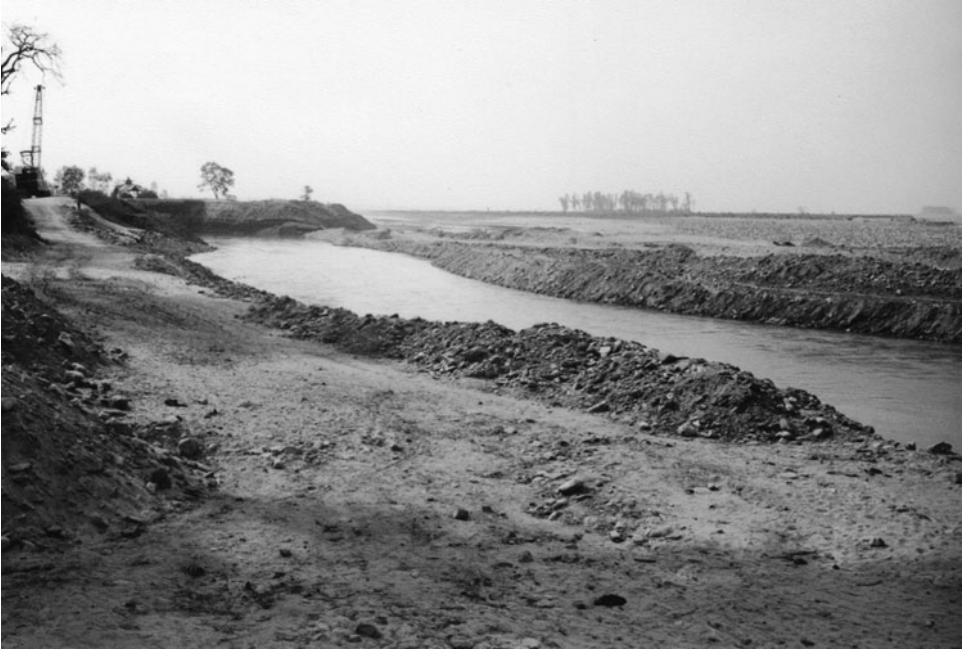
Figure 5-57. Dredging at the old intake on Kosi River. Courtesy of J. Oosterman, DHV Consulting Engineers.
