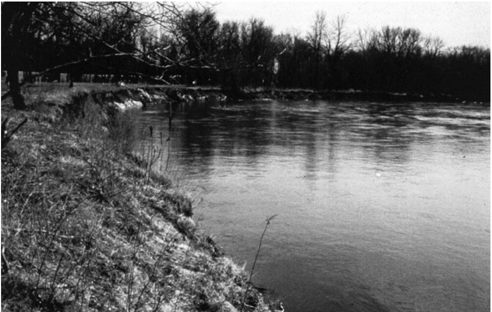
Figure 5-6. View downstream in the Wapsipinicon River, showing bank erosion along left bank. Courtesy of Robert DeWitt, River Engineering International.
