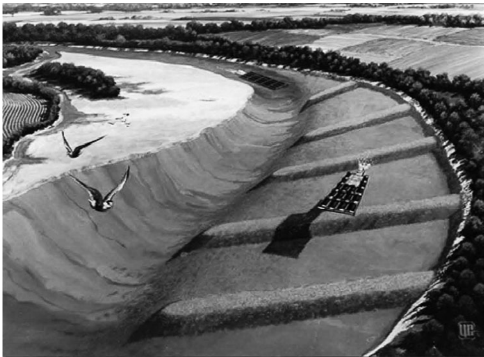
Figure 1-20. U.S. Army Corps of Engineers’s bend-way weirs. Source: U.S. Army Corps of Engineers (2008).
