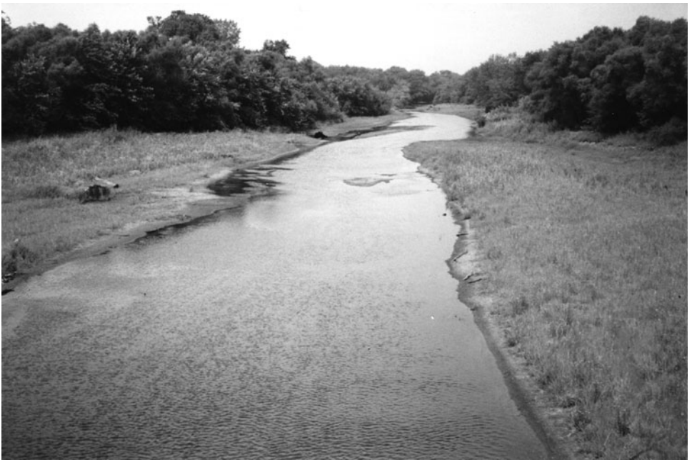
Figure 5-28. Views upstream from the bridge at low flow. Above: Old channel along right bank, now a heavily vegetated berm. Below: New channel running straight through center span of bridge.
