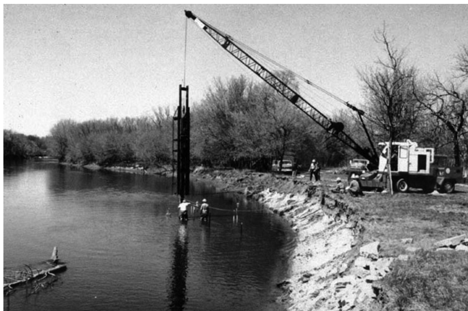
Figure 5-8. Driving of H-piles, summer, 1988. Courtesy of Robert DeWitt, River Engineering International.
