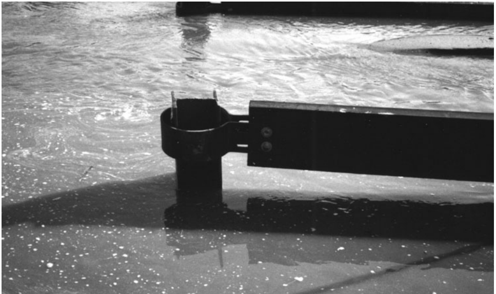
Figure 5-3. Plank with straps being lowered in place between piles.
