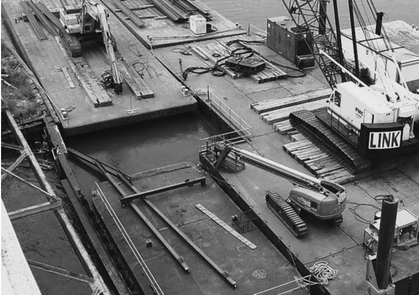
Figure 6-1. Vane installation at Cooper Station, Missouri River. The photo shows a barge-mounted guide for vane alignment near the face of the intake (left). Flow is from top left. Courtesy of Rhoël M. Tierra, Nebraska Public Power District.
