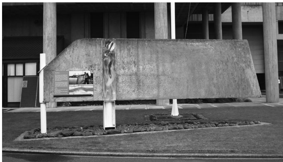
Figure 6-10. Vane display at Huntly Power Station, New Zealand, showing details of nose pipe and main H-pile with pipe connection. Source: Electricity Corporation of New Zealand (1993), with permission from Genesis Energy.
