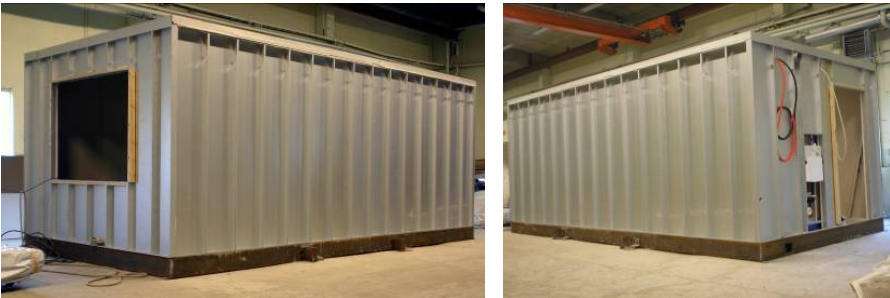
Figure 8.3 – Cassettes – Prototype for economic hotels – PARTAB – Sweden
