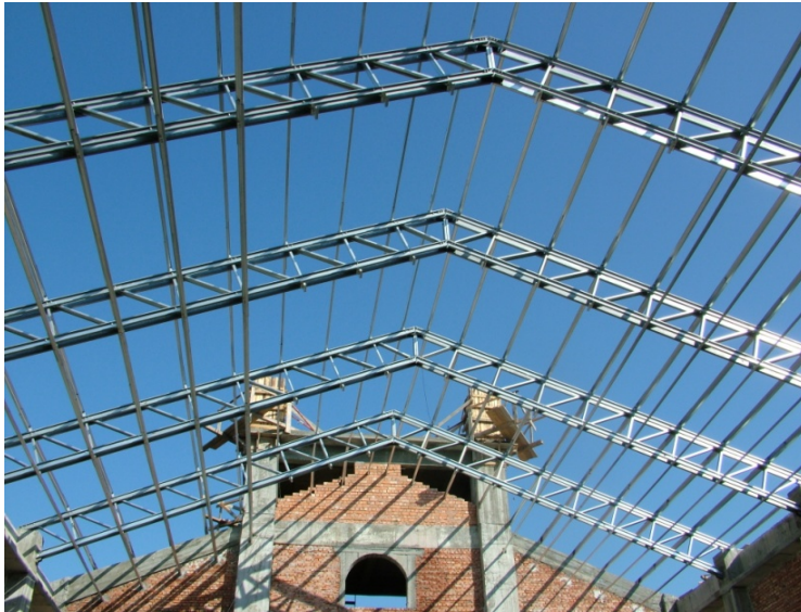
Figure 1.30 – Roof truss using C bolted sections (Constanta, Romania)
