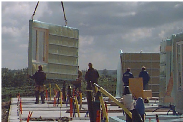
Figure 1.24 – Wall stud panels made of cold-formed steel sections
