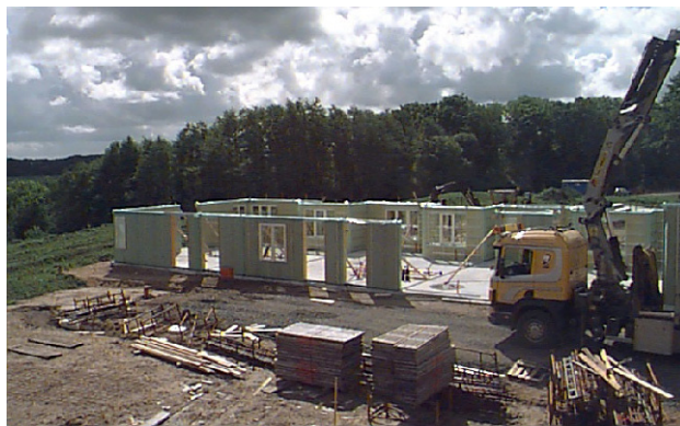
Figure 1.25 – Installing of prefabricated units
