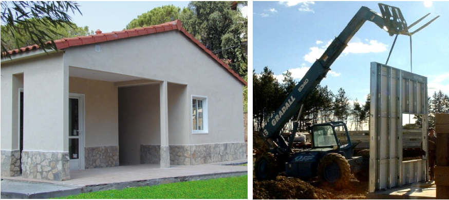
Figure 8.2 – Panellised construction – Spain
