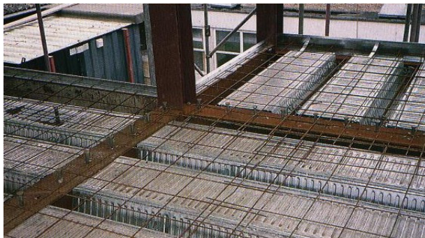
a) Decking structure and re-bar for a composite concrete steel structure
