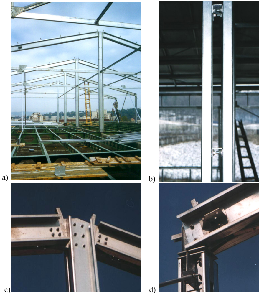
Figure 1.33 – Pitched roof portal frame made by built-up sections (back-to-back C bolted connected by stitches, Dubina et al , 2001b): a) general view; b) built-up column; c) joint detailing for ridge; d) joint detailing for eaves
