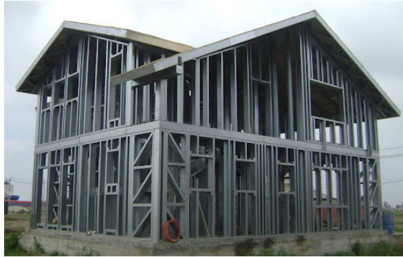
Figure 1.26 – Wall stud housing system with prefabricated cold-formed steel wall panels
