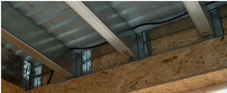
Figure 8.66 – Floor framing: Detail B
