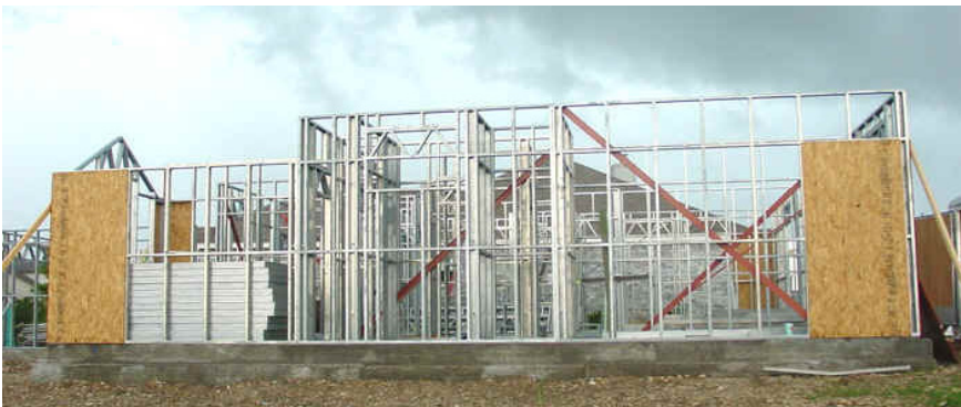
Figure 8.20 – Phase IV: Vertical structural elements of the first floor are completed
