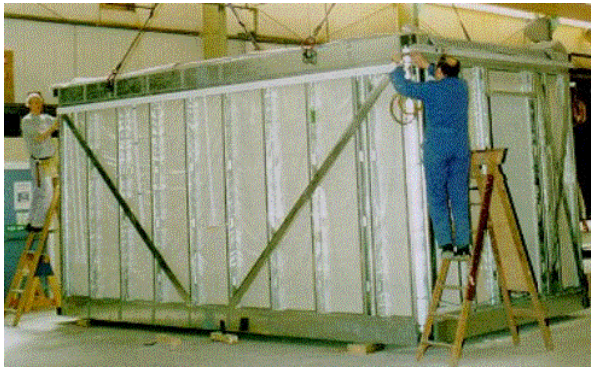
Figure 8.5 – Continuously supported module
