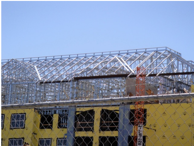
Figure 1.37 – Three-dimensional truss made by cold-formed steel sections ( http://en.wikipedia.org/wiki/File:WikiCFSbuilding.jpg )
