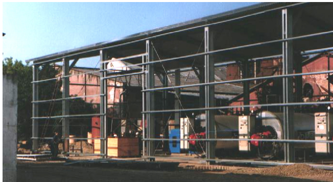
Figure 1.21 – Z and C sections used as: a) purlins; b) girts
