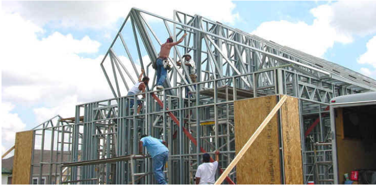
Figure 8.21 – Phase V: Roof trusses are assembled
