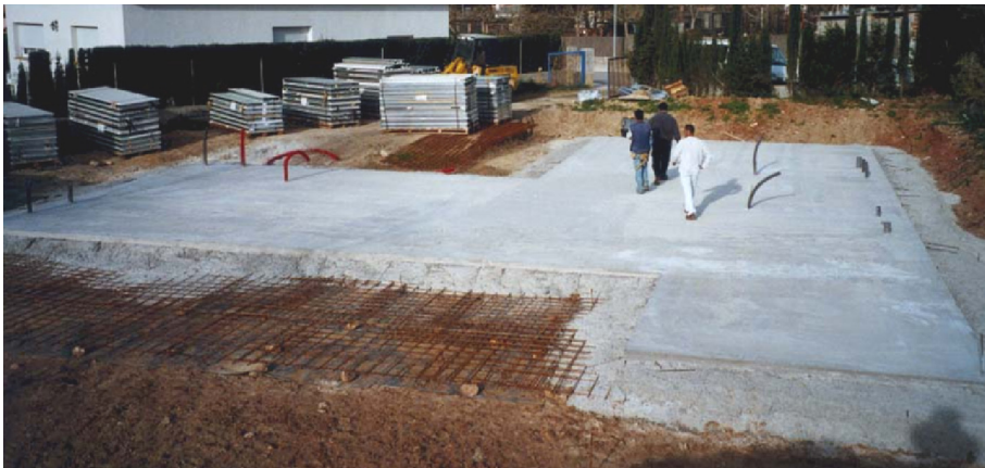
Figure 8.18 – Phase II: Foundation
