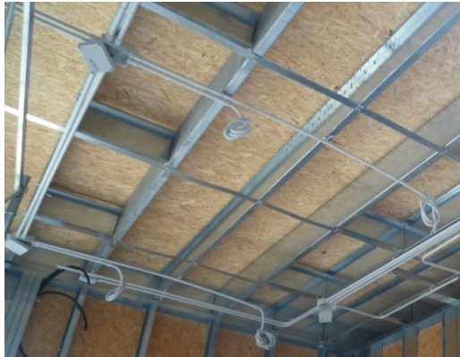
Figure 8.38 – Intermediate torsional restraints system for floors
