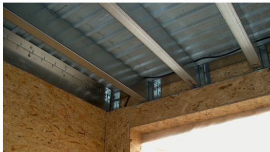
Figure 1.27 – Cold-formed steel joist positioned on the load bearing wall stud structure
