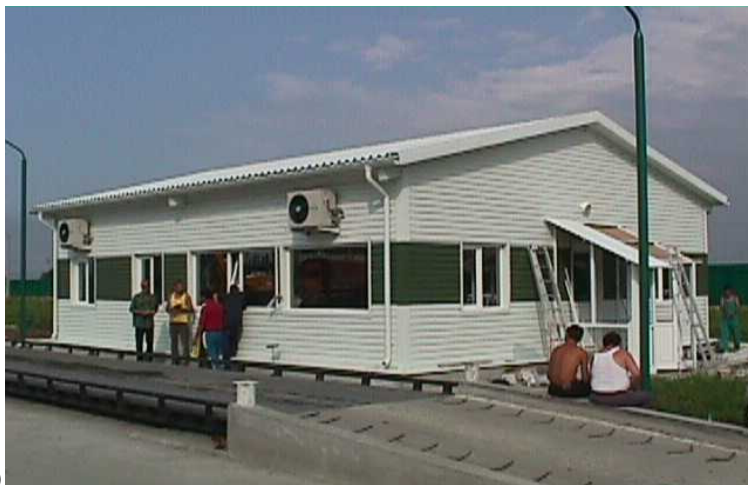
Figure 1.32 – Wall Stud Modular System (WSMS) for small and medium size building facilities using trusses for roof structure and resistance against horizontal actions:a) structural concept; b) framing structure; c) building completed (Dubina et al , 2001a)
