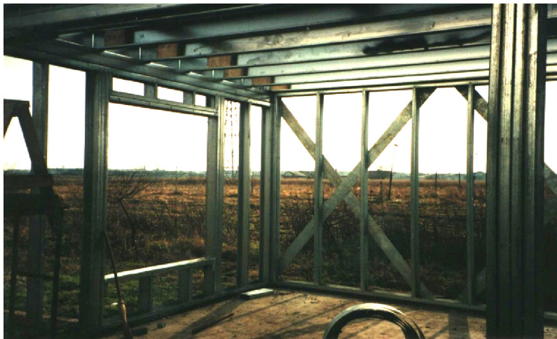
Figure 1.23 – Wall partition inside of building a) Steel house skeleton; b) Shear resistant stud wall
