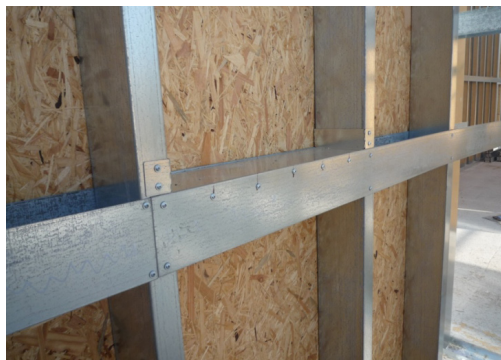
Figure 8.40 – Intermediate torsional restraints system for walls
