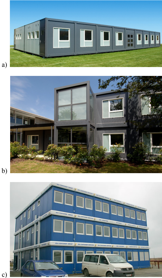
Figure 1.38 – Prefabricated modular units used for schools and offices: a) American School in Bucharest ( http://www.algeco.ro/ ); b) Office building ( http://www.algeco.ro/ ); c) Sea Container Group, Constanta – Romania ( http://www.containex.ro/ )
