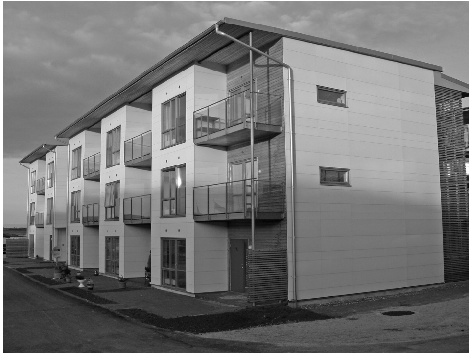
Figure 14.23 Balconies supported between the modules. (Courtesy of Open House AB.)
