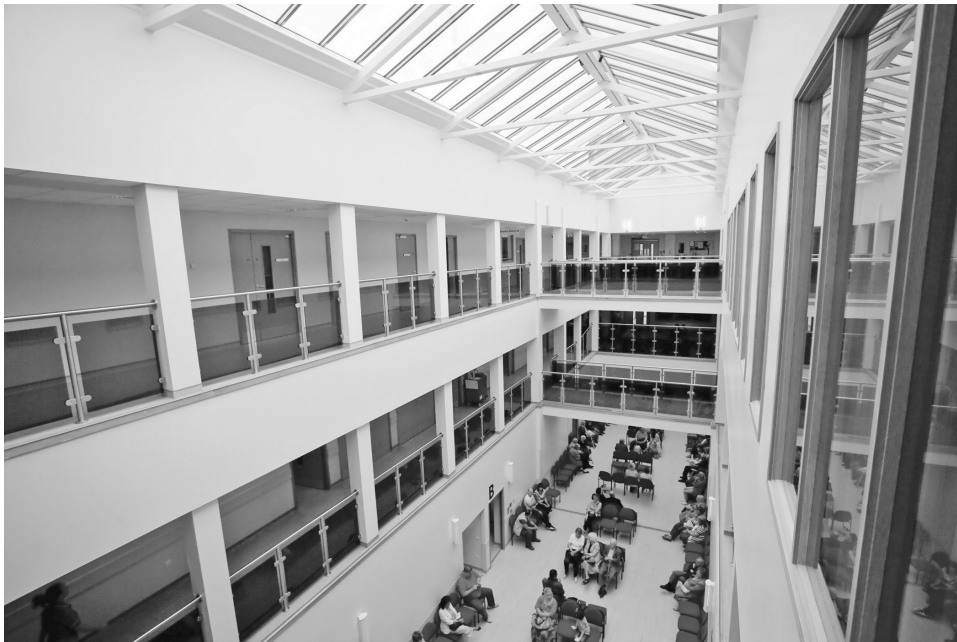
Figure 5.7 Open-sided module with corner posts used to create a walkway and atrium structure at Hull Royal Infirmary. (Courtesy of Portakabin.)
