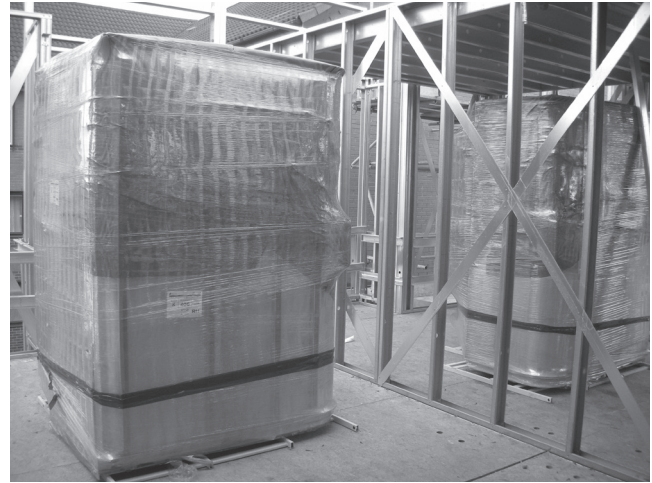
Figure 4.17 PVC bathroom pod positioned on a light steel floor. (Courtesy of Offsite Solutions and Metek.)
