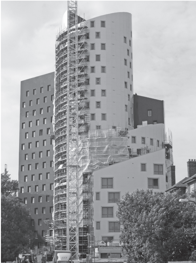
Installation of lightweight cladding by mast climbers. (Courtesy of Futureform.)
