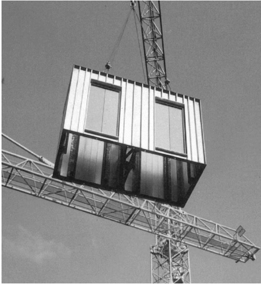
Figure 15.10 Modular lift system using light steel components. (Courtesy of Schindler.) Figure 15.11 Lift dimensions to BS ISO 419011.
