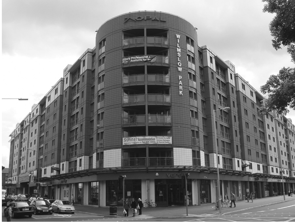
Figure 1.15 Mixed commercial–residential development at Wilmslow Road, Manchester, using 1400 modules on a steel composite podium structure. (Courtesy of Rollalong and Ayrshire Steel Framing.)
