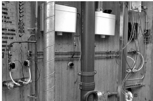
Figure 15.6 Services installed as part of a precast modular unit in manufacture. (Courtesy of Precast Cellular Structures Ltd.)
