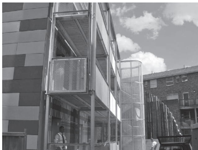
View of prefabricated steel walkways and stairs on the rear façade.
