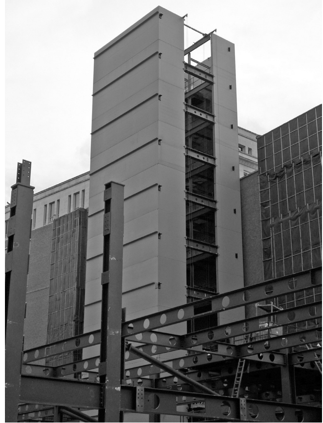
Figure 4.26 Corefast lift module as delivered to site and installed. (Courtesy of Tata Steel.)
