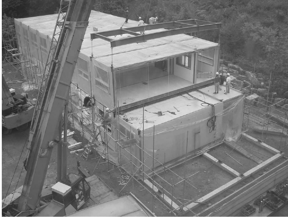
Figure 1.17 Open-sided module used with an integral corridor used in a school building in Seoul, Korea. (Courtesy of POSCO.)
