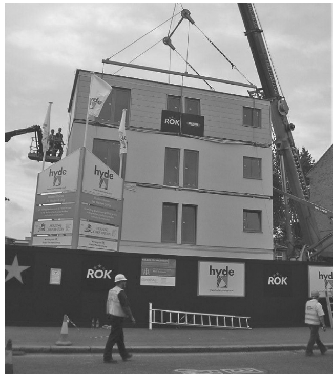
Installation of modules along the front façade to the building.
