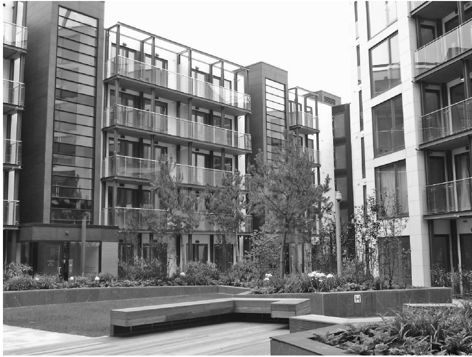
Figure 14.10 Mixed use of insulated render, rain screen cladding, and ground-supported balconies in modular apartments in Dublin.
