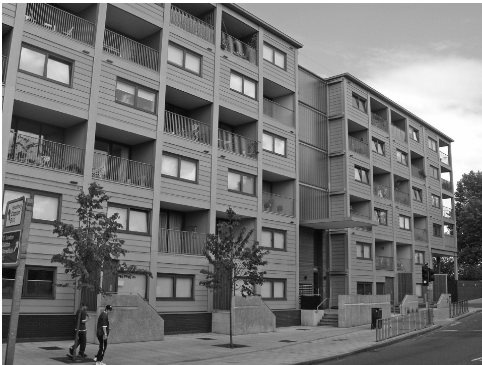
Figure 14.22 Balconies integrated into the modules at Raines Court, north London. (Courtesy of Yorkon.)
