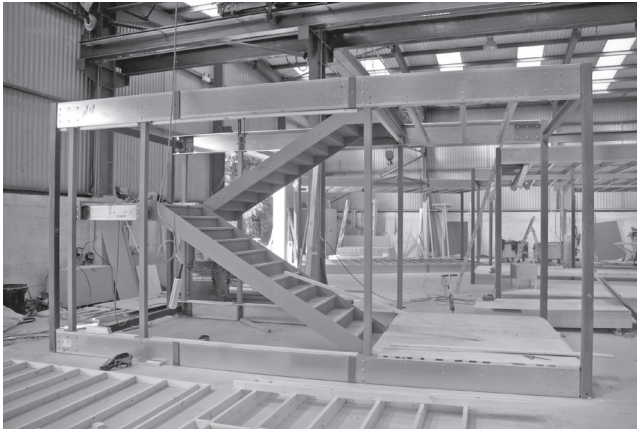
Figure 4.18 Stair module with corner posts. (Courtesy of Kingspan Steel Building Solutions.)
