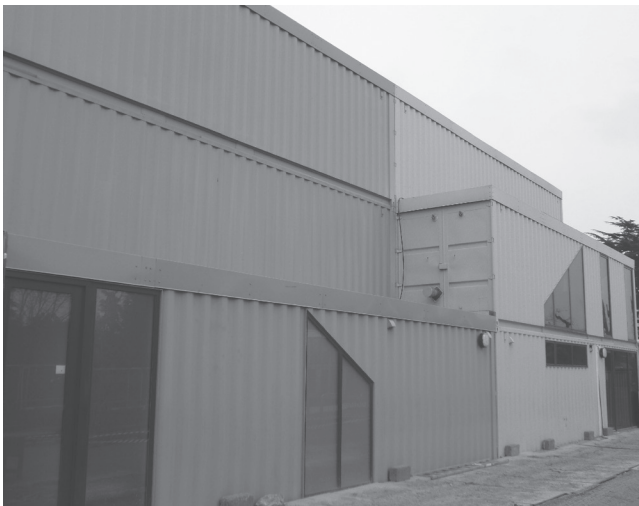
Figure 4.9 New sports hall and gymnasium using containers to support the roof. (Designed by SCABEL Architects.)
