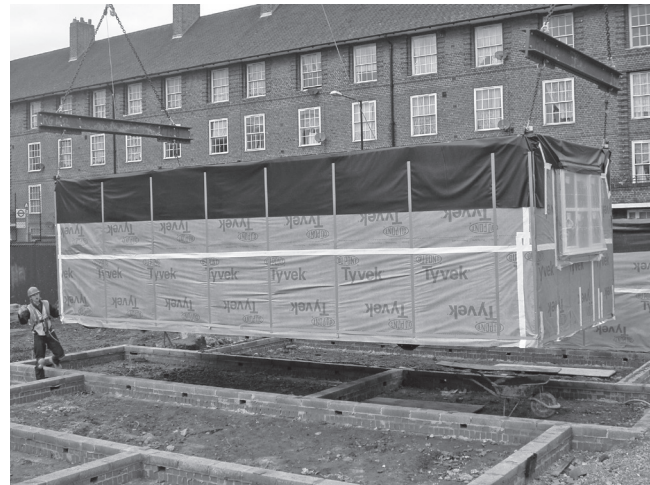
Installation of modules on brickwork footings and strip foundations.
