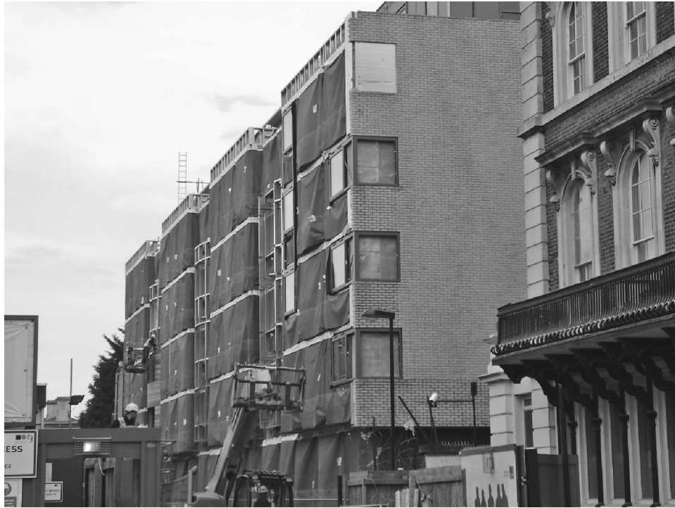
Figure 14.7 Bonded brick tile cladding to a student residence in north London. (Courtesy of Unite Modular Solutions.)
