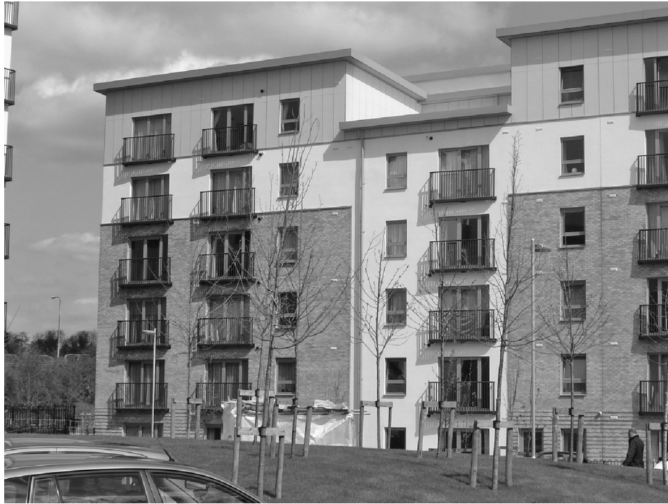
Figure 14.5 Ground-supported brickwork up to 4 storeys high and insulated render above for a modular residential development in Basingstoke.
