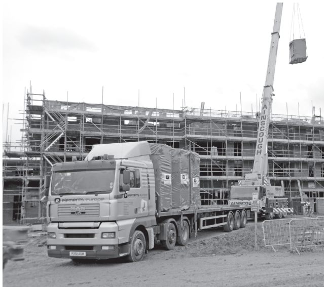
Figure 4.16 Installation of modular bathroom unit. (Courtesy of Elements Europe.)
