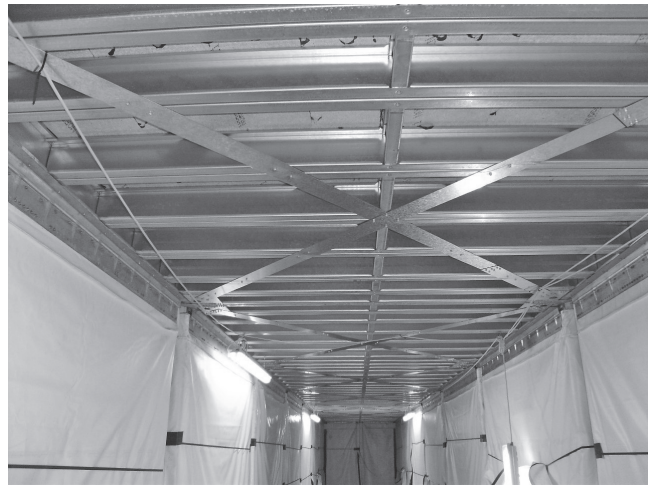
X-bracing in the corridors for stability.
