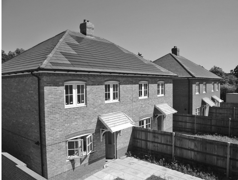
Figure 14.16 Photovoltaic roof tiles used in a traditional house. (Courtesy of Woking Borough Council.)
