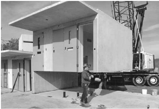
Figure 13.6 Balcony cast into a precast module. (Courtesy of Oldcastle Precast.)
