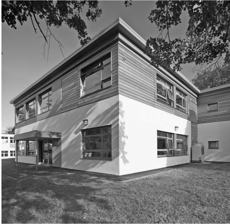
Figure 8.1 School building constructed using modules and with site-installed cladding. (Courtesy of Yorkon.)
