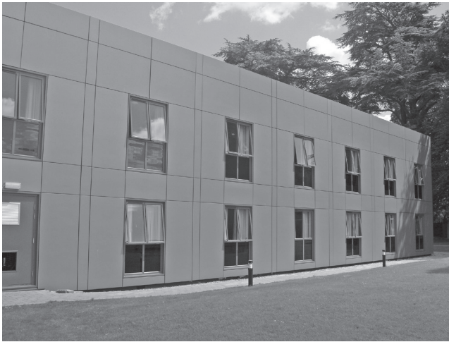
View of the large metallic cladding panels to the modular accommodation building.
