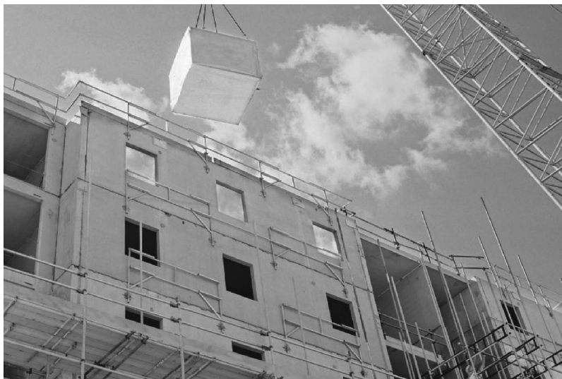
Figure 3.9 Concrete bathroom pod being lifted into student residence built in cross-wall construction at the University of West of England (UWE), Bristol. (Courtesy of Buchan, Concrete Centre, 2007.)
