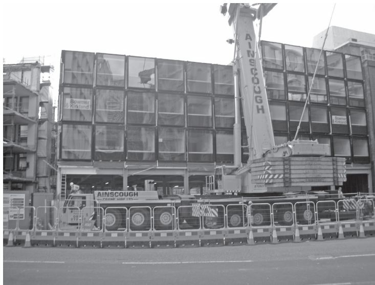
Figure 6.21 Installation of modules on a steel podium for a hotel in central London. (Courtesy of Futureform and Citizen M hotels.)
