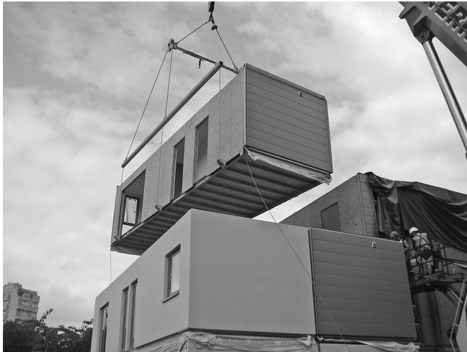
Figure 2.2 Partially open-sided module with load-bearing walls. (Courtesy of PCKO Architects.)
