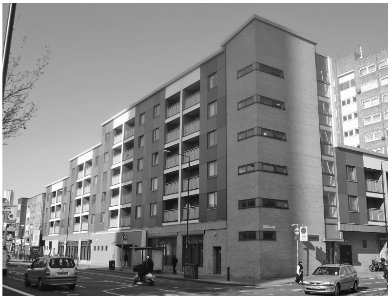
Figure 1.4 Residential building constructed on a podium structure with offices below on Commercial Road, east London. (Courtesy of Rollalong.)
