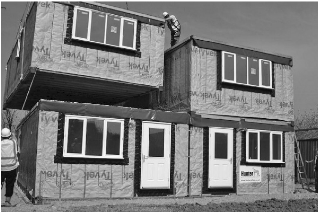
Figure 4.4 Timber modules being assembled on site. (Courtesy of Hunter Offsite Ltd.)
