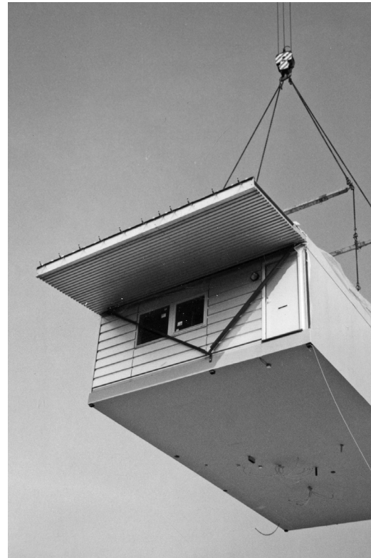
Figure 4.23 Modular rooftop units with a glazed façade used in building renovation in Copenhagen and also showing a module being lifted into place.
