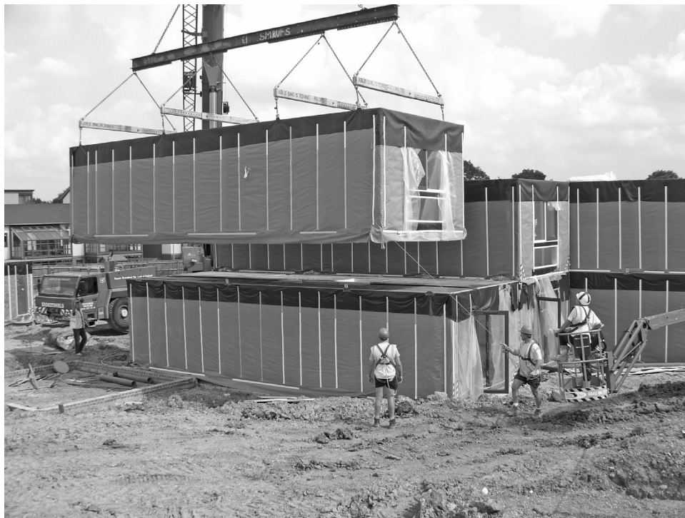
Figure 16.14 Lifting of light steel module by main beam and crossbeams. (Courtesy of Futureform.)
