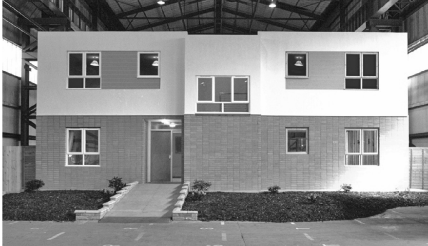
Figure 10.3 Demonstration building using hybrid modular and panel construction.
