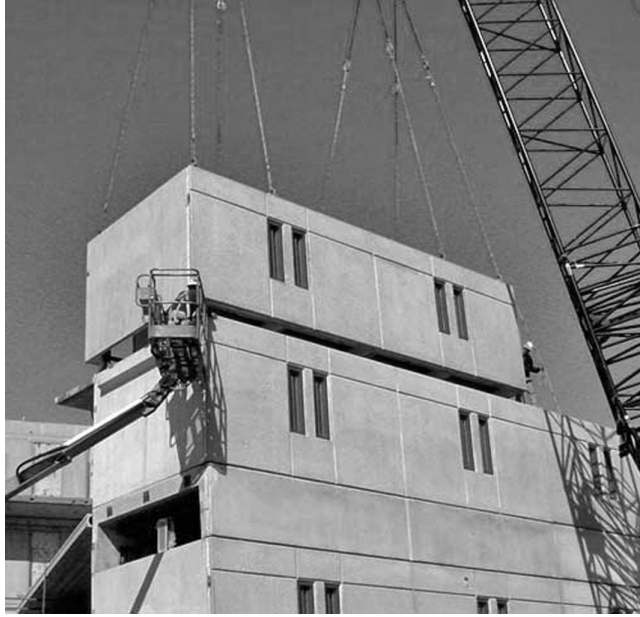
Figure 16.20 Installation of precast concrete modules on site. (Courtesy of Oldcastle Precast.)
