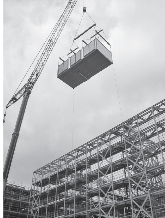
Installation of modules with three large patio windows. (Courtesy of Yorkon.)
