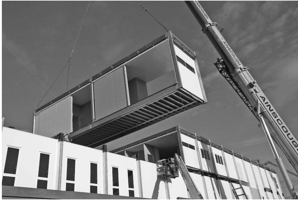
Figure 7.3 Modular hospital unit during construction. (Courtesy of Yorkon.)
