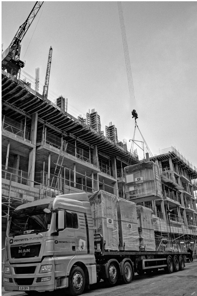
Figure 1.10 Installation of bathroom pods in a concrete-framed building. (Courtesy of Elements Europe.)
