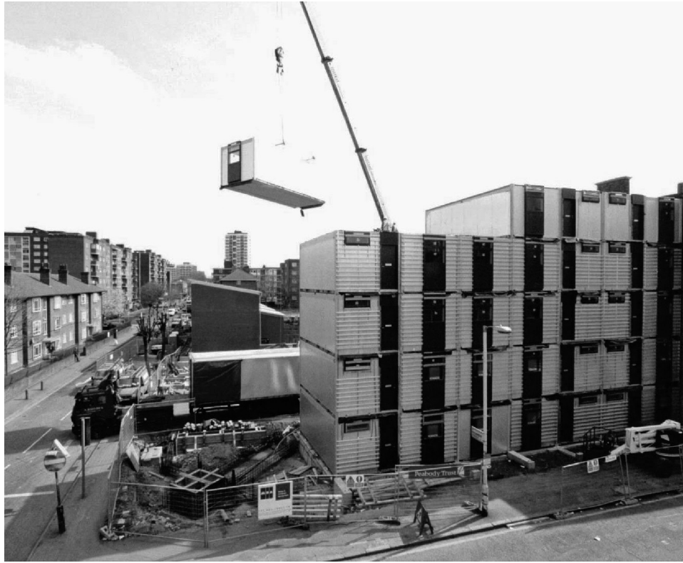
Figure 1.1 Installation of modular units and completed building at Murray Grove, north London. (Courtesy of Yorkon and Cartwright Pickard architects.)
