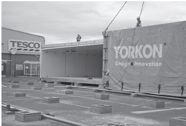
Installation of single-storey modules for the supermarket. (Courtesy of Yorkon.)
