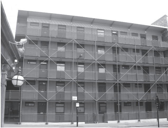
Roadside view showing the external walkways and X-bracing. (Courtesy of Yorkon and Cartwright Pickard Architects.)
