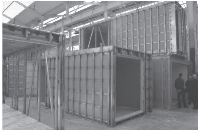
Partially completed modules built in the nearby field factory set up for this project.
