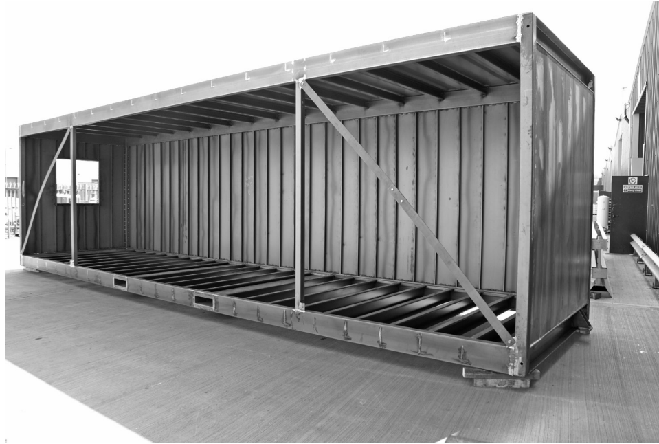
Figure 2.6 Corner-supported module with intermediate posts. (Courtesy of BW Industries.)
