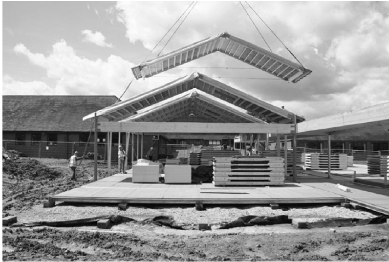
Figure 4.1 Flat-pack modular timber panels used at Stantonbury School, Milton Keynes. (Courtesy of Terrapin.)
