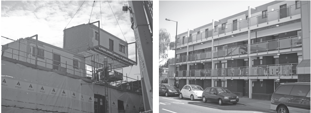
Figure 4.24 Installation of rooftop modules and completed renovation of a 1960s housing block in west London. (Courtesy of Powerwall.)
