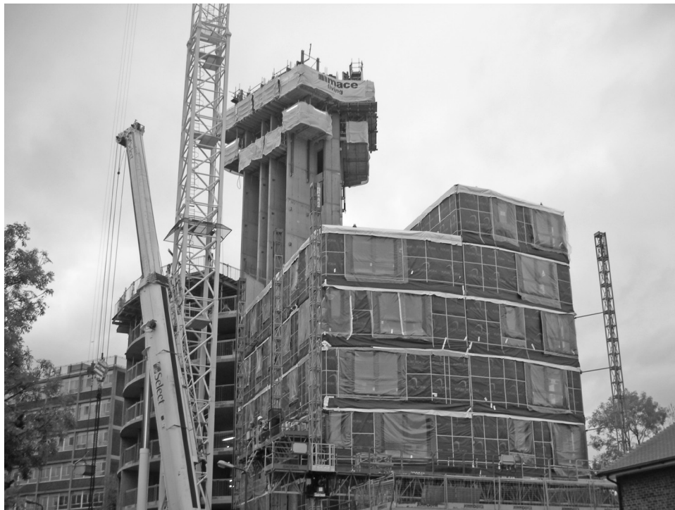
Figure 6.23 High-rise modular building in Wembley using an in situ concrete core. (Courtesy of Futureform.)
