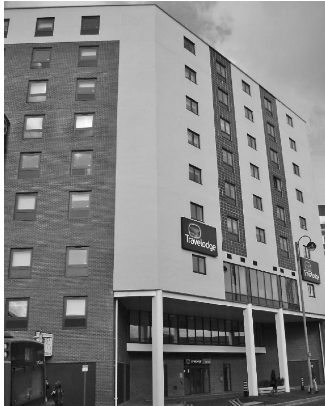
Figure 4.12 Hotel in Uxbridge, West London, constructed using shipping containers. (Courtesy of Verbus.)
