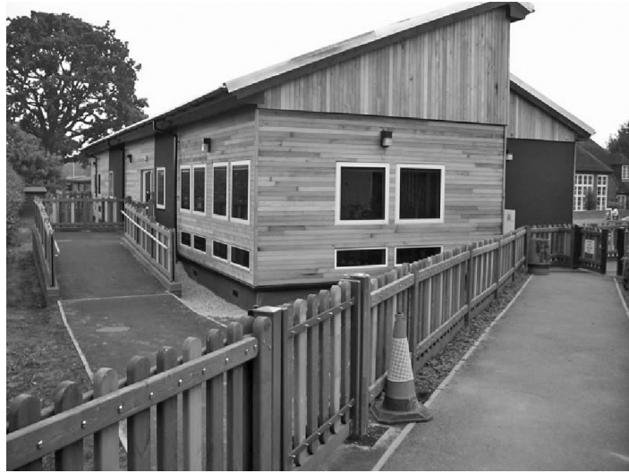
Figure 8.5 Primary school using timber modules and cladding. (Courtesy of Terrapin.)
