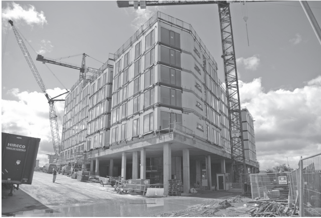
Installation of modules on a concrete podium.
