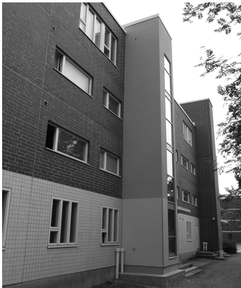
Figure 4.25 Four-storey modular lift used in building renovation in Helsinki. (Courtesy of NEAPO.)
