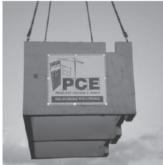
Double-lift shaft module being lifted into place.
