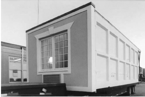
Figure 3.6 Precast modular hotel units being transported to site. (Courtesy of Oldcastle Precast.)
