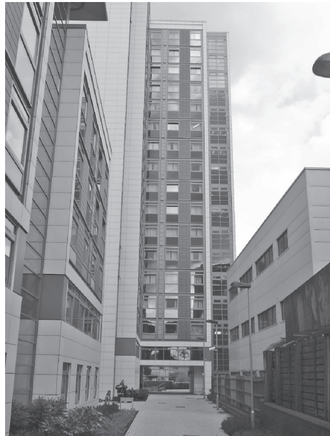
Figure 5.9 Modular building stabilised by a concrete core in construction and completed. (Courtesy of Caledonian Modular.)
