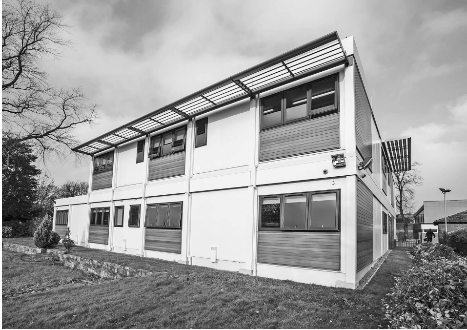
Figure 8.3 Modules with prefinished cladding used in Sixth Form College near Wigan. (Courtesy of Foremans Relocatable Building Systems.)
