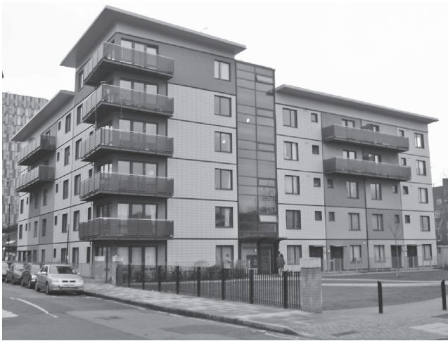
View of the building showing the large balconies attached to the modules.
