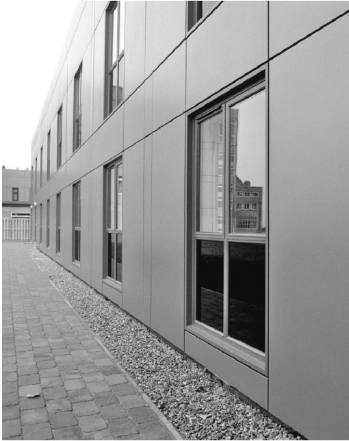
Figure 14.9 Metallic cladding to conference centre in Leamington Spa. (Courtesy of Terrapin.)
