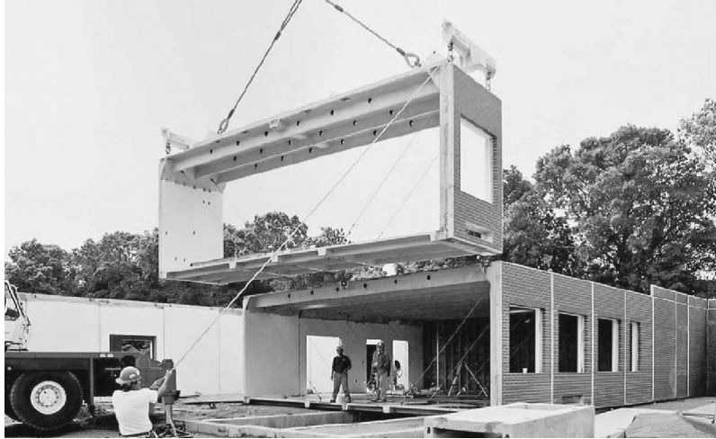
Figure 3.8 Installation of precast modular units for a school. (Courtesy of Oldcastle Precast.)
