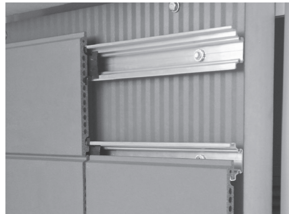
Figure 14.4 Tiles supported by composite panels. (Courtesy of Kingspan.)
