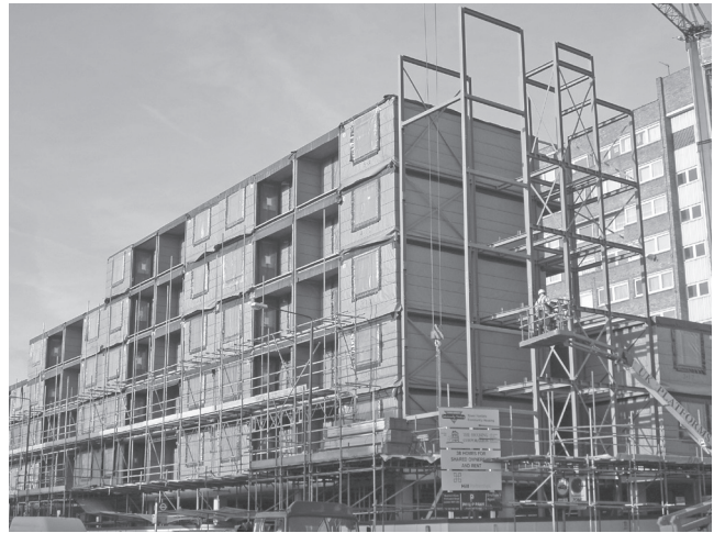
Modules with the braced steel access cores at one end. (Courtesy of Rollalong.)
