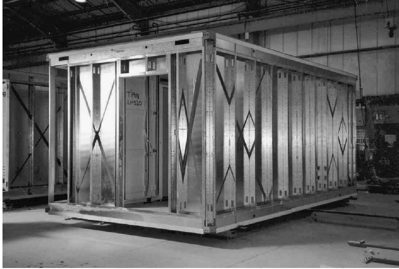
Figure 2.1 Continuously supported module in light steel framing in which wall loads are transferred by bearing through the floor and ceiling cassettes. (Courtesy of Terrapin.)
