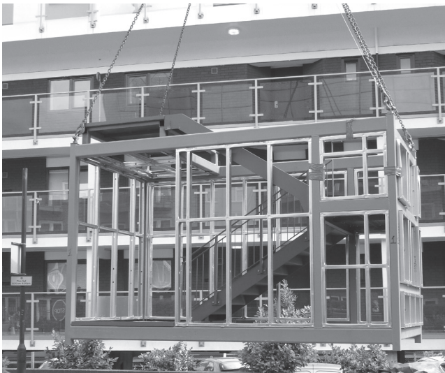
Figure 4.19 Stair module using welded RHS members being lifted into place. (Courtesy of Powerwall.)
