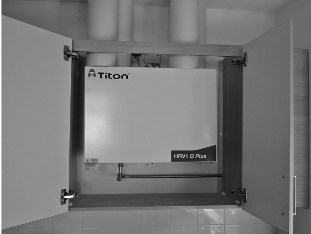
Figure 14.18 Mechanical ventilation and heat exchanger installed in a kitchen unit in a module. (Courtesy of Futureform.)
