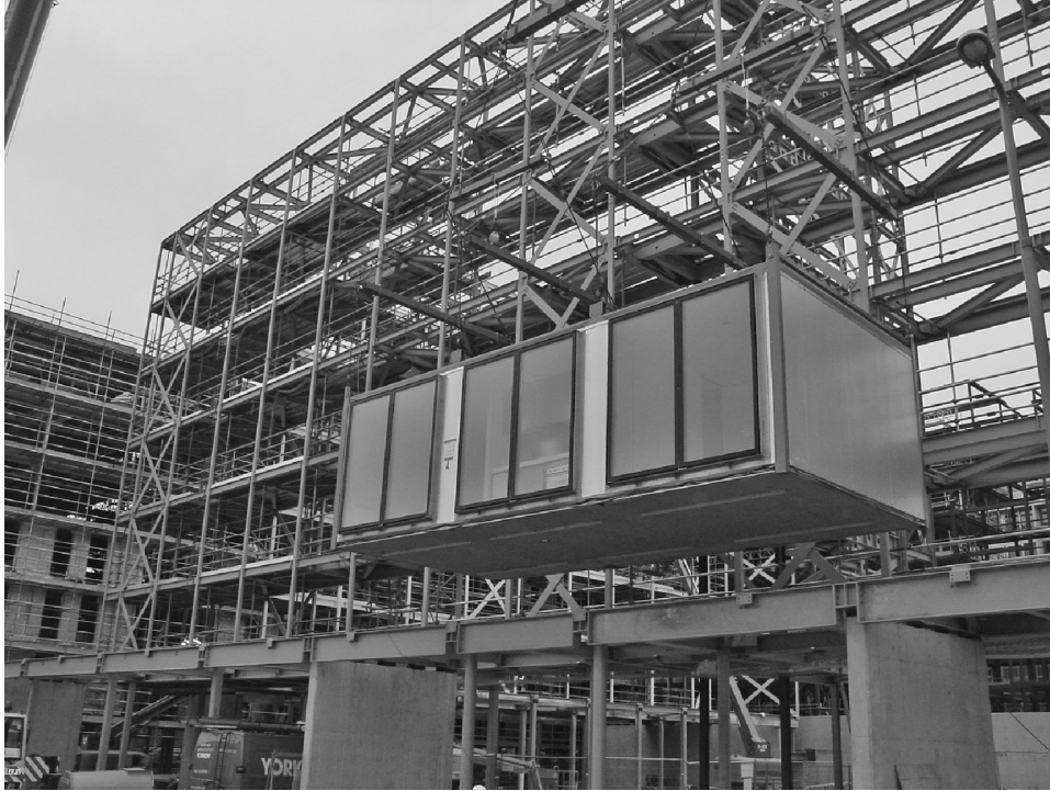
Figure 5.6 Open-sided module with corner and intermediate posts supported by a structural frame. (Courtesy of Yorkon and Joule Engineers.)
