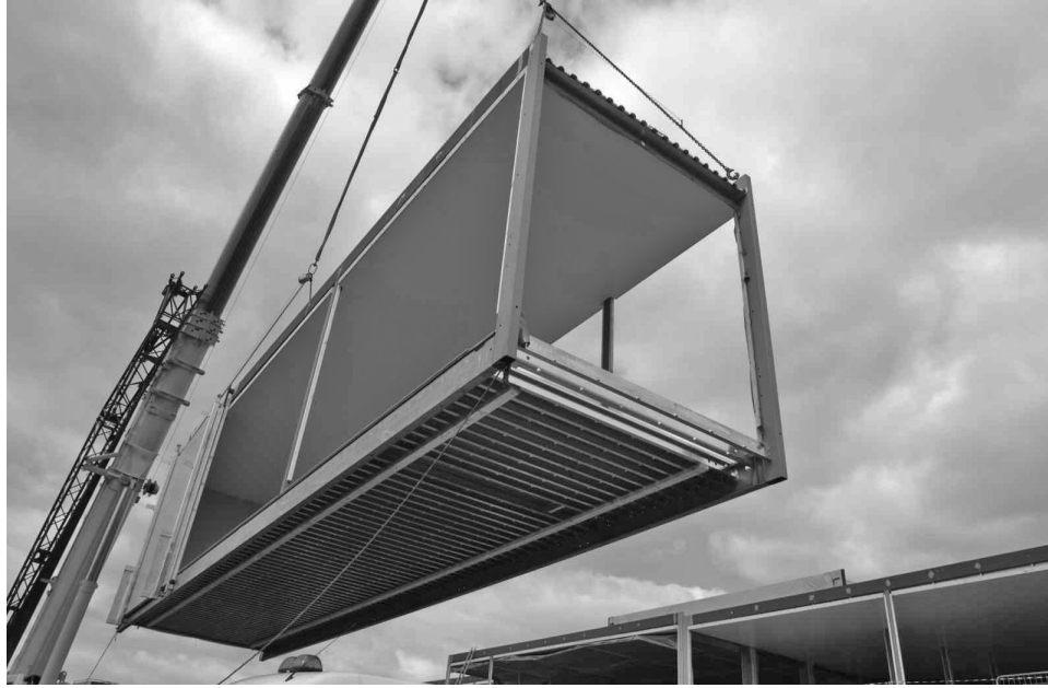
Figure 16.13 Lifting of module from the corner posts without a lifting beam. (Courtesy of Yorkon.)
