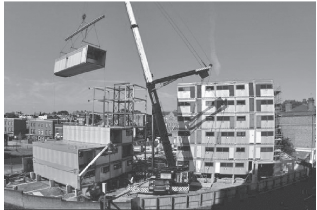
View of a module being installed. (Courtesy of Yorkon.)
