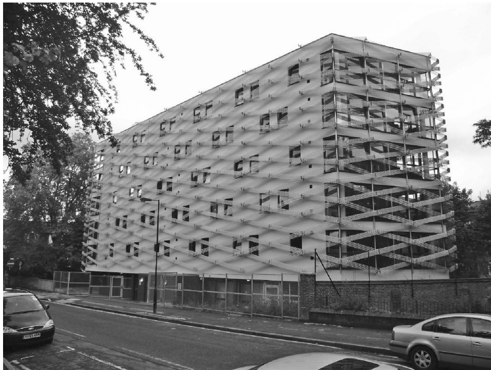
Figure 14.6 Innovative insulated render and metallic cladding to a student residence in north London. (Courtesy of Unite Modular Solutions.)
