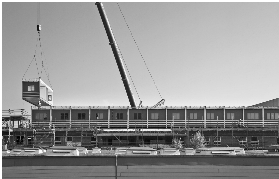
Figure 7.14 Installation of open-sided rooftop modules at Harrogate District Hospital. (Courtesy of Yorkon.)
