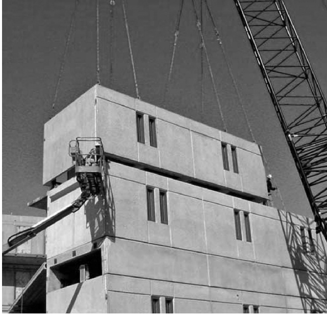
Figure 3.1 Installation of precast concrete modules on site. (Courtesy of Oldcastle Precast.)
