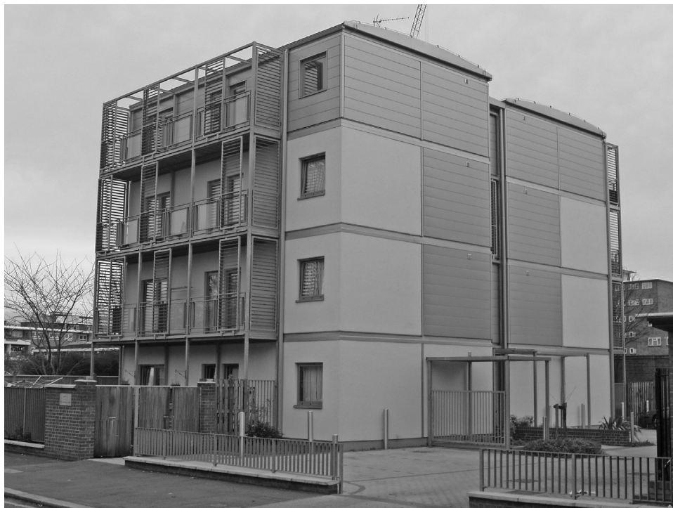
Figure 6.11 Modules create flexible use of space in Stockwell, south London. (a) Plan form showing partially open sides (alternate modules are shaded). (b) View of completed building. (Courtesy of PCKO Architects.)
