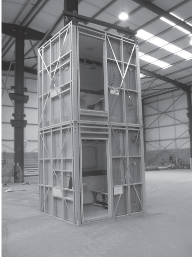
Figure 4.15 Light steel load-bearing bathroom modules.
