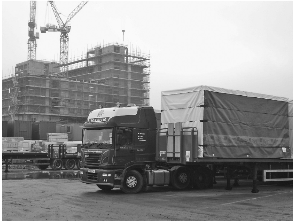
Figure 17.13 Protective breathable shroud around a module for delivery to the site. (Courtesy of Unite Module Solutions.)
