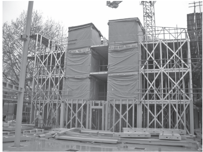
Internal view of X-braced cross-walls and modular bathrooms.
