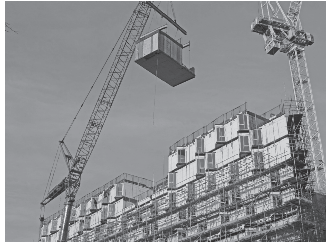
Installation of a module with a concrete base.
