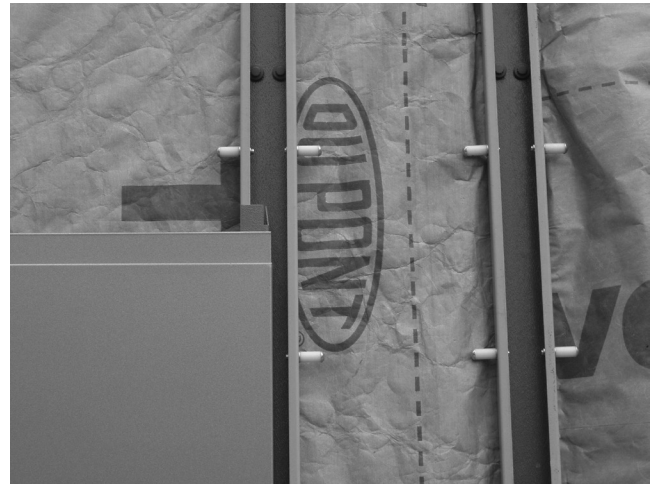
Detail of attachment of rain screen panels to vertical runners fixed to the modules.
