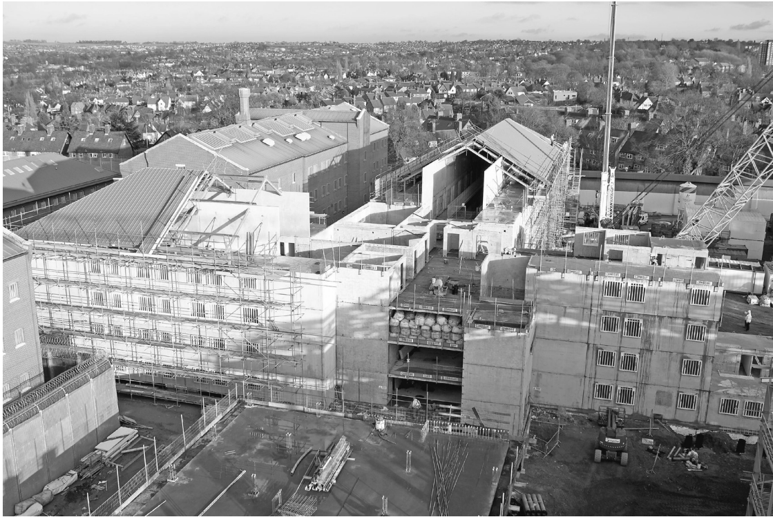
Precast concrete modules during installation. (Courtesy of Pre-cast Cellular Structures Ltd.)
