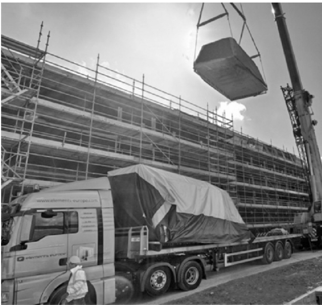
Figure 14.14 Mansard roof modules used in a 5-storey student residence in York. (Courtesy of Elements Europe.)
