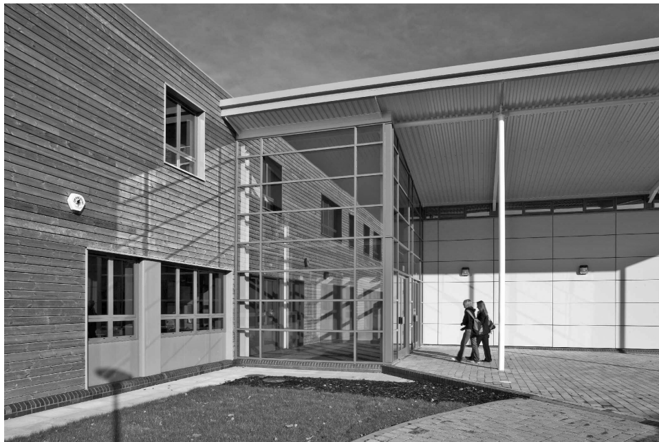
Figure 8.2 Mixed use of steel frames and modules in a school entrance area. (Courtesy of Yorkon.)
