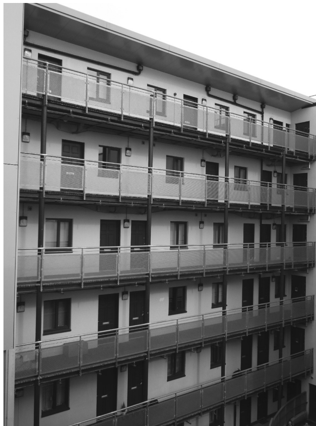
Figure 5.5 Rear view of a group of modules with an external access structure supported by intermediate posts. (Courtesy of Caledonian Modular.)
