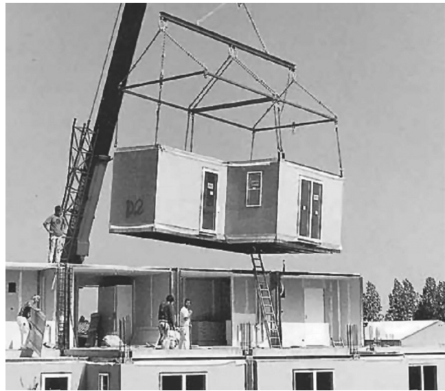
Installation of L-shaped module. (Courtesy of Open House AB.)
