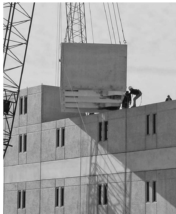
Figure 13.7 Installation of precast concrete modules on site showing the temporary support to the base of the walls. (Courtesy of Oldcastle Precast.)
