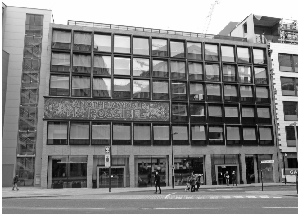
Figure 2.8 Citizen M hotel in Southwark, London, with fully glazed open-ended modules. (Courtesy of Futureform.)
