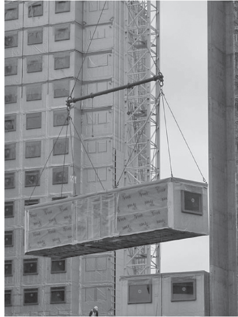
Installation of double-length module at the lower levels.
