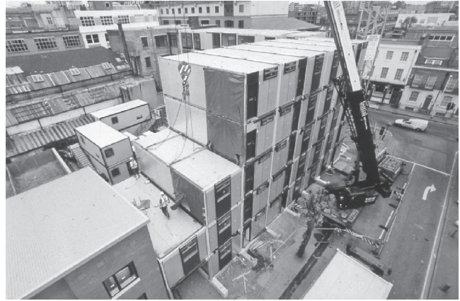
Installation of a module by mobile crane (Courtesy of Yorkon.)
