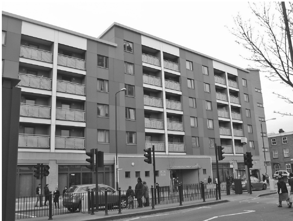
Figure 14.8 Rain screen cladding to social housing in east London. (Courtesy of Rollalong.)
