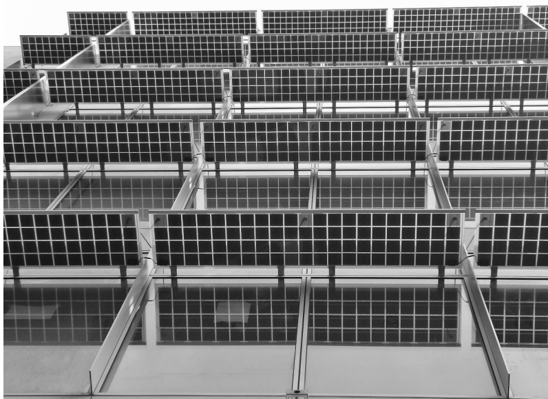
Figure 14.17 Photovoltaic glazing used as solar shading.
