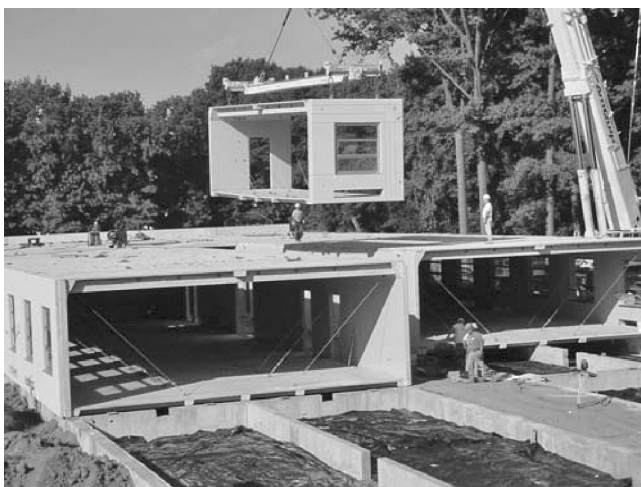
Figure 16.11 Installation of open-sided modular precast concrete units onto ground beams. (Courtesy of Oldcastle Precast.)
