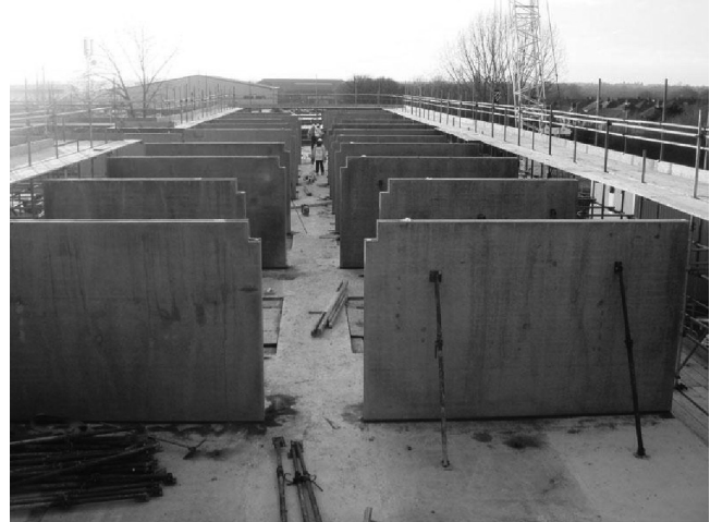
Figure 3.2 Typical cross-wall construction. (Courtesy of Precast Structures.)
