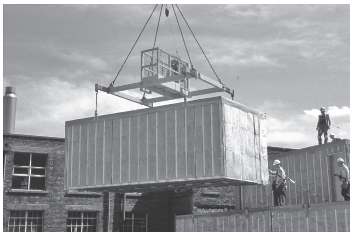
Figure 16.16 Lifting of module using a protective cage attached to the crane hook. (Courtesy of Ayrshire Framing.)
