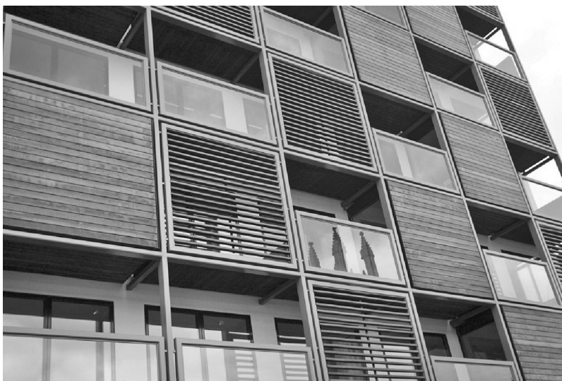
Figure 14.20 Balconies supported by a separate structure at MOHO Manchester. (Courtesy of Yorkon.)
