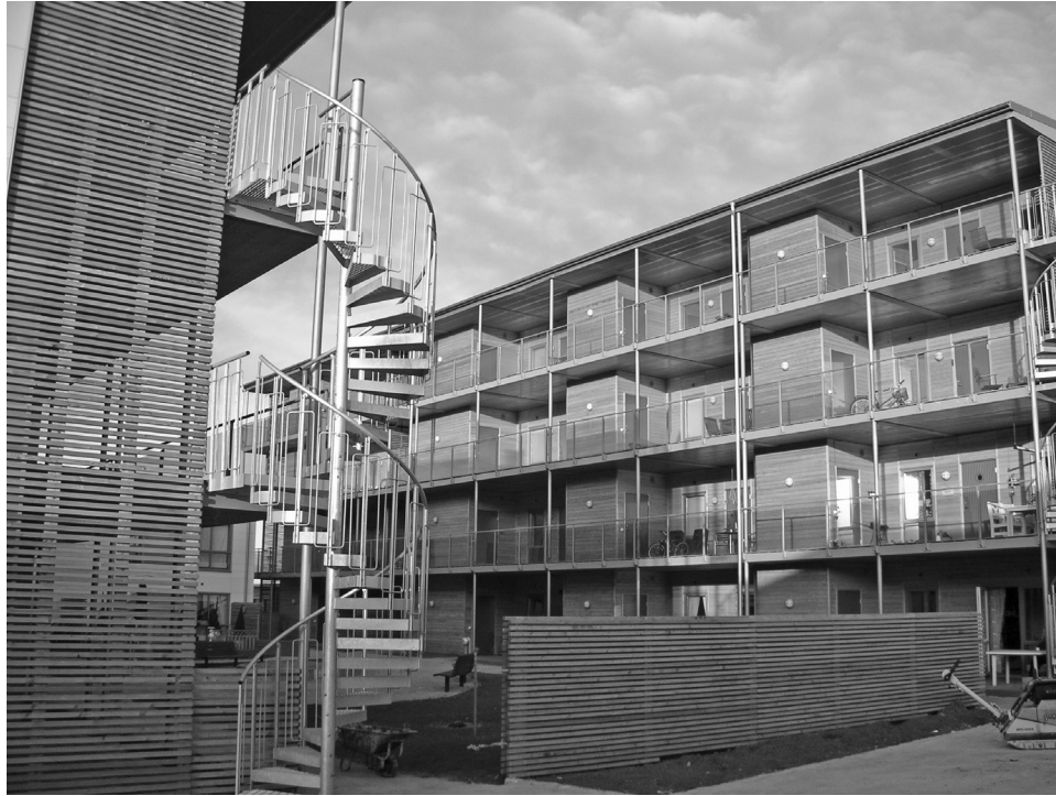
Figure 14.19 Ground-supported balconies in a modular housing, Malmö, Sweden. (Courtesy of Open House AB.)
