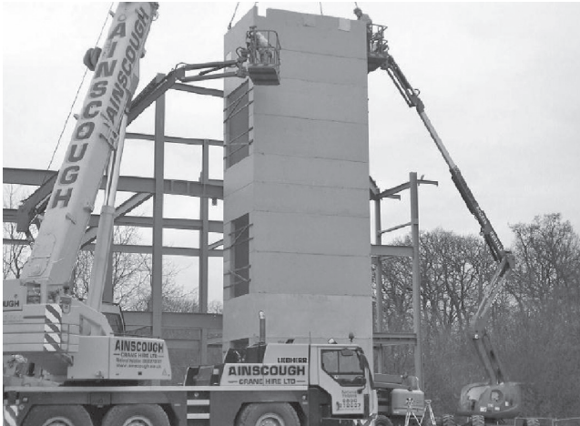
Precast concrete lift modules during installation. (Courtesy of PCE Design & Build.)
