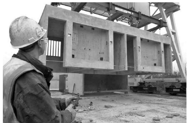
Figure 16.19 Lifting a concrete module using a spreader beam. (Courtesy of PCSL.)
