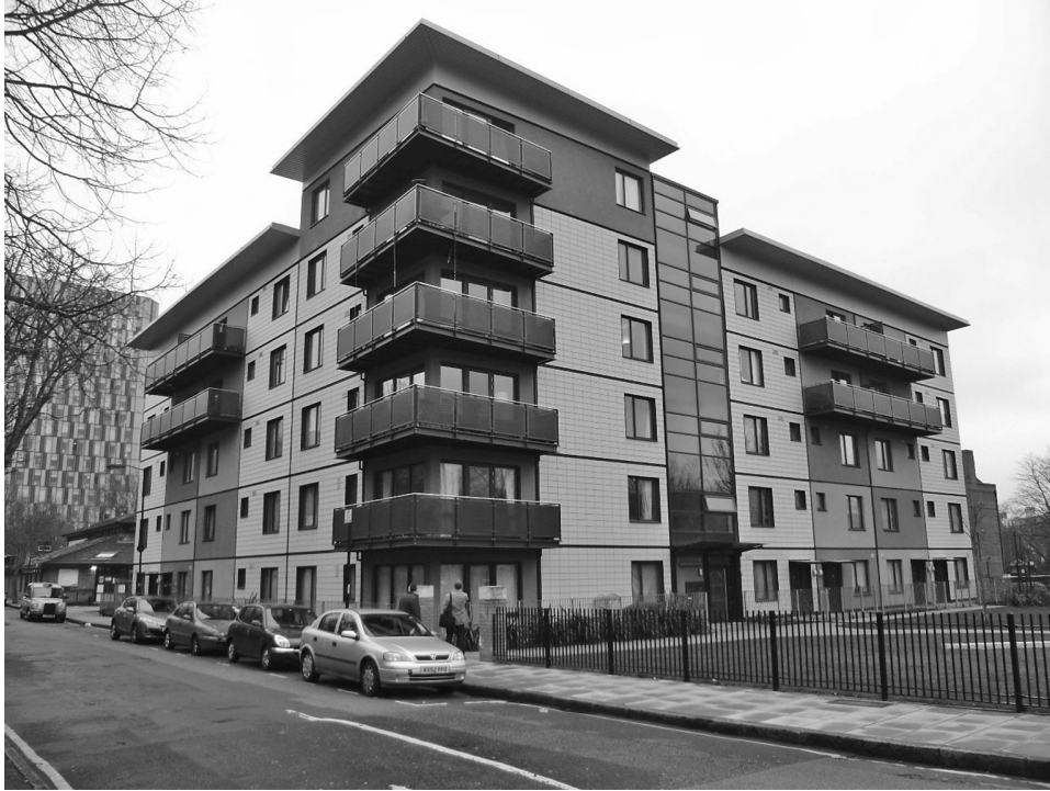
Figure 14.21 Balconies supported at corner posts of modules. (Courtesy of Caledonian Modular.)
