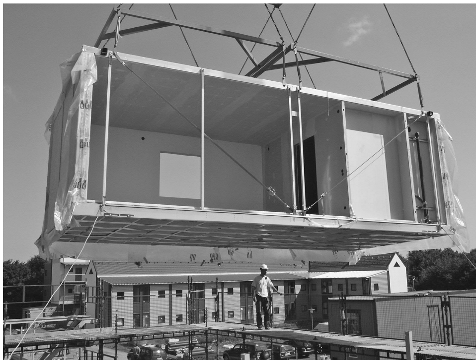
Figure 16.15 Lifting of light steel module from a rectangular frame. (Courtesy of Open House AB.)
