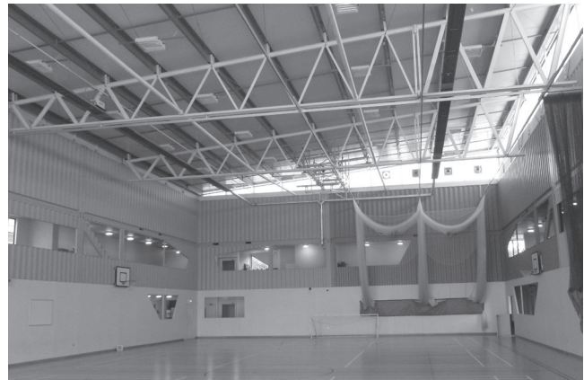
Figure 4.9 New sports hall and gymnasium using containers to support the roof. (Designed by SCABEL Architects.)
