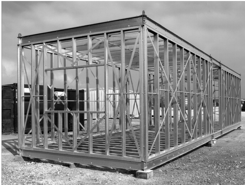
Figure 2.4 Corner-supported module with an intermediate corridor. (Courtesy of Kingspan Steel Building Solutions.)
