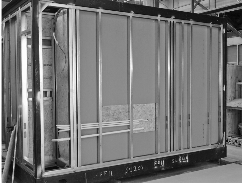
Figure 15.1 Service riser in the corner of a module. (Courtesy of Caledonian Modular.)
