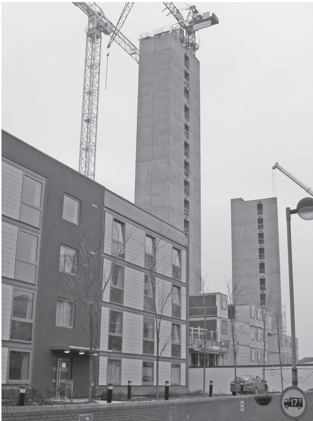
Figure 5.9 Modular building stabilised by a concrete core in construction and completed. (Courtesy of Caledonian Modular.)
