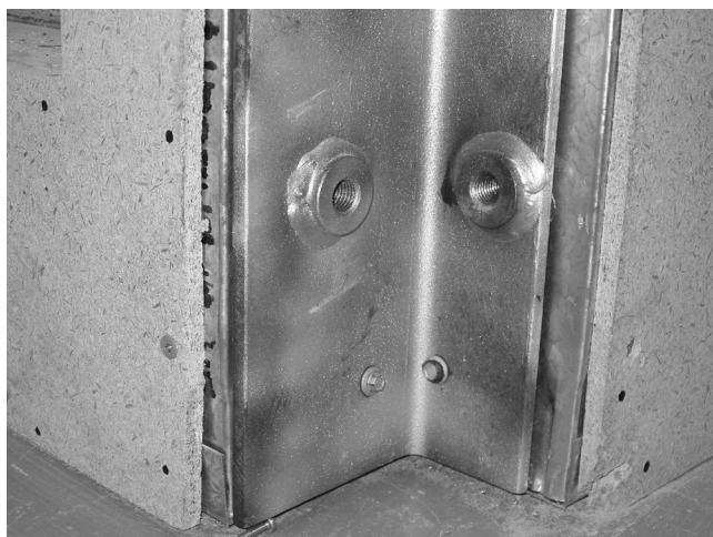
Figure 12.5 Corner angle with welded nut to connect the tie plate.
