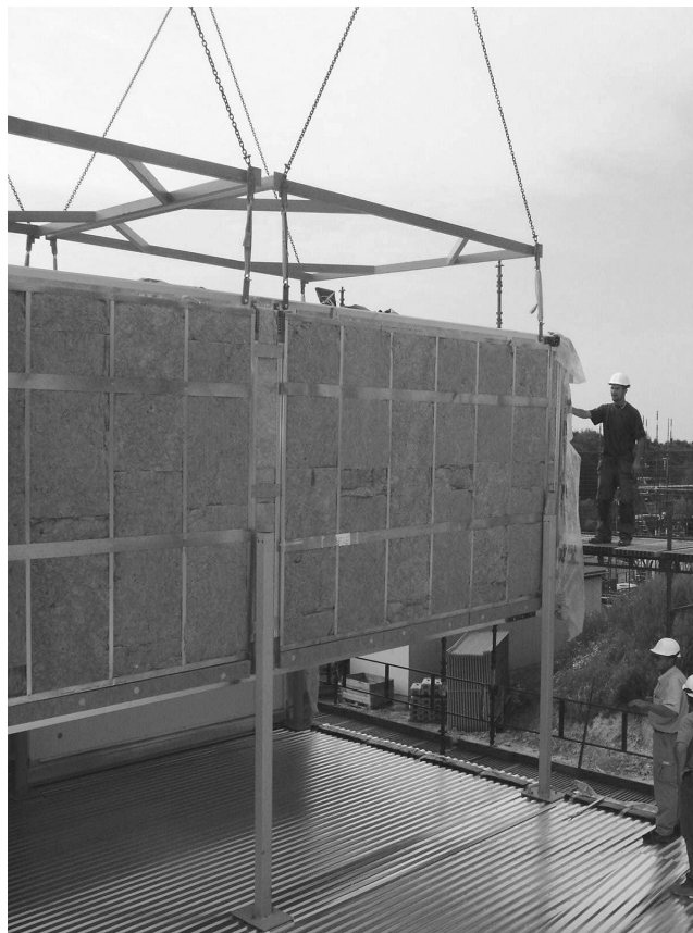
Figure 5.15 Installation of modules with recessed corners around SHS posts. (Courtesy of Open House AB.)
