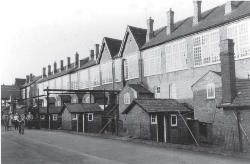
**Figure 6.** Home and workplace: some of Cash's "Hundred Houses" in Coventry in the 1970s. The top floor workshops housed jacquard ribbon looms, supplied by power from a central steam engine.
