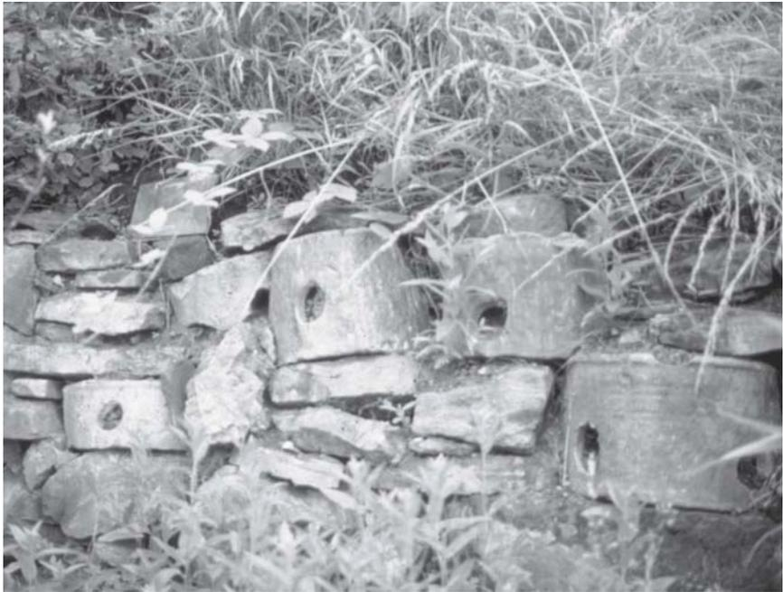
**Figure 4.** Saggars to hold salt-glazed pottery in a kiln were used to create garden walls in Jackfield. There is considerable archaeological evidence for local pottery manufacture which is not always well-documented.
