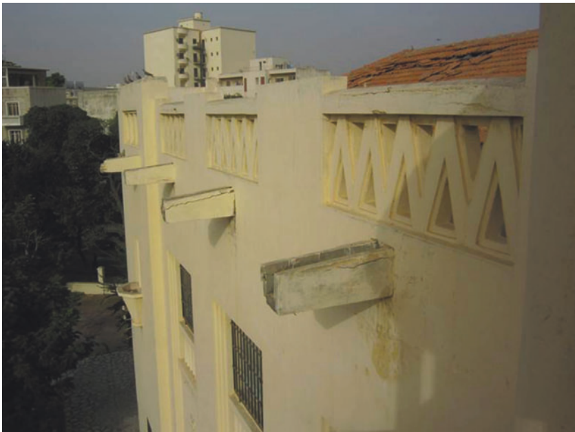
Fig. 10.3 Charles Wulffleff, Museum of Dakar, constructed 1936. Parapet detail with neo-Sudanese downspouts and Zig-Zag balustrade. Author's photograph
