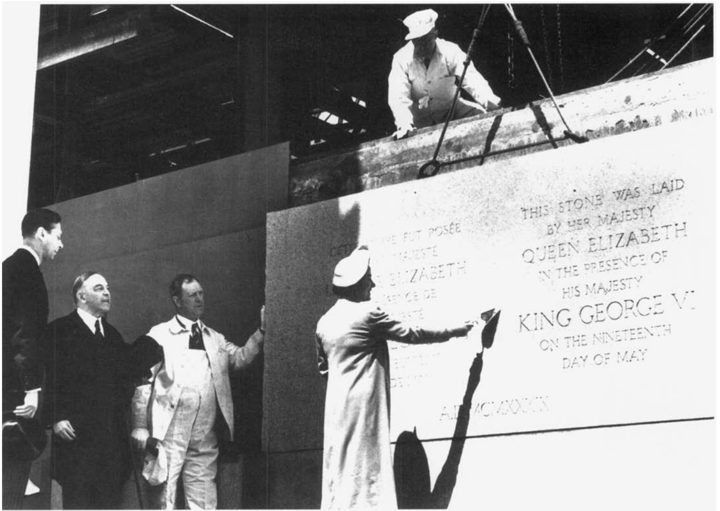
Queen Elizabeth lays the cornerstone of the new building in the presence of King George VI and Prime Minister Mackenzie King
