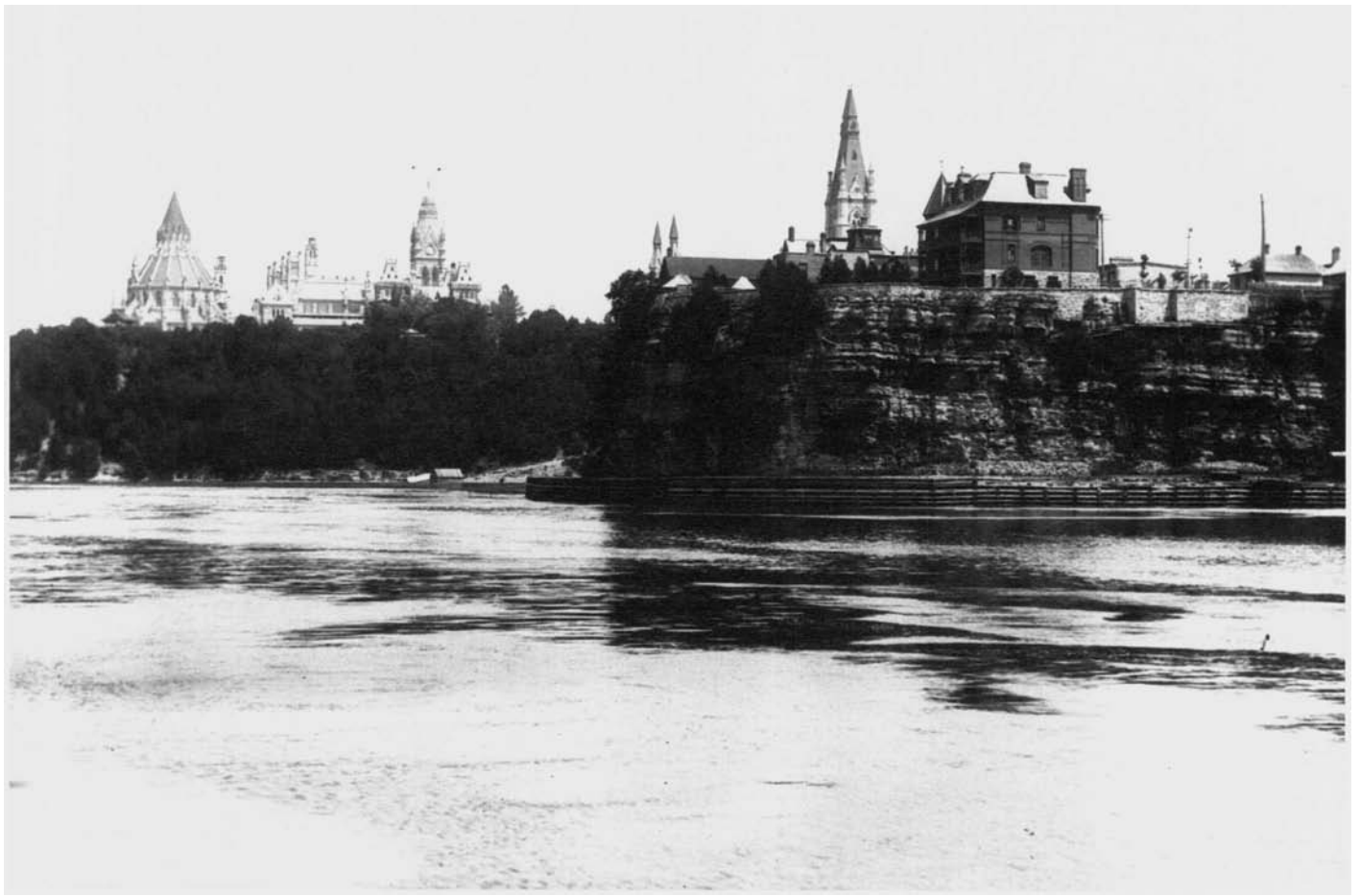
Future site of the Court as it appeared in the 1880s
