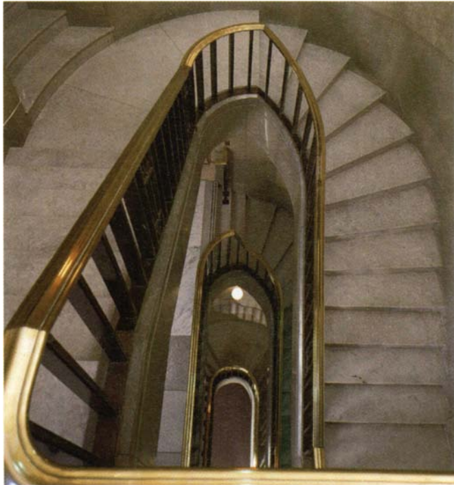
A staircase with grey Missisquoi marble
