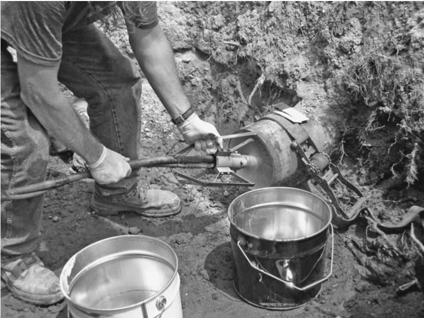
FIGURE 3.7 Epoxy spray head is removed from the pipe. (Source: CuraFlo Inc.)
