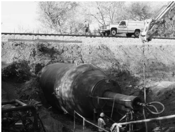
FIGURE 8.20 Culvert installation under railroad using pipe ramming. (Source: TT Technologies.)
