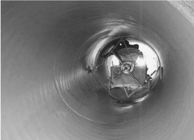
FIGURE 3.6 Cement-mortar lining troweled finish. (Source: www.cementlining.com .)
