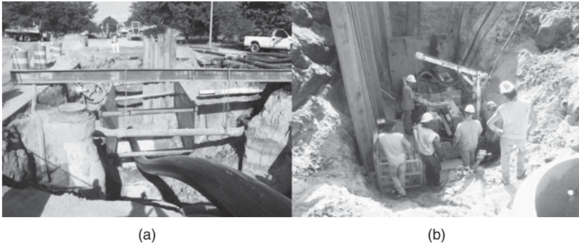
FIGURE 6.1 The pipe bursting operation. (a) Insertion Shaft, and (b) Pulling Shaft.
