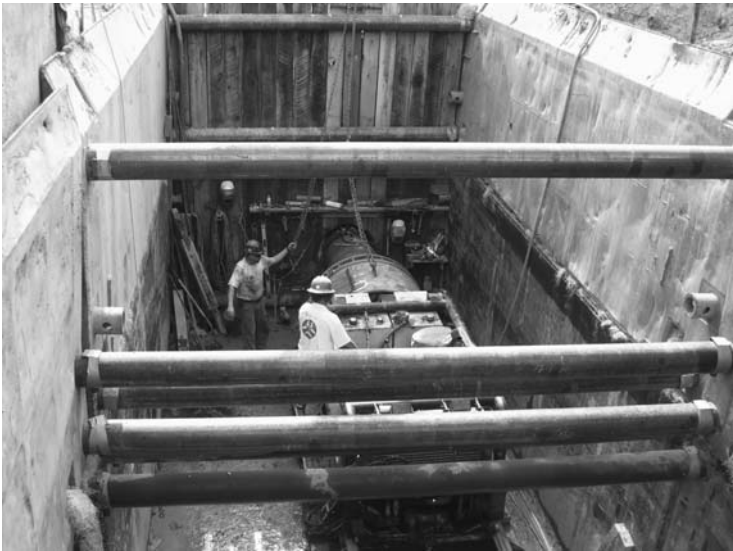
FIGURE 8.17 Horizontal auger-boring method. ( Source: Midwest Mole. )
