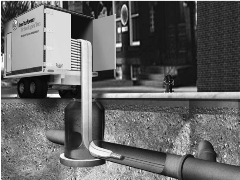
FIGURE 2.5 CIPP installation process. (Source: Insituform Technologies.)
