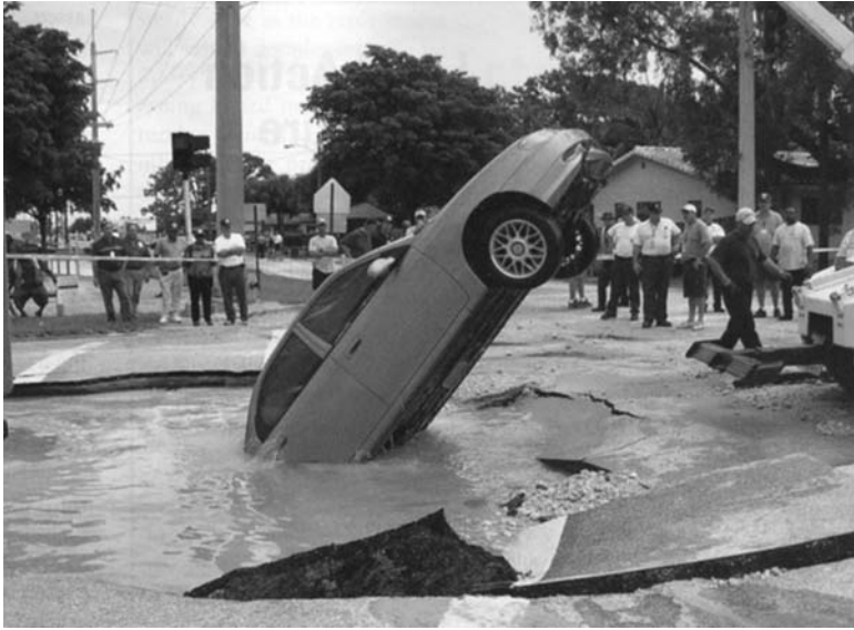
FIGURE 2.2 High emergency cost expected for the pipe failures in urban areas (Source: City of Fort Lauderdale Public Works Department.)
