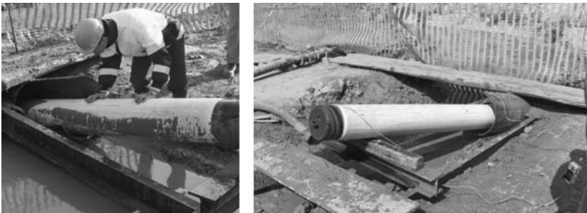
FIGURE 5.11 Coating inspection.
