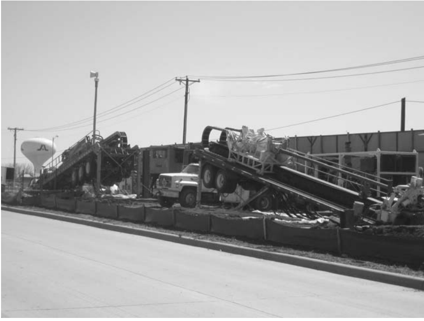
FIGURE 9.1 Staging HDD equipment to minimize environmental impacts.
