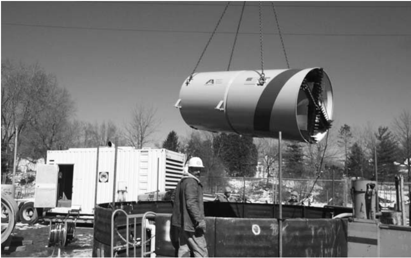
FIGURE 8.1 Conventional pipe jacking. (Source: Akkerman, Inc.)
