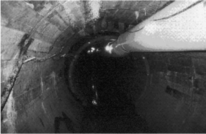
FIGURE 1.11 Inside view of a utility tunneling operations.
