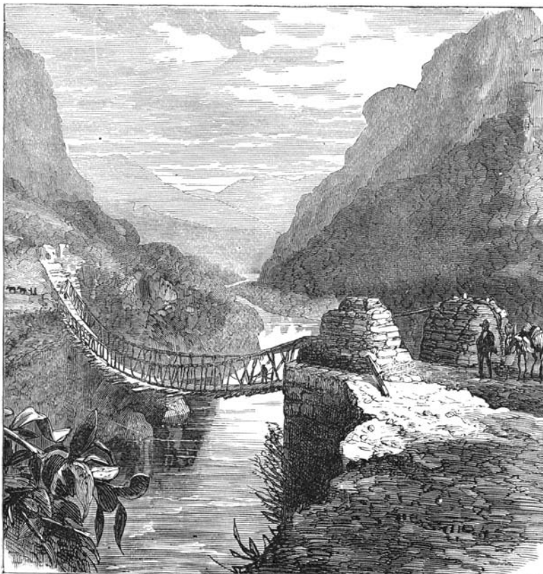
HANGING BRIDGE OVER THE RIO PAMPAS.
