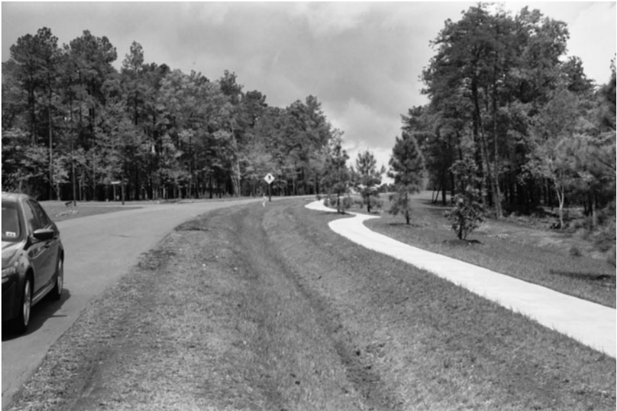
Figure 3-3. Regulatory Issues. Roadway sections imposed at the local level will establish the basis in which the subdivision is designed. Road sections without curb and narrow pavement widths provide best management practices solutions. Source: David E. Johnson, P.E., P.P.
