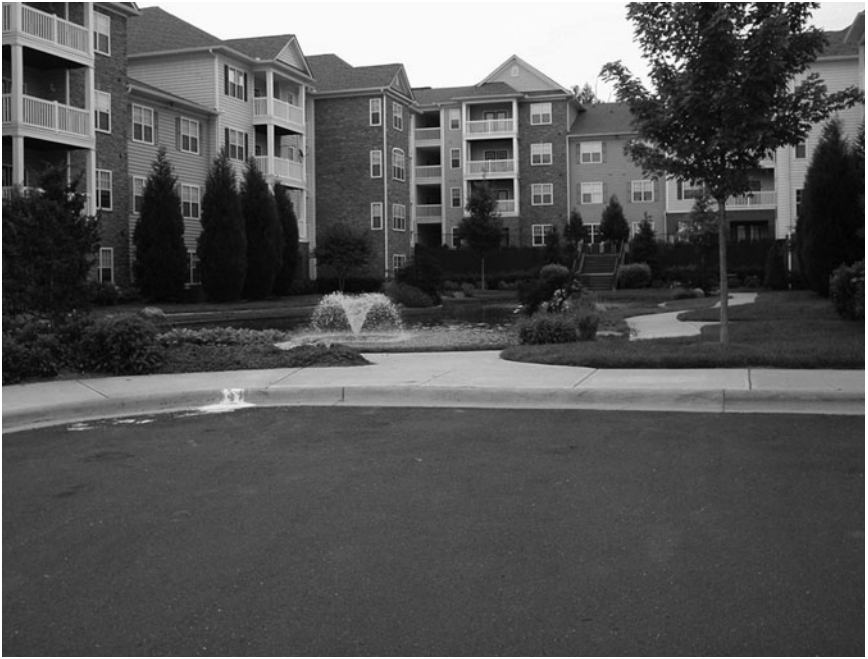
Figure 2-6. High-Density, Multistory Residential Use. A housing product achieving more than 16 units per acre will be a multistory building. Project planning of a high-density, multistory project provides opportunities to separate pedestrian traffic from vehicular movement.
