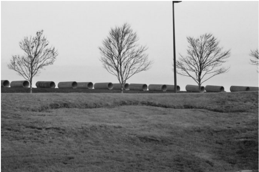
Figure 17-1. Residential Infrastructure. Subdivision improvements are taken for granted until a component fails. Minimizing infrastructure problems starts with quality design, construction, and inspection.
