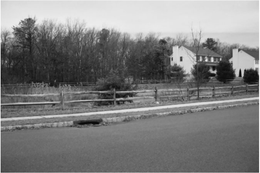
Figure 12-2. Detention Basin. Stormwater management facilities that are dry most of the time are called detention basins. Municipalities require fencing and landscaping if basins are visible from the interior subdivision streets.
