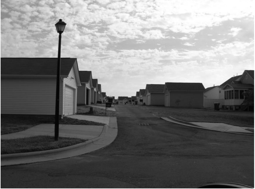
Figure 2-8. Traditional Neighborhood Developments. Most traditional neighborhood development projects include neotraditional site design that locates garage access via backyard alleyways. These alleys are designed for one-way access and may be 14 to 18 feet in width.
