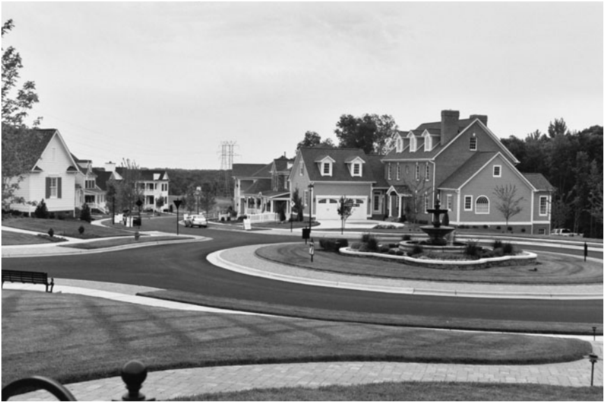
Figure 7-4. Consultants. Creative design and balance between architecture, landscaping features, and infrastructure elements are cost-effective innovations. Source: David E. Johnson, P.E., P.P.
