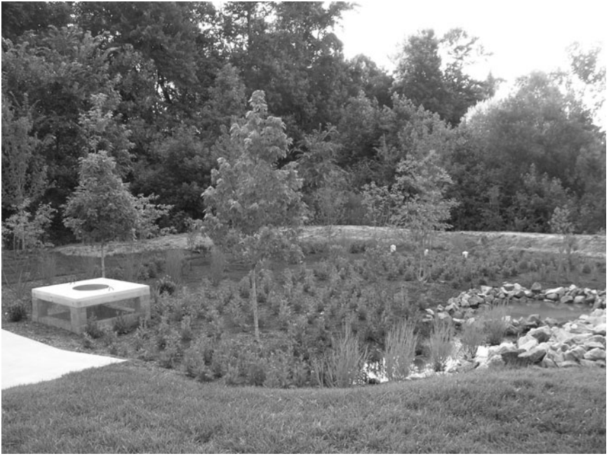
Figure 12-6. Landscaping Material. Stormwater management facilities and best management practices require landscape material designed to enhance runoff filtration. In most cases, landscape architects are involved in selecting the proper plant material. Source: David E. Johnson, P.E., P.P.
