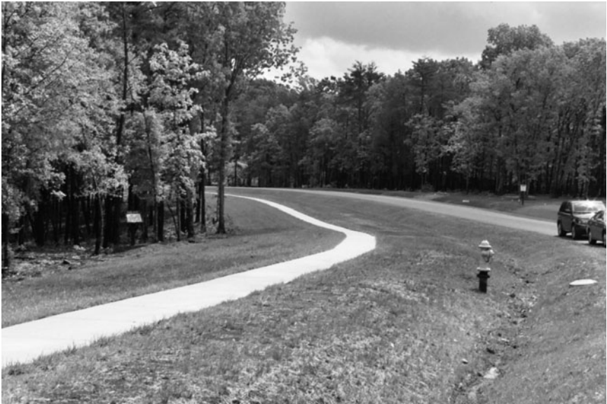
Figure 2-2. Low-Density Residential Use. Many projects located beyond public services will use onsite water and wastewater treatment systems requiring larger lot sizes. The ability to save trees, reduce pavement widths and eliminate curb are consistent design approaches for rural single-family subdivisions.
