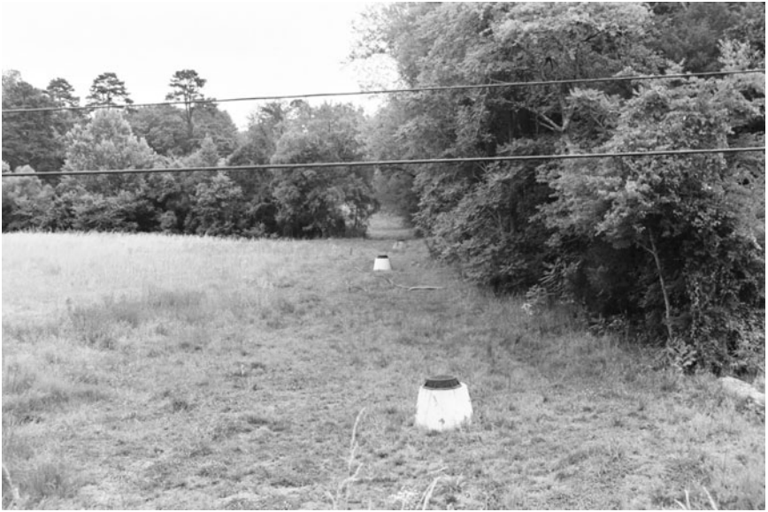
Figure 13-3. Water and Sewer. The availability and capacity of existing water and sewer facilities continue to guide residential growth patterns. In-fill or overlooked properties are developed cost effectively due to the availability of existing infrastructure.
