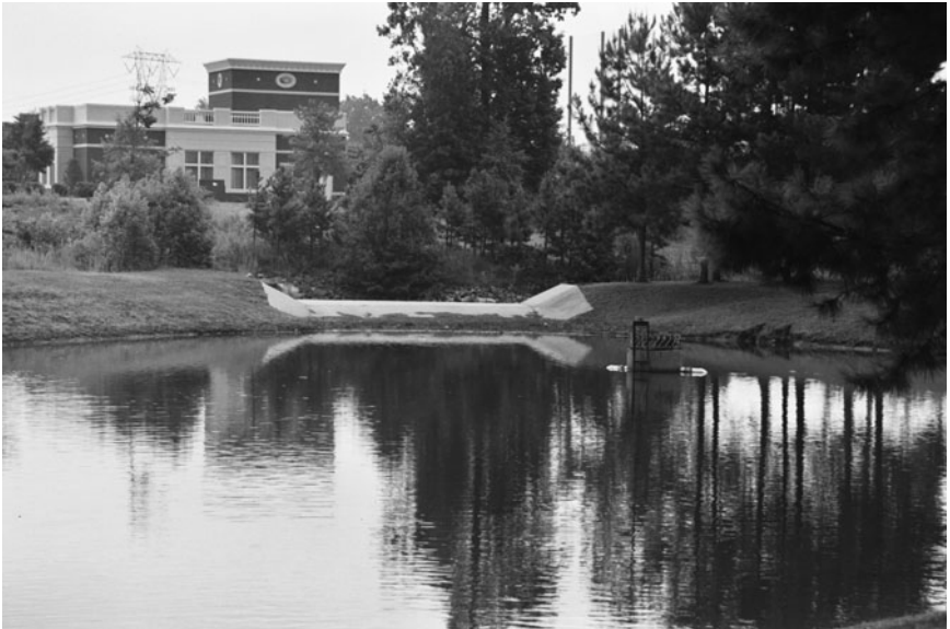
Figure 12-5. Permanent Water Surface. A pond or lake with a permanent water surface is designed with a control structure and concrete emergency overflow weir. The post development runoff is stored within the water body above the permanent water surface elevation and discharged at a controlled rate.
