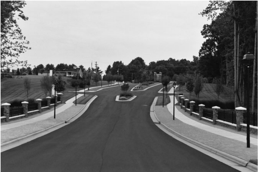
Figure 13-1. Permits. Residential housing projects are subjected to multiple government reviews and permit approvals, including the approval of water and sewer extensions serving new subdivisions. Local, county, regional, state and federal government agencies are involved in the approval and permitting of residential projects. Source: Sidney T. Burns, P.E. Due Diligence Associates, Parkland, Florida
