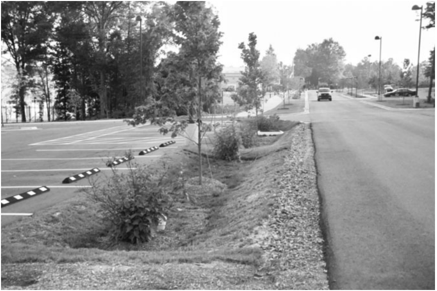
Figure 12-3. Rain Garden. A bio-retention facility or rain garden will be designed in many forms and function as a water quality device. Rain gardens consist of filter media and landscape material, and are best designed for small drainage areas. Source: David E. Johnson, P.E., P.P.
