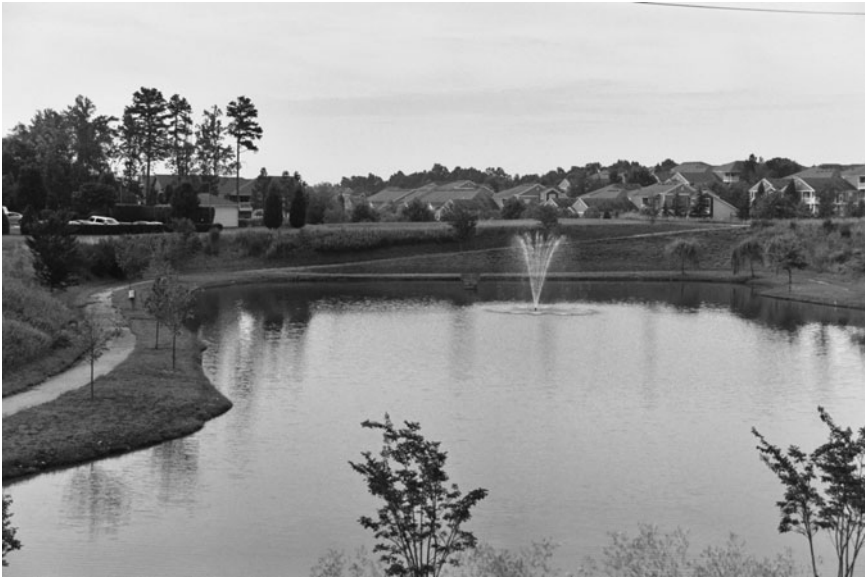
Figure 12-1. Retention Basin. Stormwater management facilities with a permanent water surface are called retention basins. If designed properly, the basin is a designed amenity for the project, including a walking path around the basin. Source: David E. Johnson, P.E., P.P.
