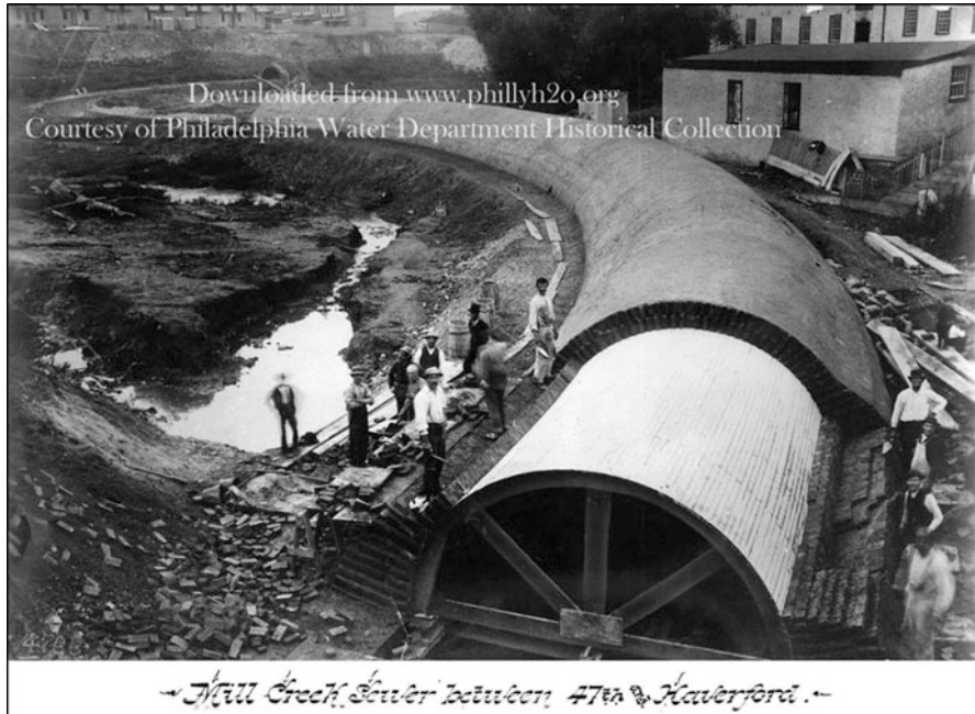
Fig. 1 Mill Creek Sewer under construction, West Philadelphia, USA ca. 1883 (Image courtesy of Adam Levine, from the Philadelphia Water Department Historical Collection)
