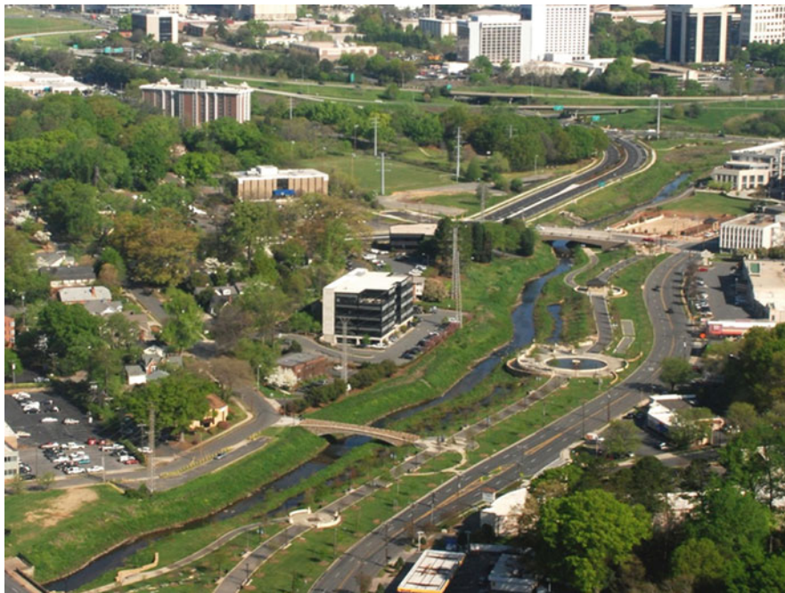
Fig. 13 Little Sugar Creek after construction, Meredith Moore, Mecklenburg County Storm Water Services (Image courtesy of Crystal Taylor, P.E., Charlotte–Mecklenburg Storm Water Services, 2012)
