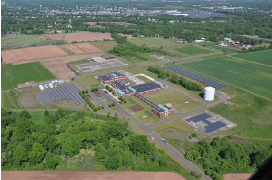
Fig. 6 Photovoltaic system at NJAW Canal Road WTP ( Source: New Jersey American Water ) (with permission from NJAW – August 31, 2015)
