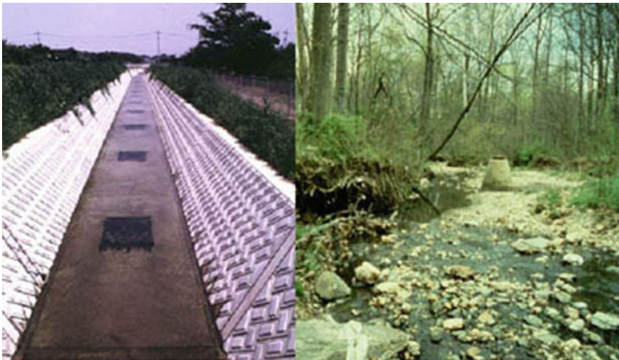
Fig. 1 An urban channelized and “hardened” stream ( left ). An eroded stream (with sewer manhole exposed) ( right ) ( Source: US EPA )
