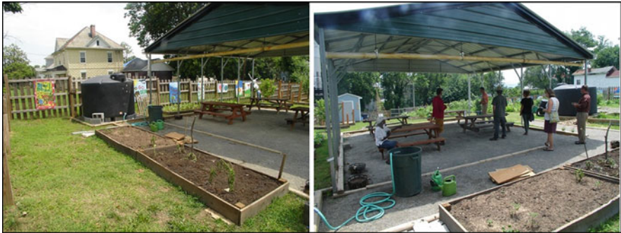
Fig. 9 Rainwater harvesting systems at Hurt Park Community Garden, photo on the left shows a 1500 gal (5.7 m 3 ) barrel to the left of the pavilion; photo on the right shows a second barrel to the right of the pavilion (Photos: Third author 2013)
