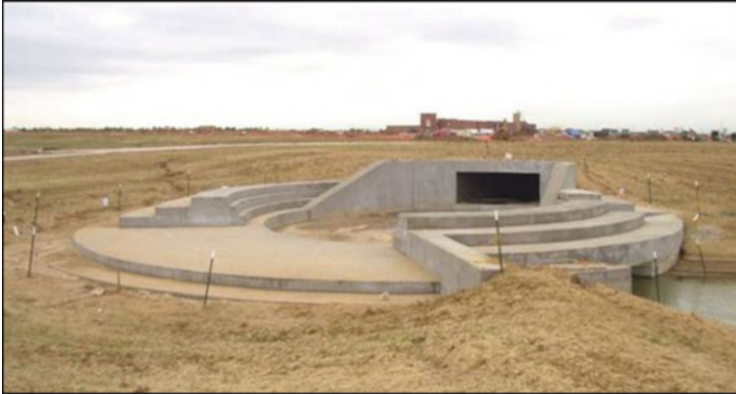
Fig. 17 Architectural outfall structures at constructed wetlands (Image courtesy of Jane Kopperl, Matrix Design Group (EDAW) 2002)
