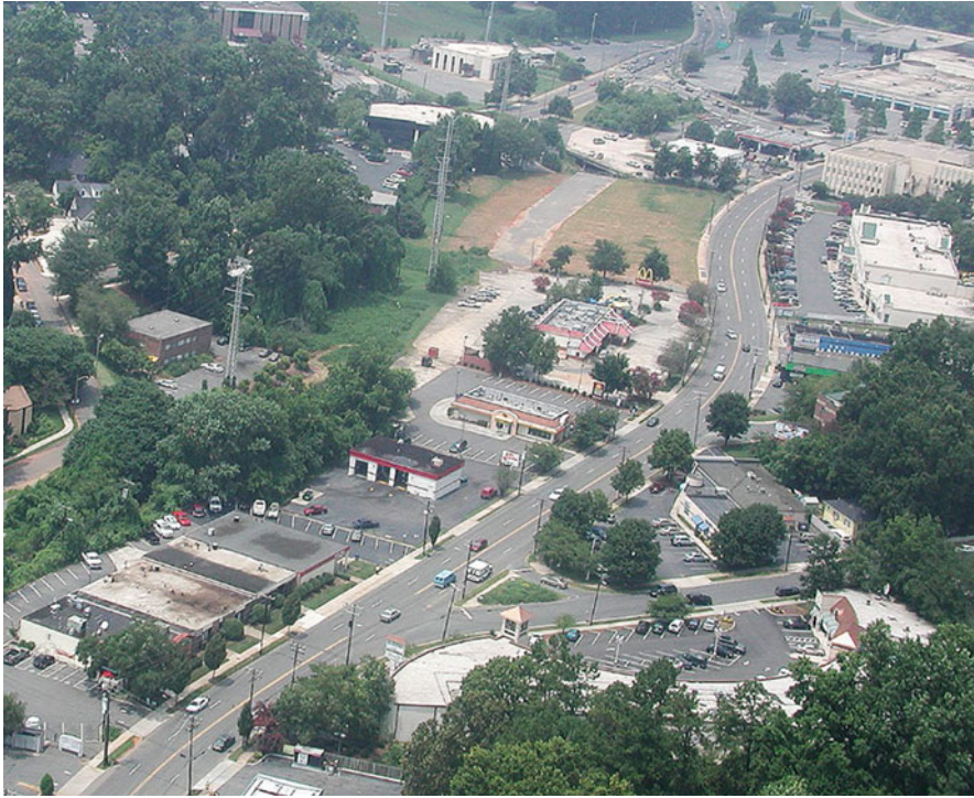
Fig. 10 Little Sugar Creek prior to construction, Meredith Moore, Mecklenburg County Storm Water Services (Image courtesy of Crystal Taylor, P.E., Charlotte–Mecklenburg Storm Water Services, 2002)
