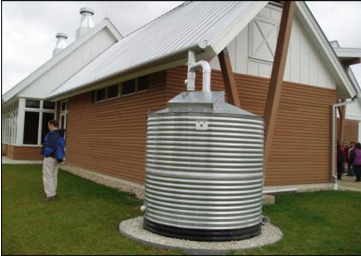
Fig. 18 Rainwater harvesting ( Source: Center for Watershed Protection )
