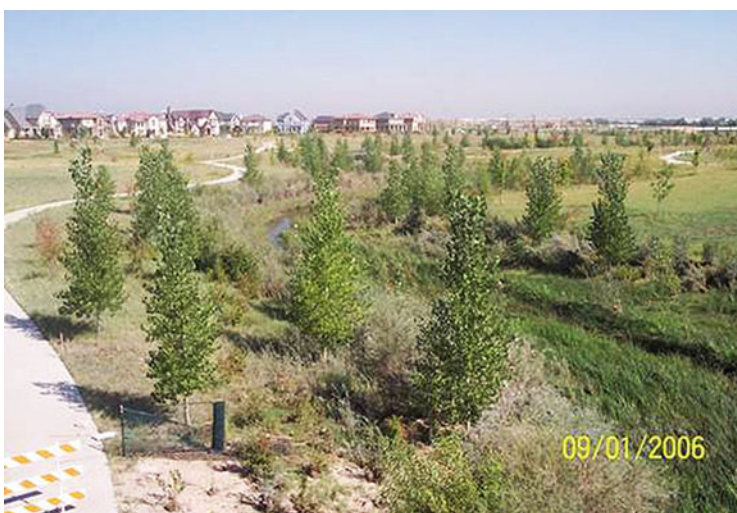
Fig. 20 Westerly Creek at Stapleton after construction (Image courtesy of Jane Kopperl, Matrix Design Group (EDAW), 2006)
