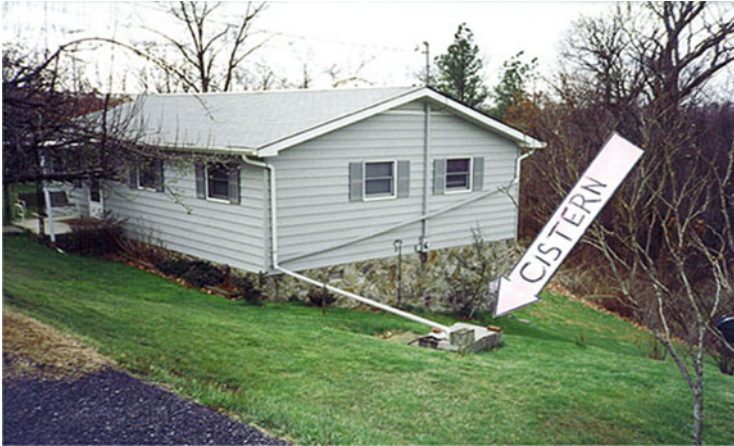
Fig. 2 Traditional rainwater capture and use in a mountaintop house, Southwest Virginia, USA (Source: first author)
