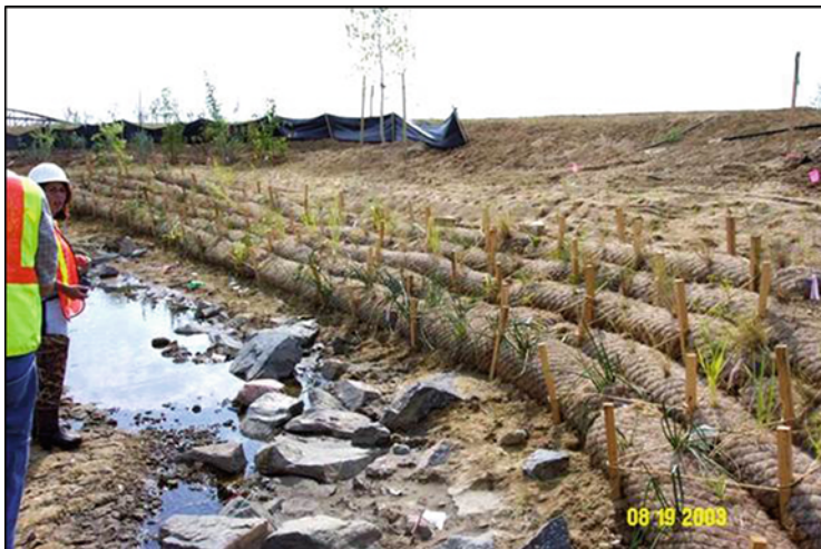
Fig. 19 Vegetated biologs at installation (Image courtesy of Jane Kopperl, Matrix Design Group (EDAW), 2003)
