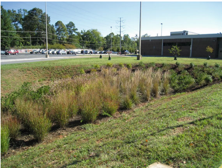
Fig. 13 Bioretention ( Source: first author )
