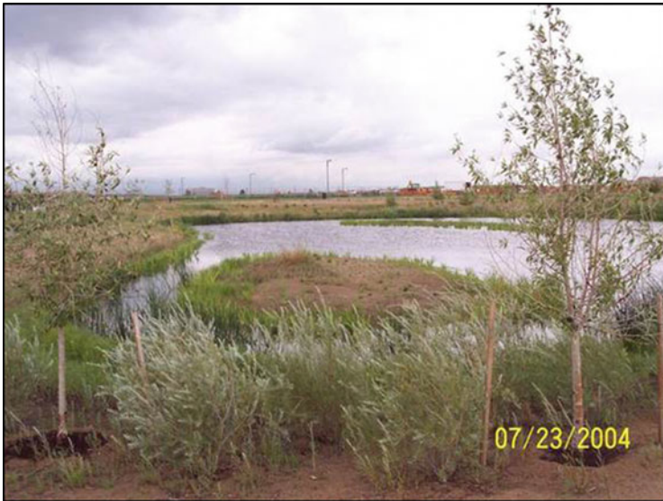
Fig. 18 Outfall structures and constructed wetlands after construction (Image courtesy of Jane Kopperl, Matrix Design Group (EDAW) 2004)
