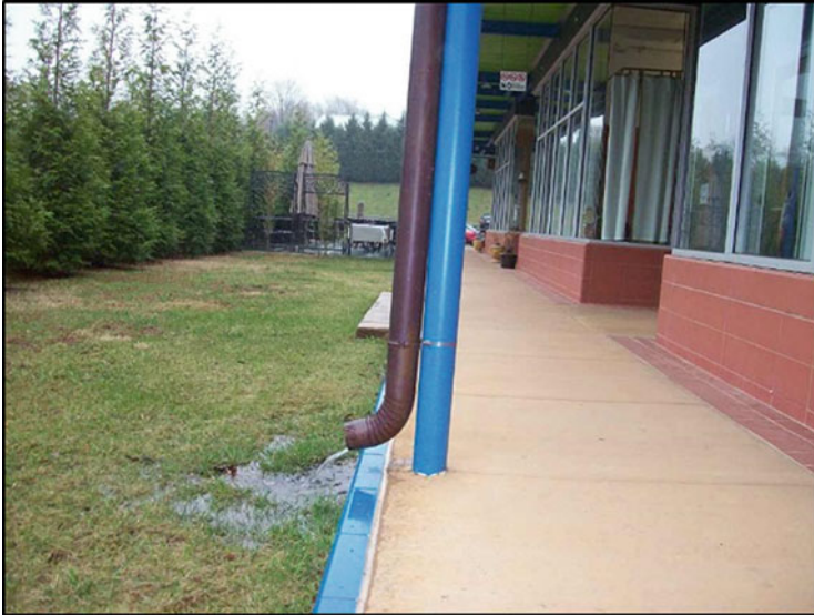
Fig. 11 Simple impervious surface disconnection ( Source: first author )
